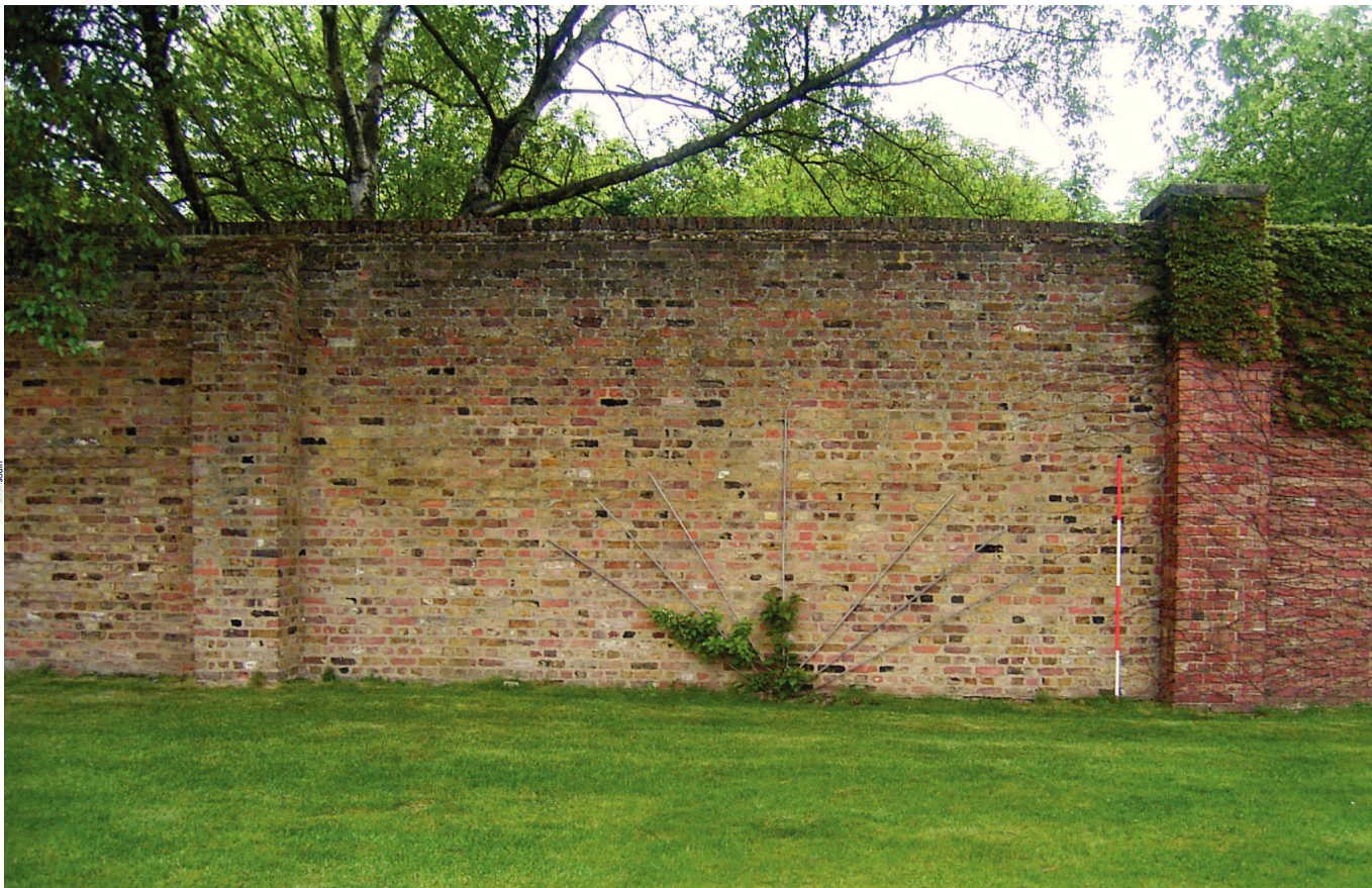
Plate 19: West elevation of west boundary wall with former tennis court showing modern refacing and darker brickwork belonging to the 18th century
