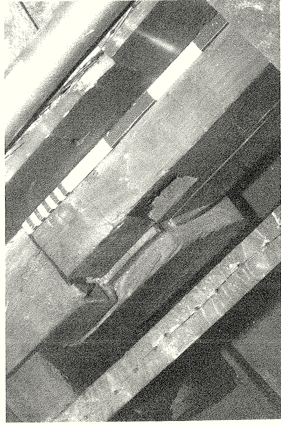
Figure 14: Detail showing large primary ridge-piece supporting smaller secondary ridge-piece (added when the louvre was removed)
