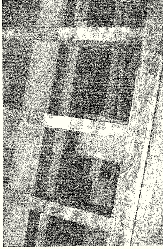
Figure 15: Detail of purlin adjoining west face of Truss 4
