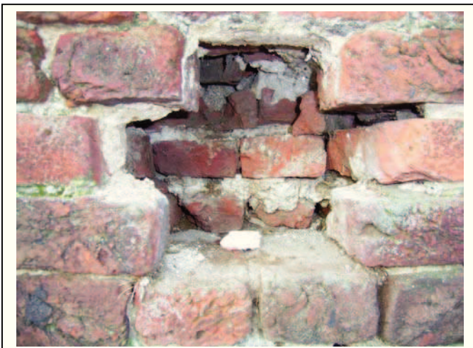
Plate 3 External intervention showing core of south wall.
