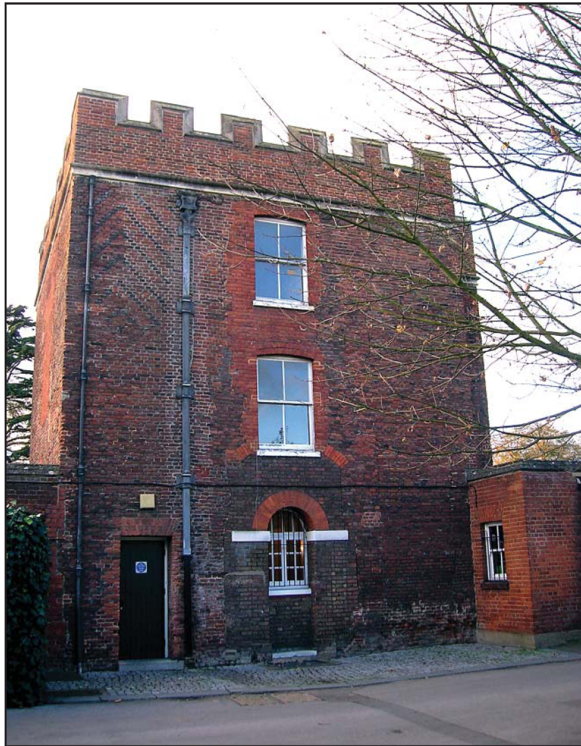
Plate 1: East elevation, external view (pre-works)
