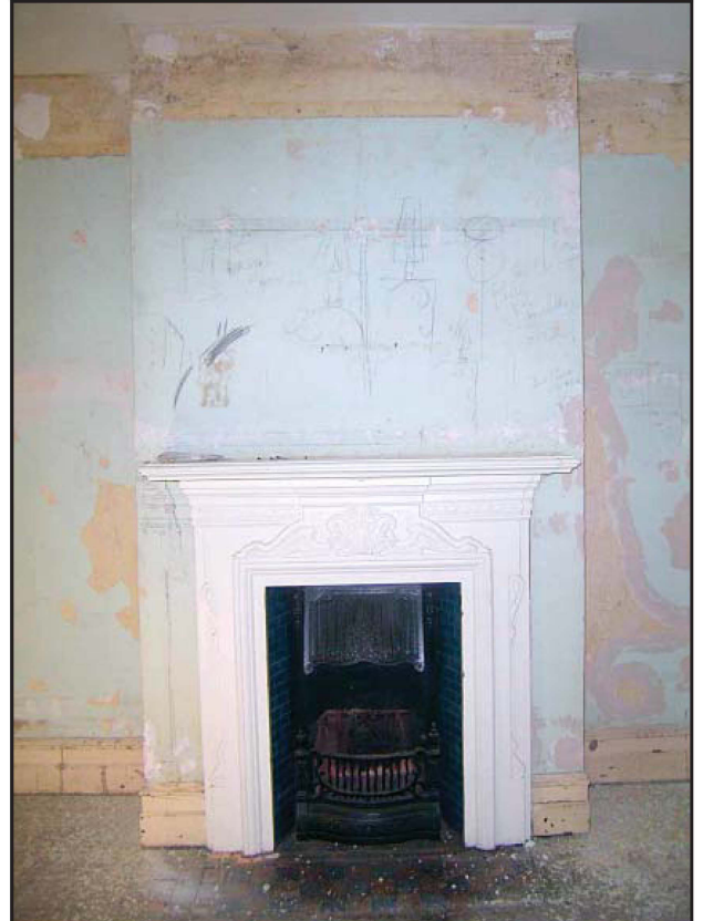
Plate 60: Fireplace, first floor, internal view, room TYFF01
