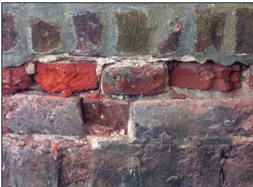
Plate 47: South parapet, internal face, illustrating Tudor brickwork
