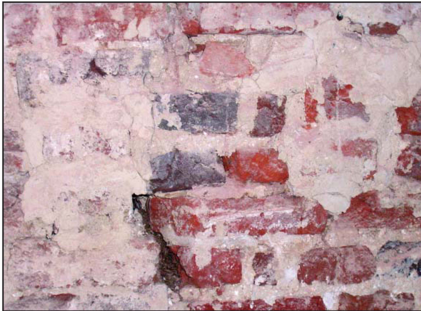
Plate 9: East elevation, internal view, first floor, showing chamfered Tudor brick
