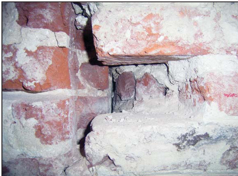
Plate 8: East elevation, internal view, second floor, showing Tudor plaster reveal
