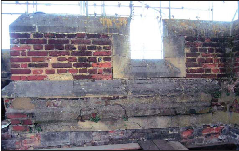
Plate 43: North parapet, east section, internal face, showing consolidation and surviving brick corbel
