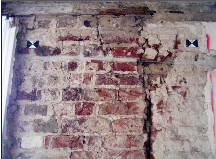
Plate 10: East elevation, internal view, second floor, illustrating truncated Tudor break below ceiling
