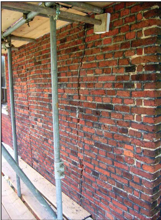
Plate 4: East elevation, external view, illustrating Tudor brickwork and phasing break to north of the window (the jagged break is structural)
