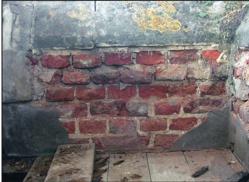
Plate 45: North parapet, central section, internal face, showing Tudor brickwork
