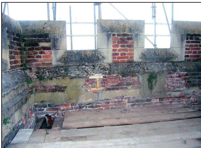
Plate 41: East parapet, internal face, north end illustrating earlier consolidation
