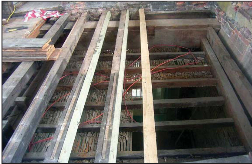
Plate 56: Parapet floor, north view
