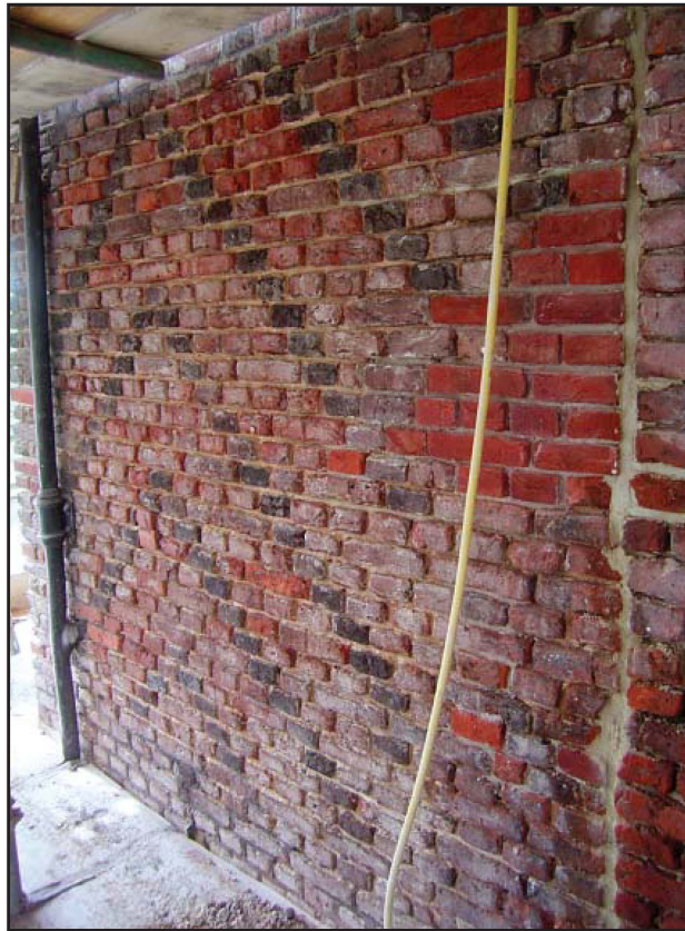
Plate 15: East elevation, external view, second floor, illustrating Tudor diaperwork
