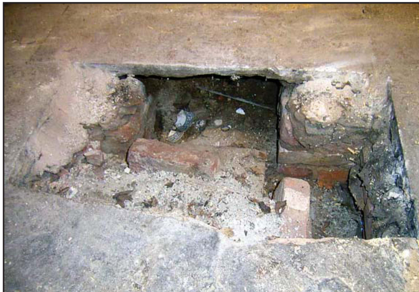
Plate 63: Culvert, internal view, exposed in basement
