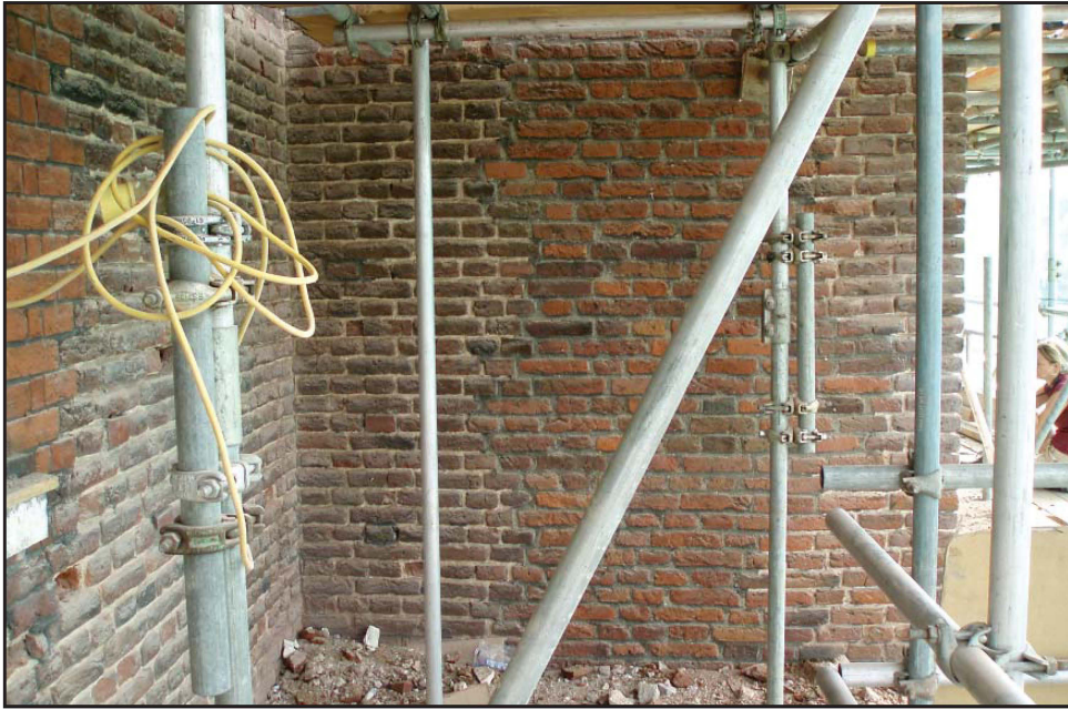
Plate 12: North elevation, external view, second floor, showing central panel of 18th century patching
