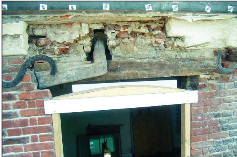
Plate 53: West elevation, external view, second floor, timber lintels exposed above window
