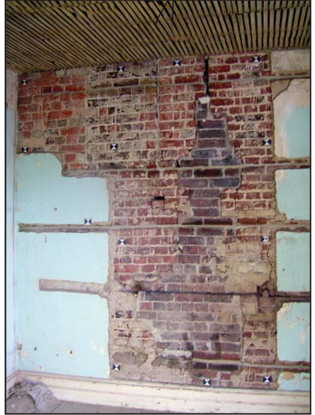
Plate 7: South elevation, internal view, first floor, illustrating Tudor break below ceiling and 20th century patching
