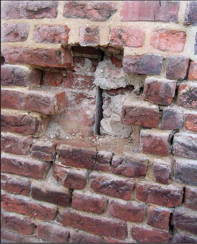
Plate 6: South elevation, external view, showing Tudor plaster reveal
