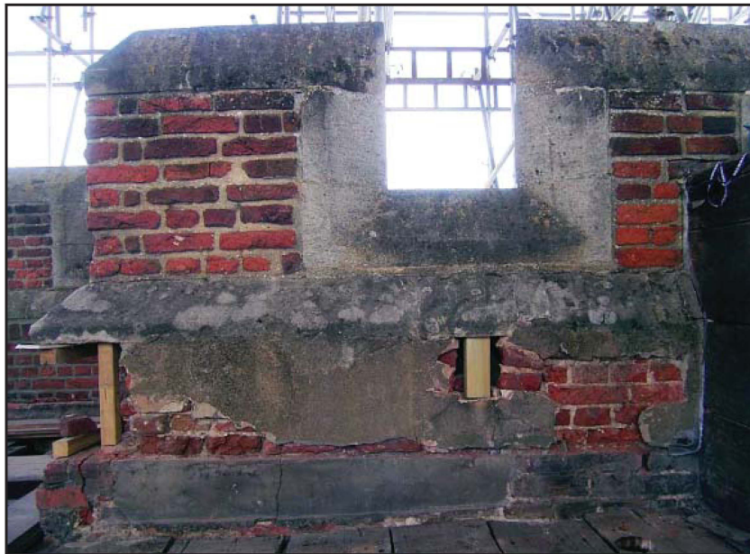
Plate 49: West parapet, internal face, showing consolidation and Tudor brickwork
