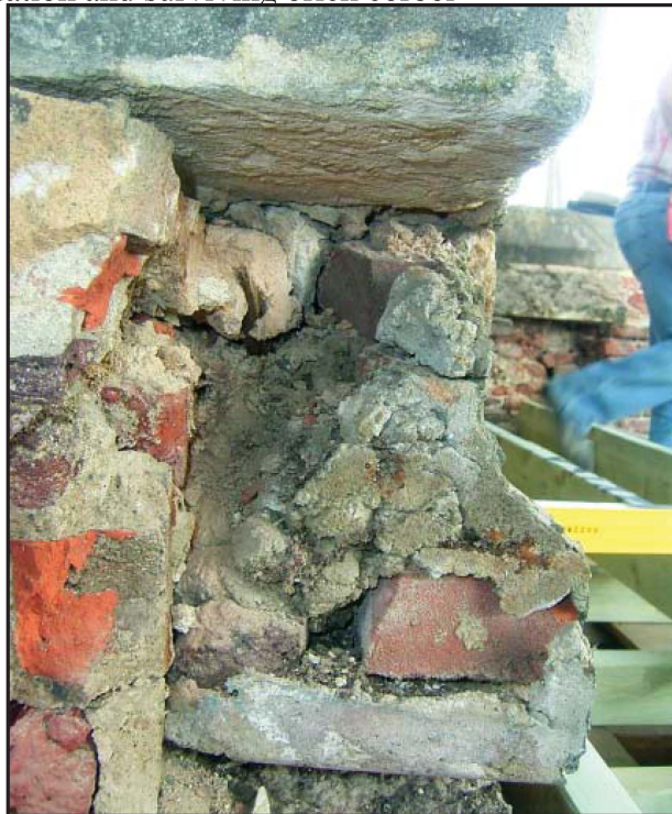
Plate 44: North parapet, east section, internal face, illustrating inner core
