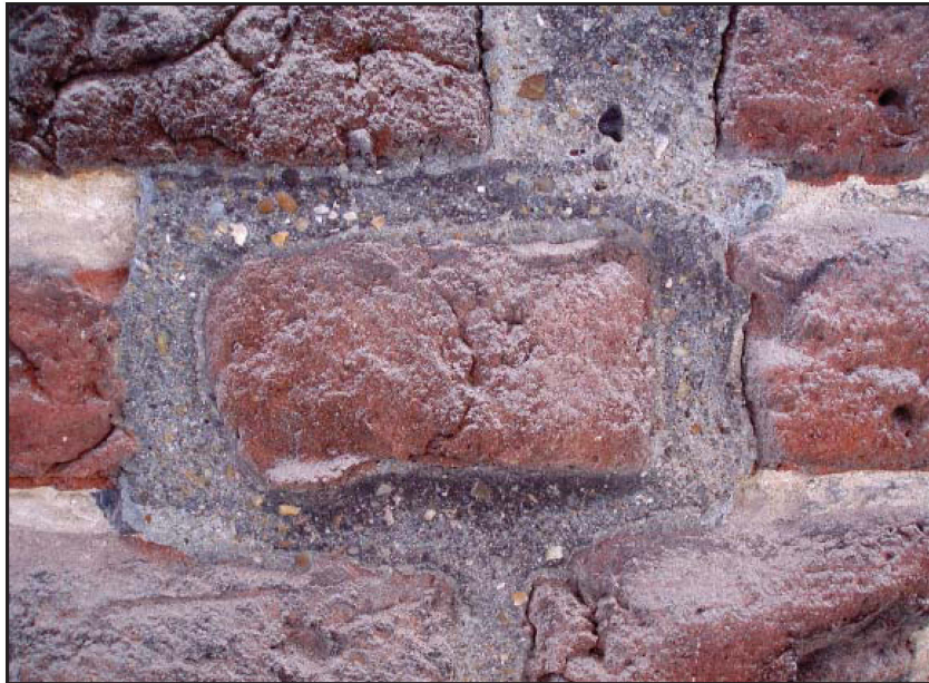
Plate 39: North elevation, first floor, external view, showing brick repair
