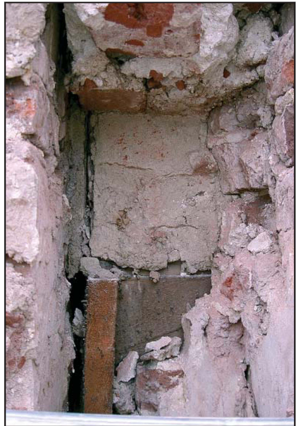
Plate 14: West elevation, external view, illustrating timber elements within vertical shaft
