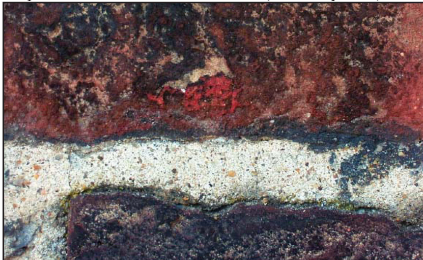
Plate 69: South elevation, external view, red paint evident on brick (centre of picture)
