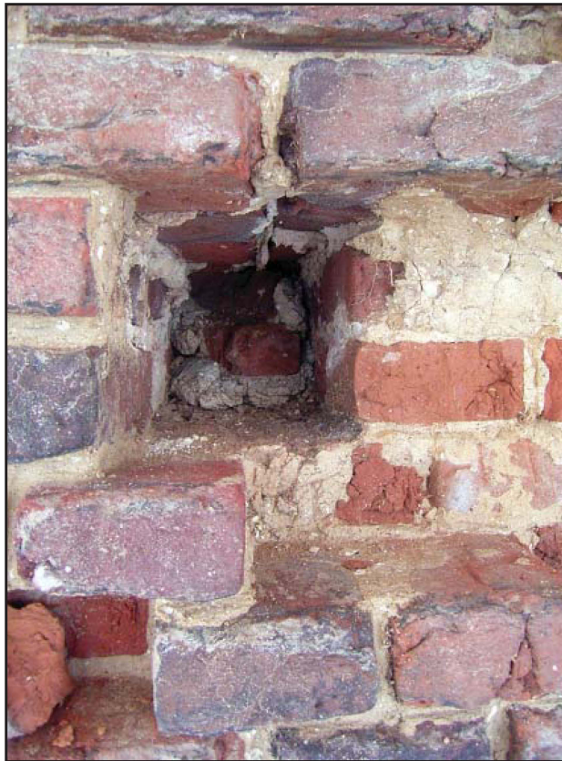
Plate 18: East elevation, external view, second floor, showing possible Tudor putlog
