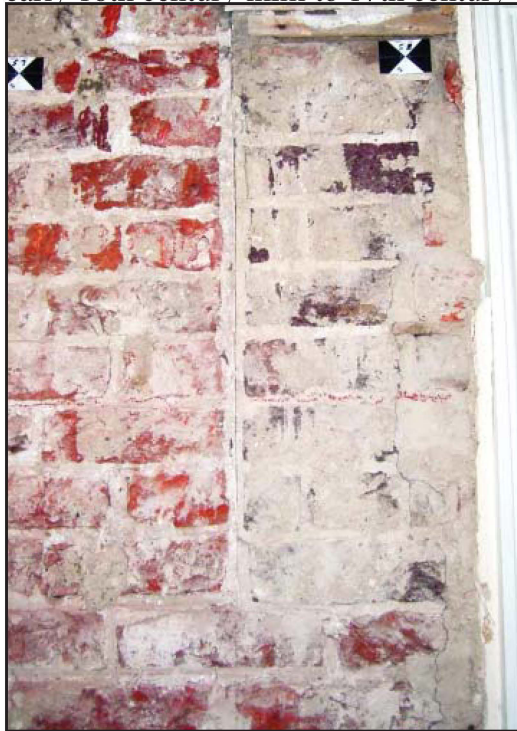
Plate 31: East elevation, first floor, showing 17th plaster reveal and infill
