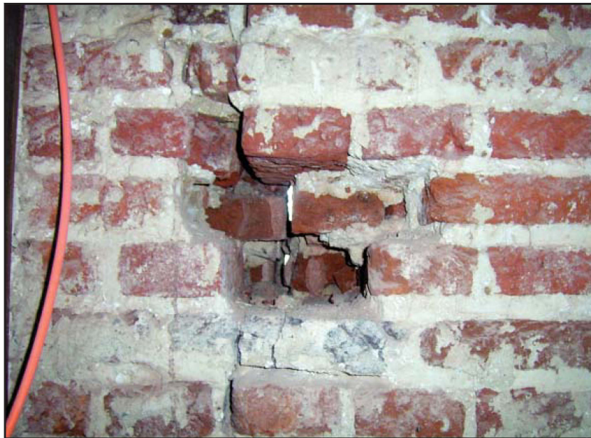
Plate 16: East elevation, internal view, second floor, showing possible Tudor putlog (north)
