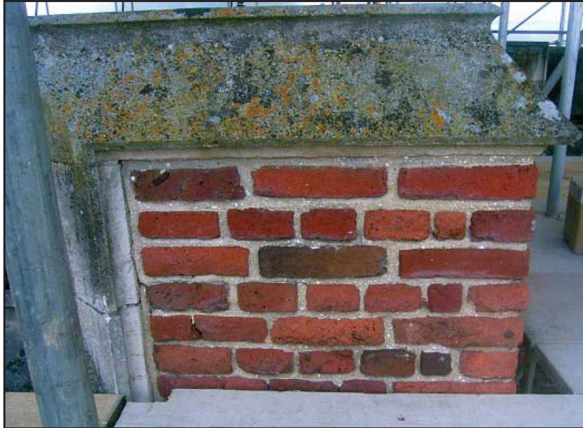
Plate 42: East parapet, external face, north crenelation illustrating Tudor and later bricks in top course
