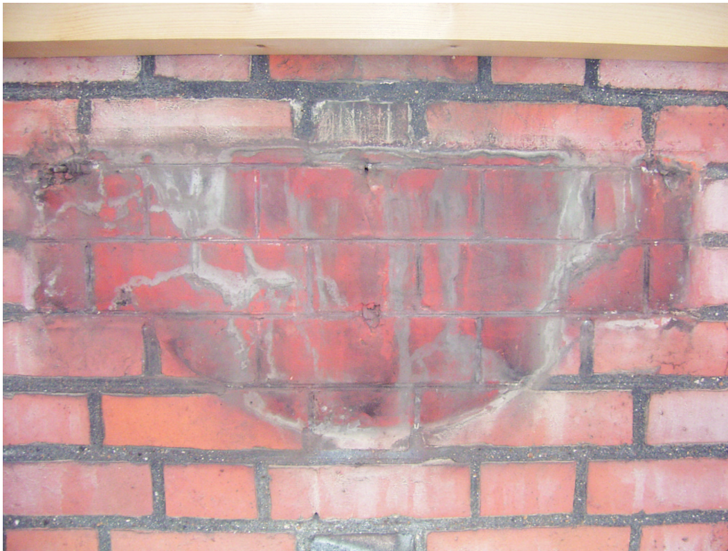
Plate 51: NW turret brickwork following removal of lead plaque
