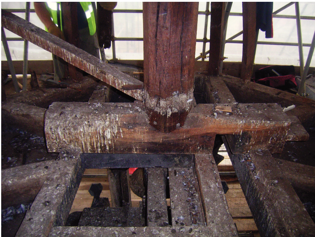
Plate 41: Base of octagonal post within lantern cap frame
