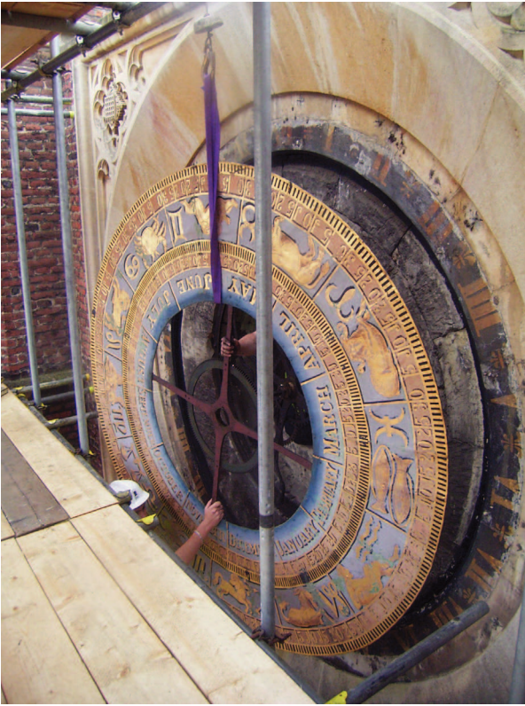
Plate 14: Astronomical clock - removal of dial
