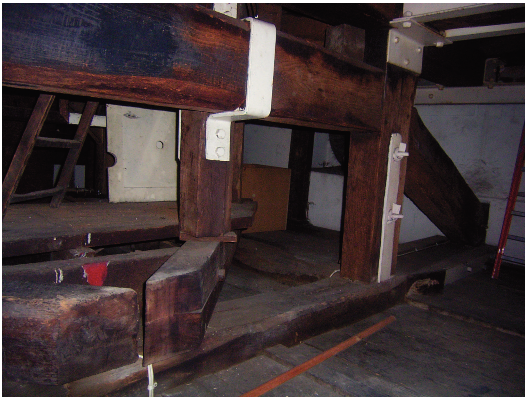
Plate 47: 18th century and later supports within cupola
