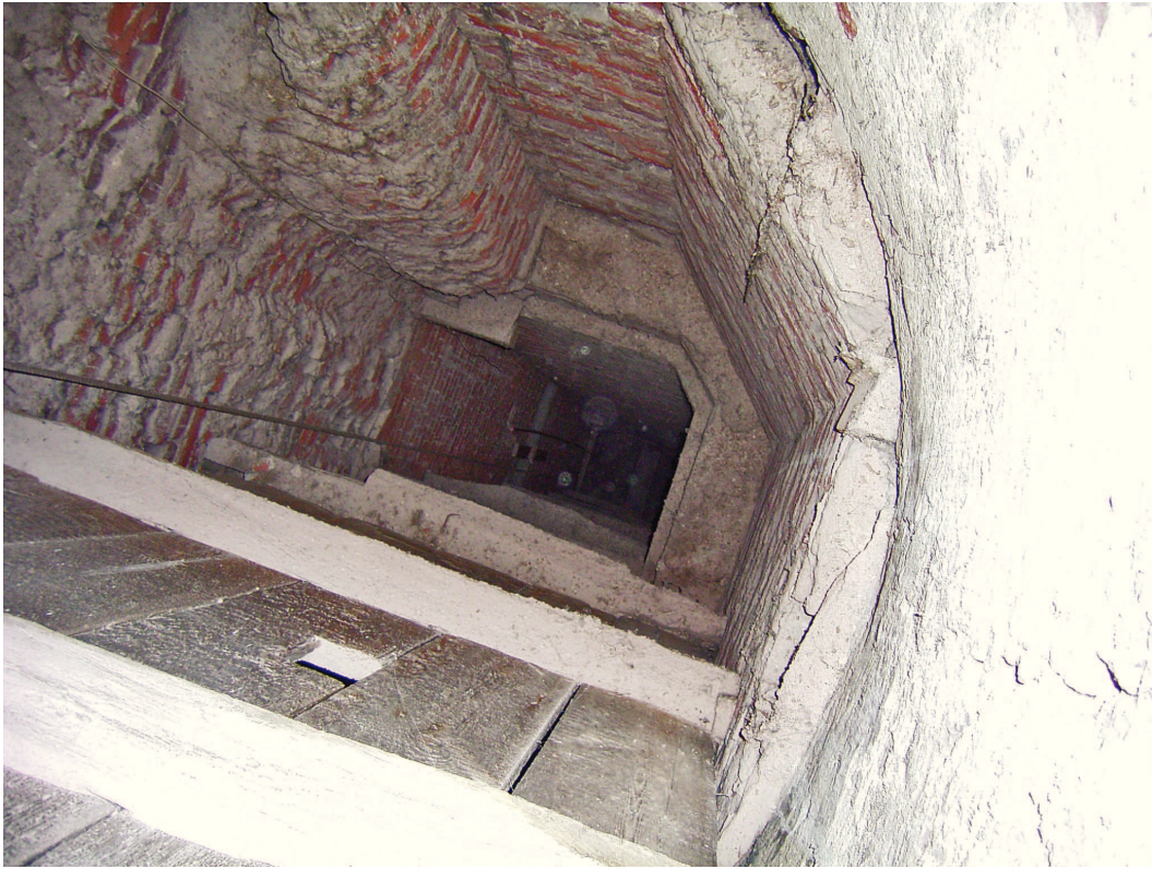
Plate 30: NW turret, view down turret from second floor level
