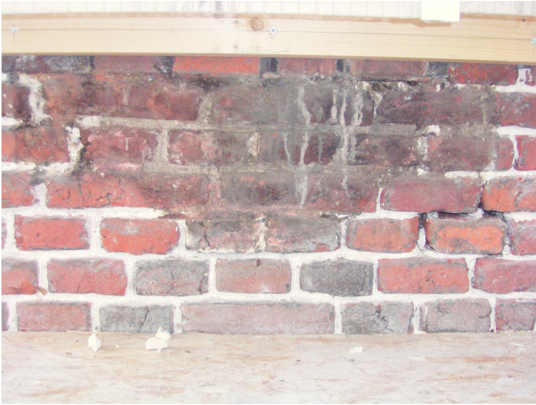
Plate 48: SE turret brickwork following removal of lead plaque
