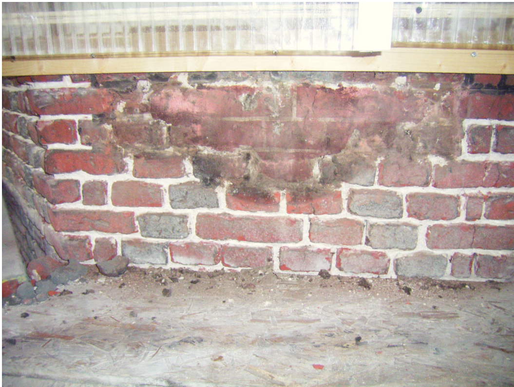
Plate 49: NE turret brickwork after removal of lead plaque
