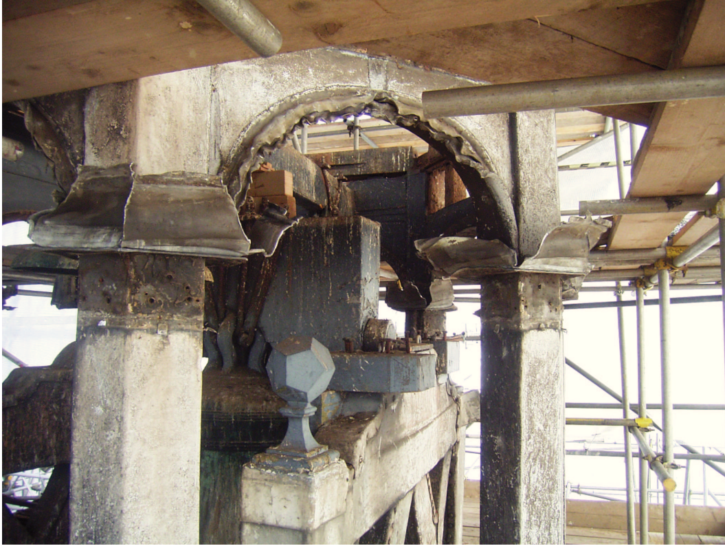
Plate 42: Removal of lead from lantern
