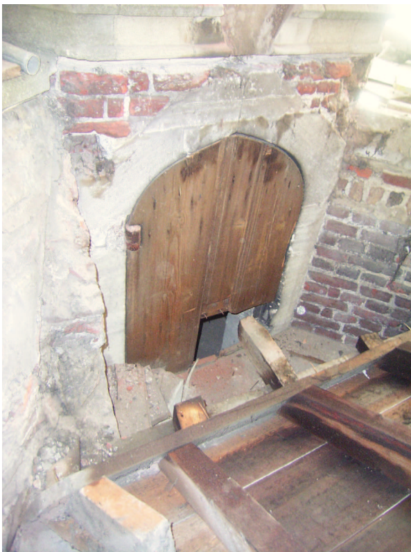
Plate 25: SE turret exterior, view of doorway hidden beneath cupola valley boards
