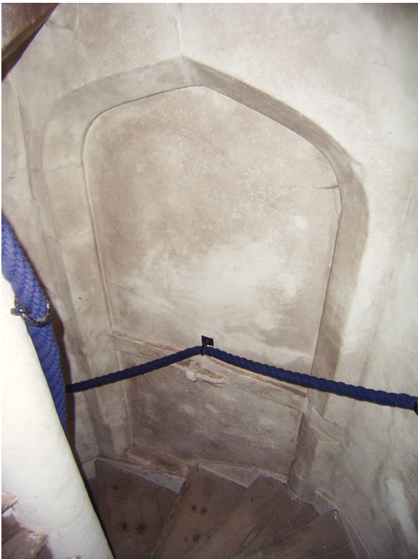
Plate 18: Blocked doorway within NE turret
