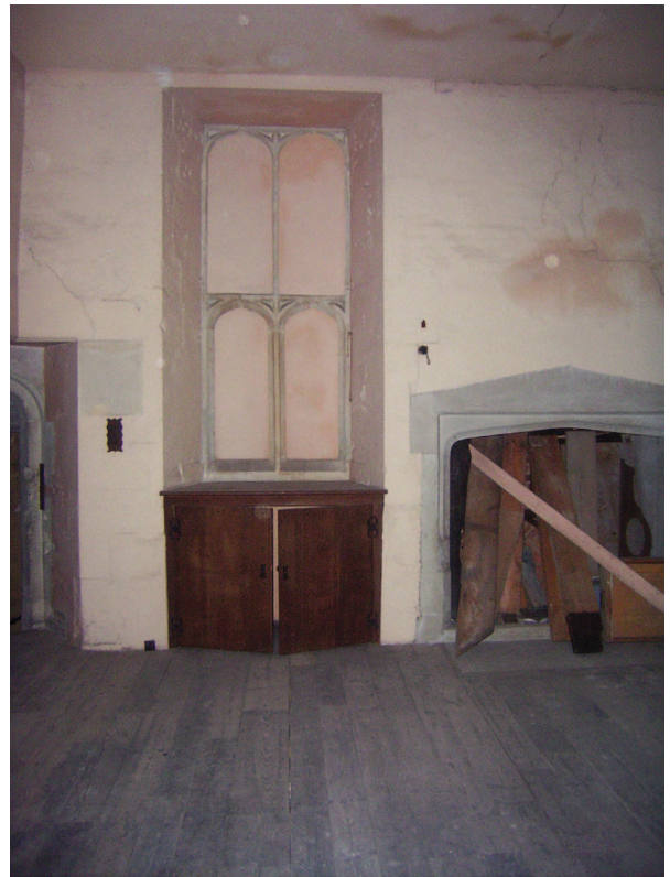
Plate 32: Room beneath clock room, blocked window
