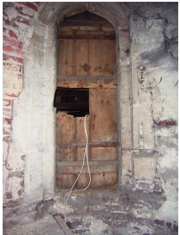
Plate 26: SE turret interior, view of doorway hidden beneath cupola valley boards
