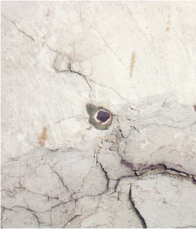
Plate 23: SW turret interior, nail with lead
