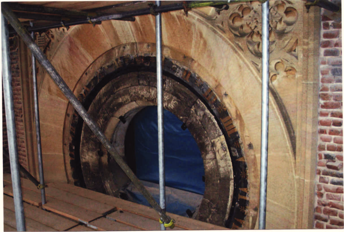
Plate 6. Astronomical Clock. Earlier dial of Caen stone normally hidden behind astronomical dial.
