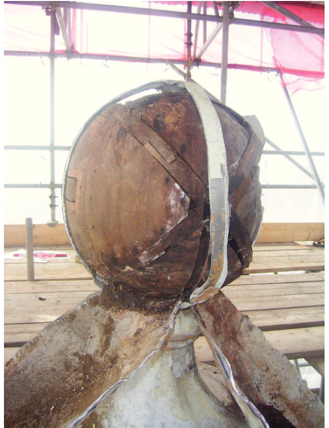
Plate 38: Ball finial during removal of leadwork
