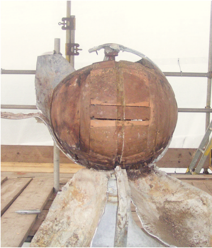
Plate 39: Ball finial during removal of leadwork
