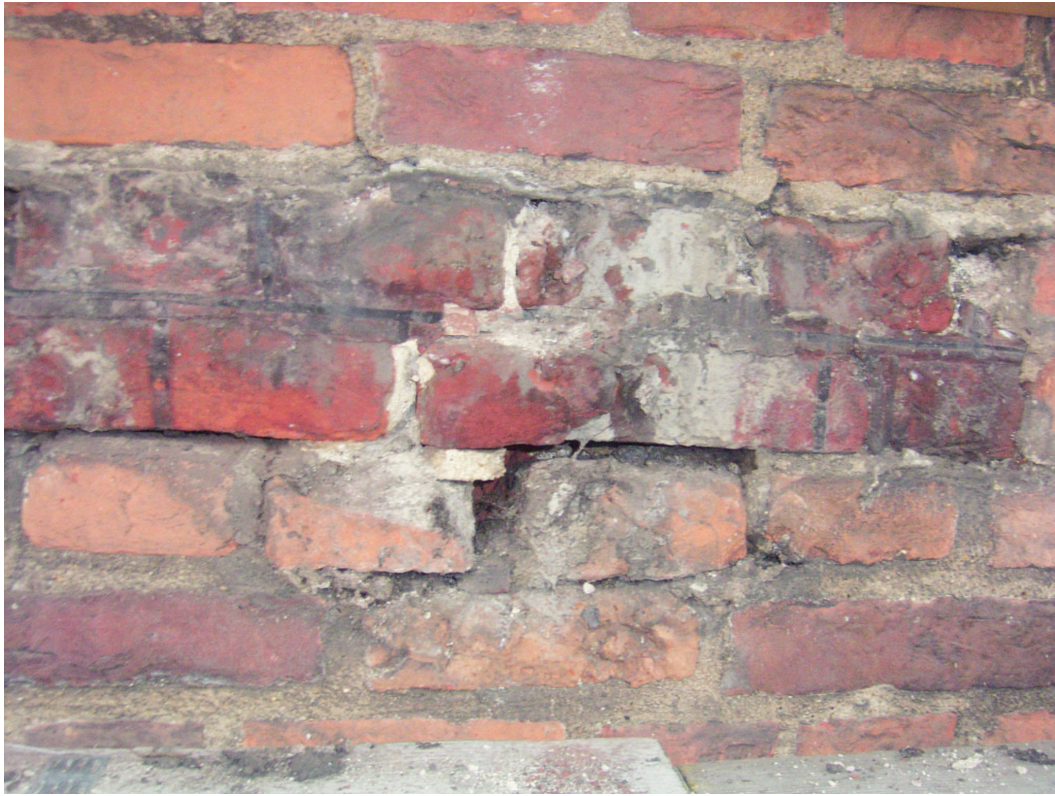
Plate 50: SW turret brickwork following removal of lead plaque
