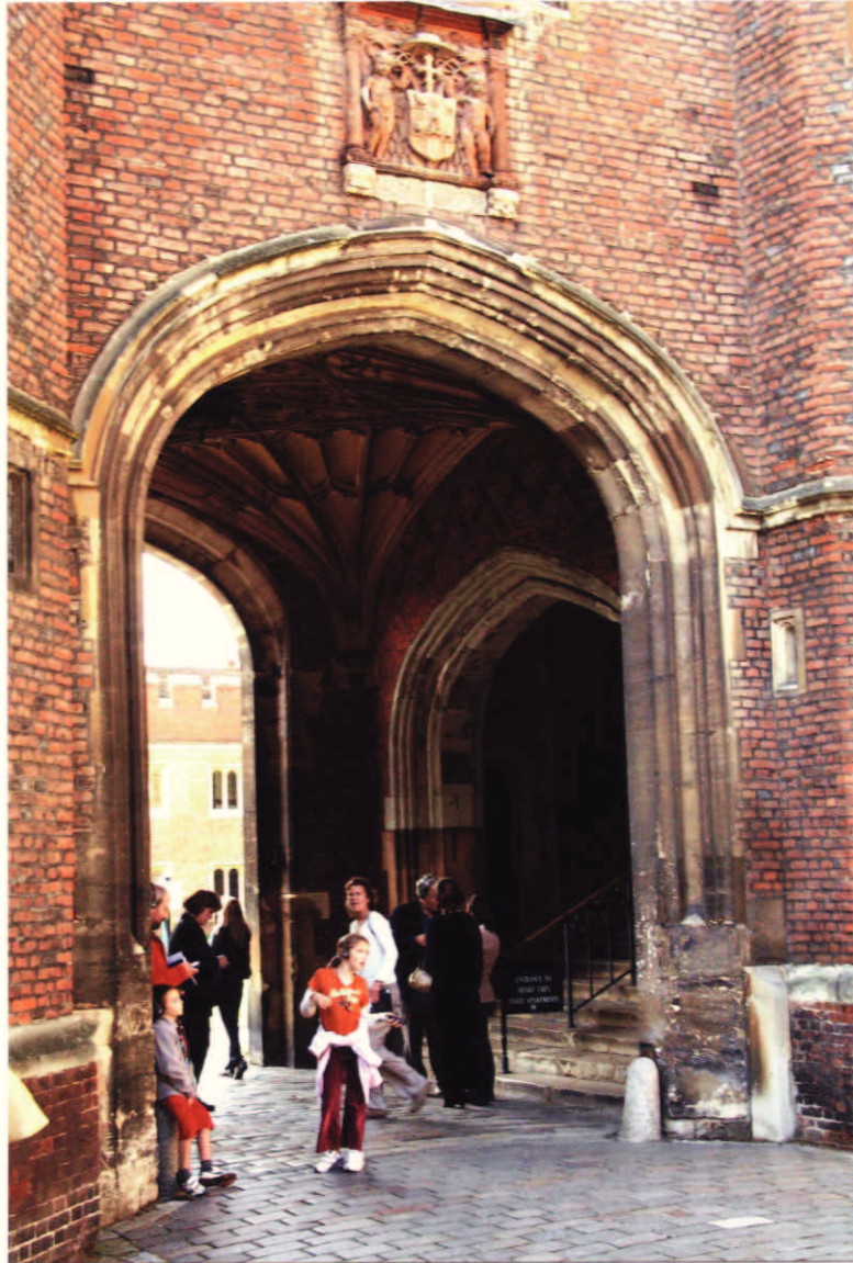
Plate 5. Clock Tower, east entrance showing Caen stone arch and Wheatley Limestone jambs.
