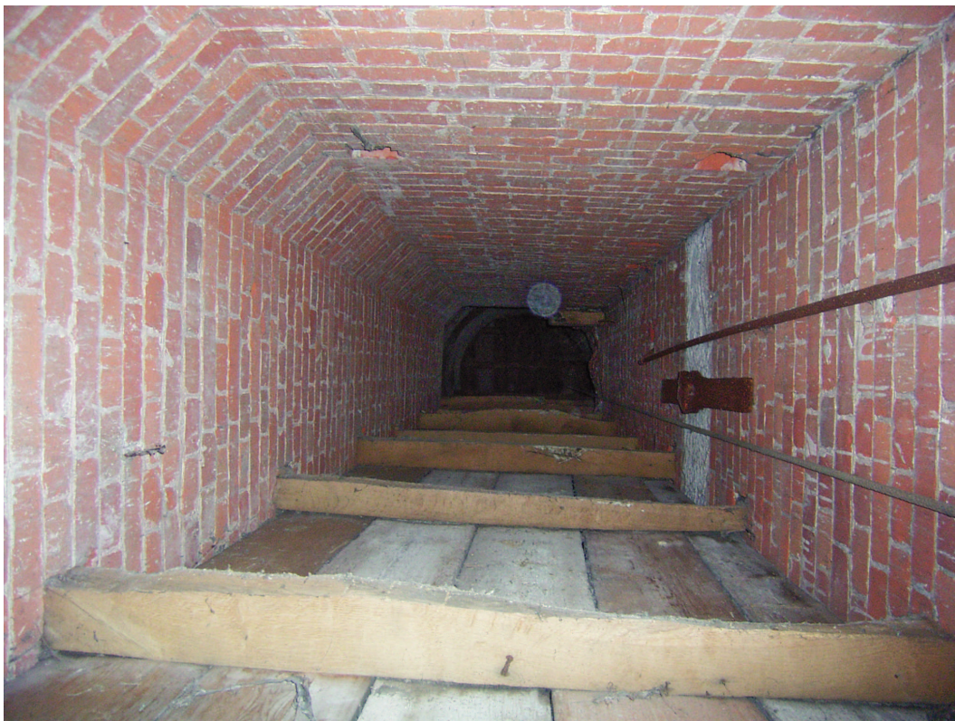
Plate 29: NW turret, view up turret from ground level
