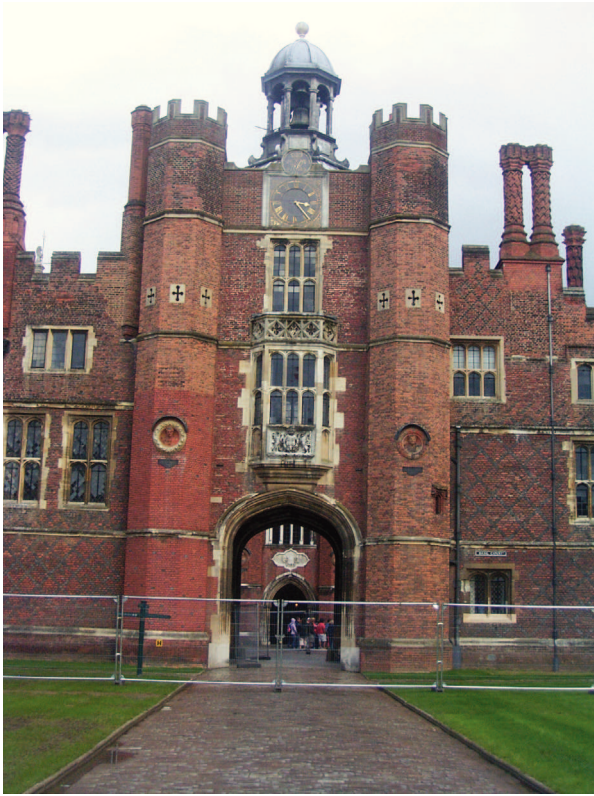
Plate 8: West elevation of gatehouse prior to works
