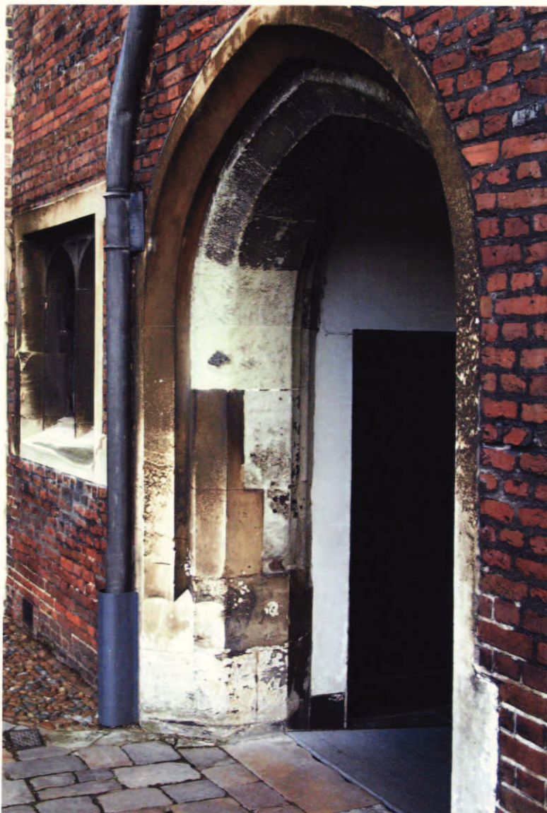
Plate 10. Clock court, 4-flue chimney stack plinth. Yellow Guiting stone? replacement in Bath stone offset course.
