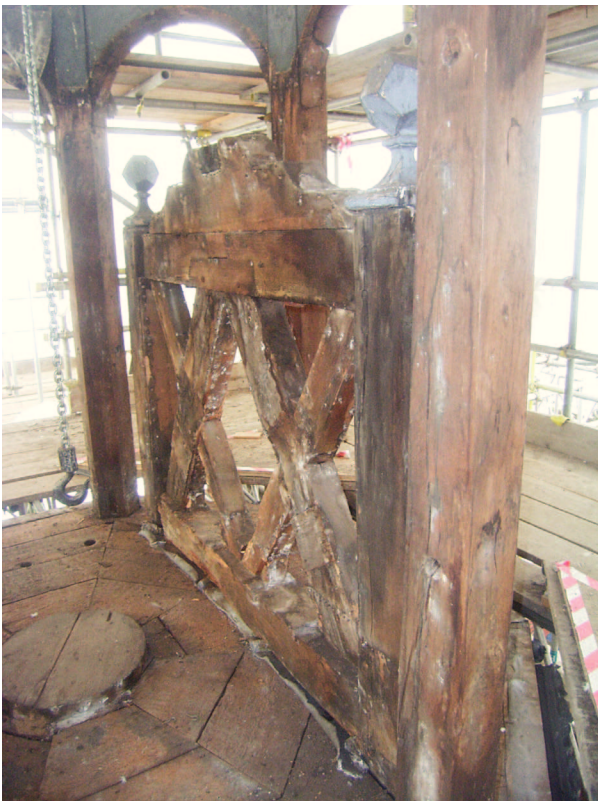
Plate 43: Bell frame following removal of lead
