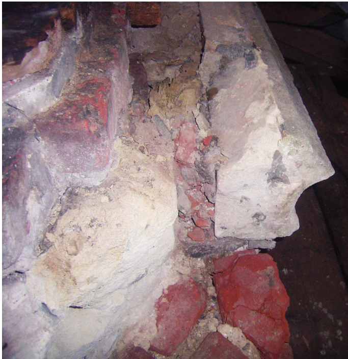
Plate 58: Reused stonework within NE turret upper string course
