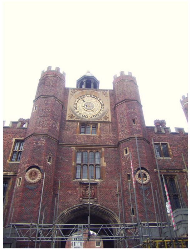
Plate 9: East elevation of gatehouse prior to works
