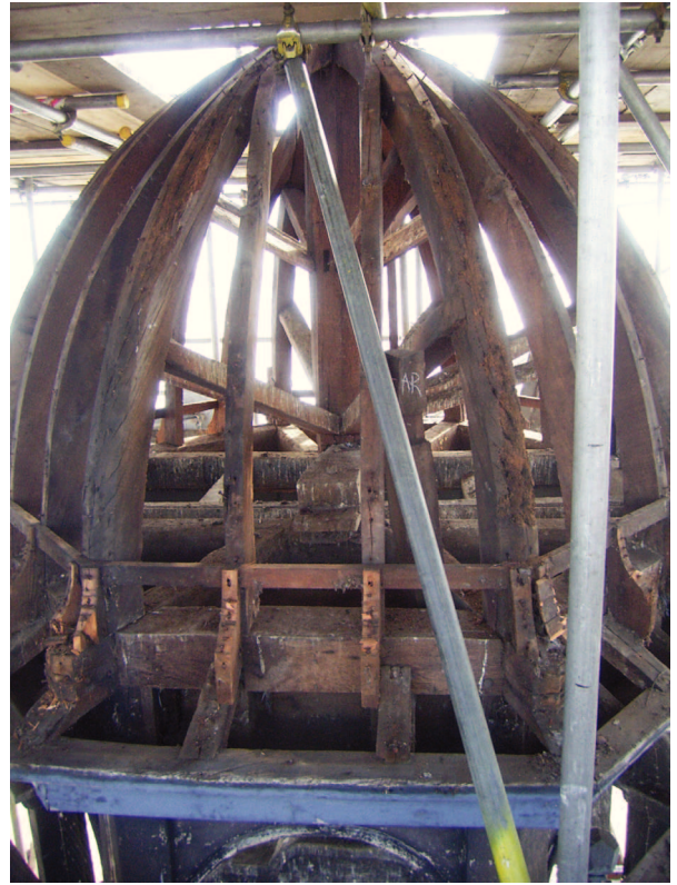
Plate 40: lantern cap frame following removal of lead and sarking boards
