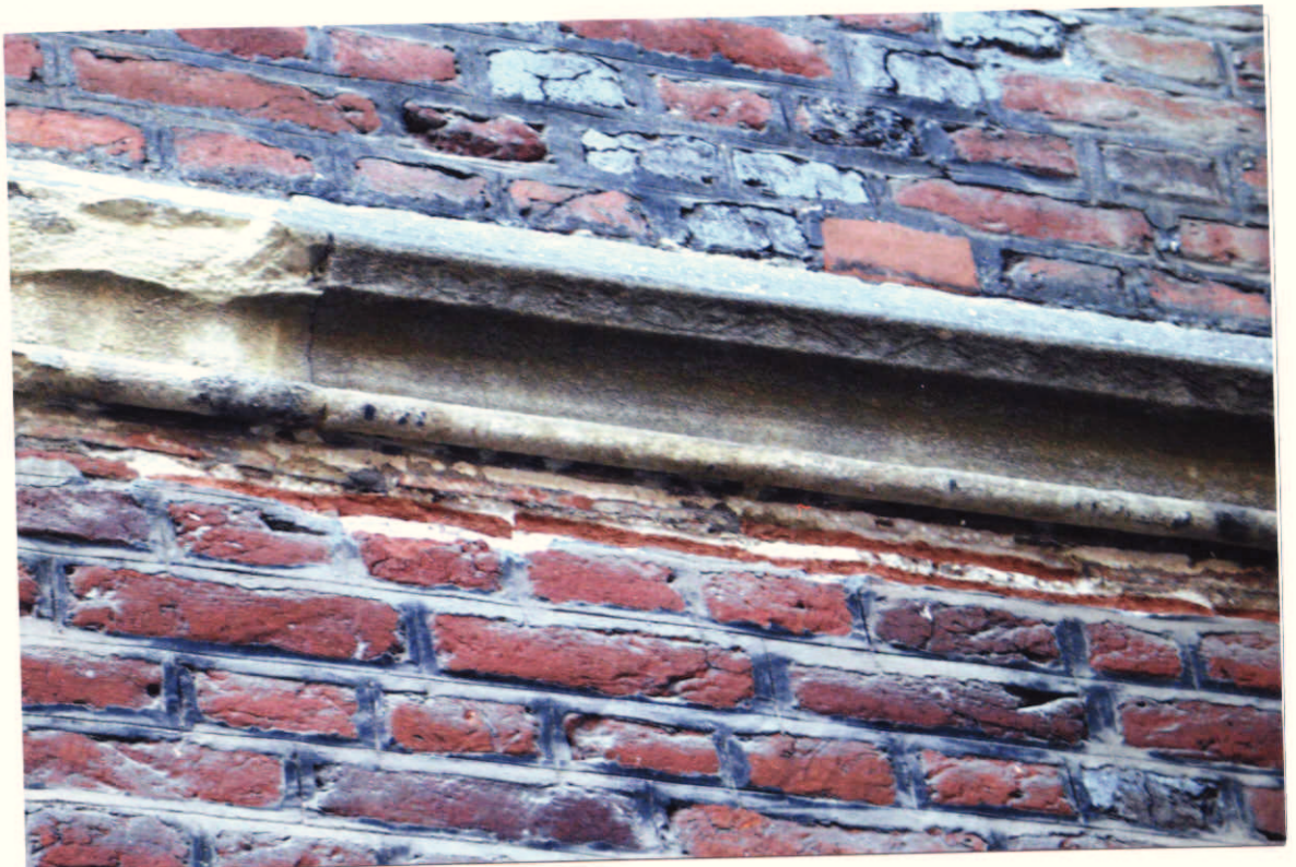
Plate 13. Clock Court. Tile levelling course below Wheatley Limestone string course.
