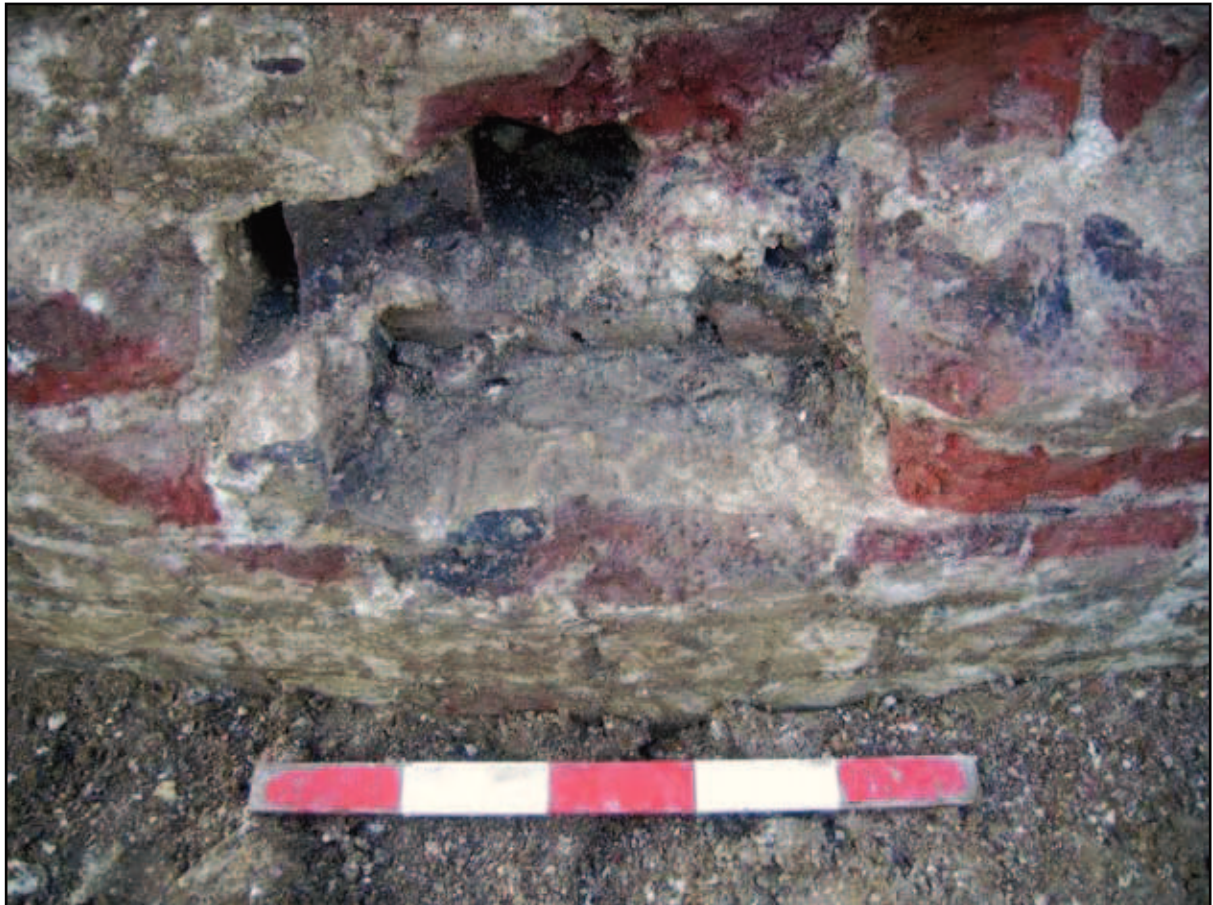
Plate 5: Trench 2. Elevation view of recess for horizontal support in wall 3001, looking north-west
