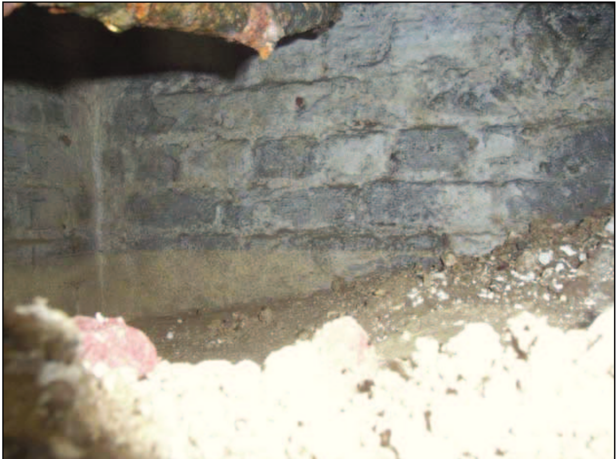
Plate 14: Trench 2. Walls within void
