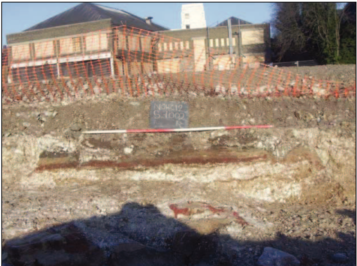
Plate 34: Trench 7. Section view, showing 737, looking north
