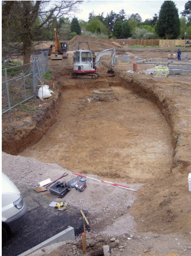
Plate 1: General view of the northern end of the access road strip, map and sample area
