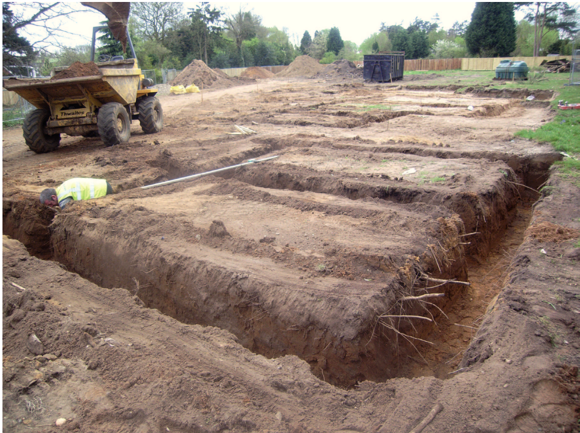
Plate 2: General view of the site after excavation of foundation trenches
