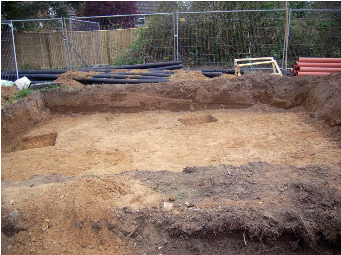
Plate 4: Soakaway pit RS3 from the north-west
