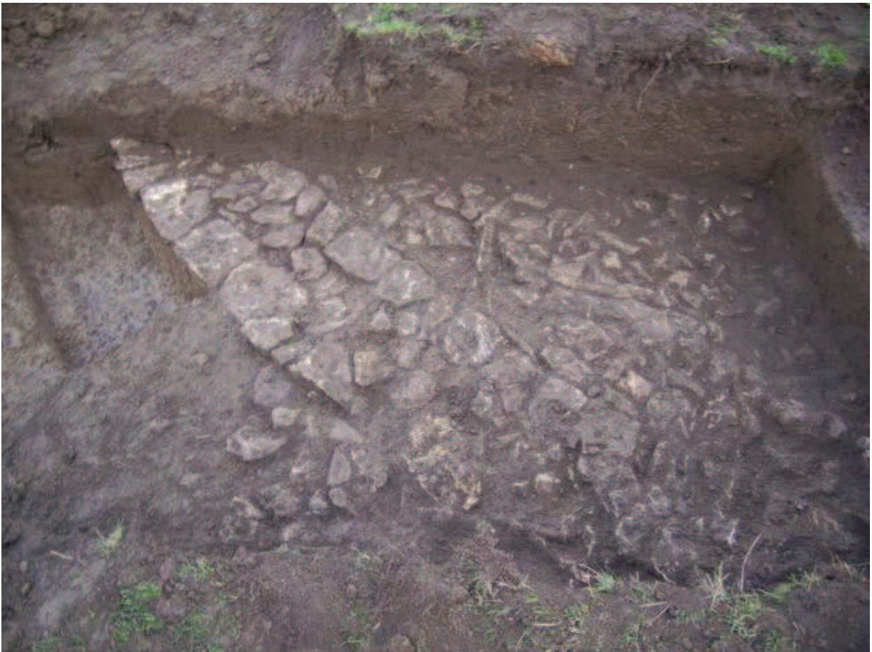
Plate 10: Trench 18: wall 1814, looking north
