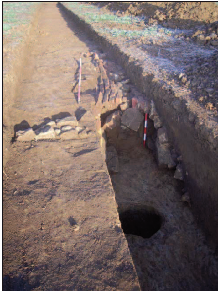
Plate 6 - Trench 87: Culvert and retaining wall
