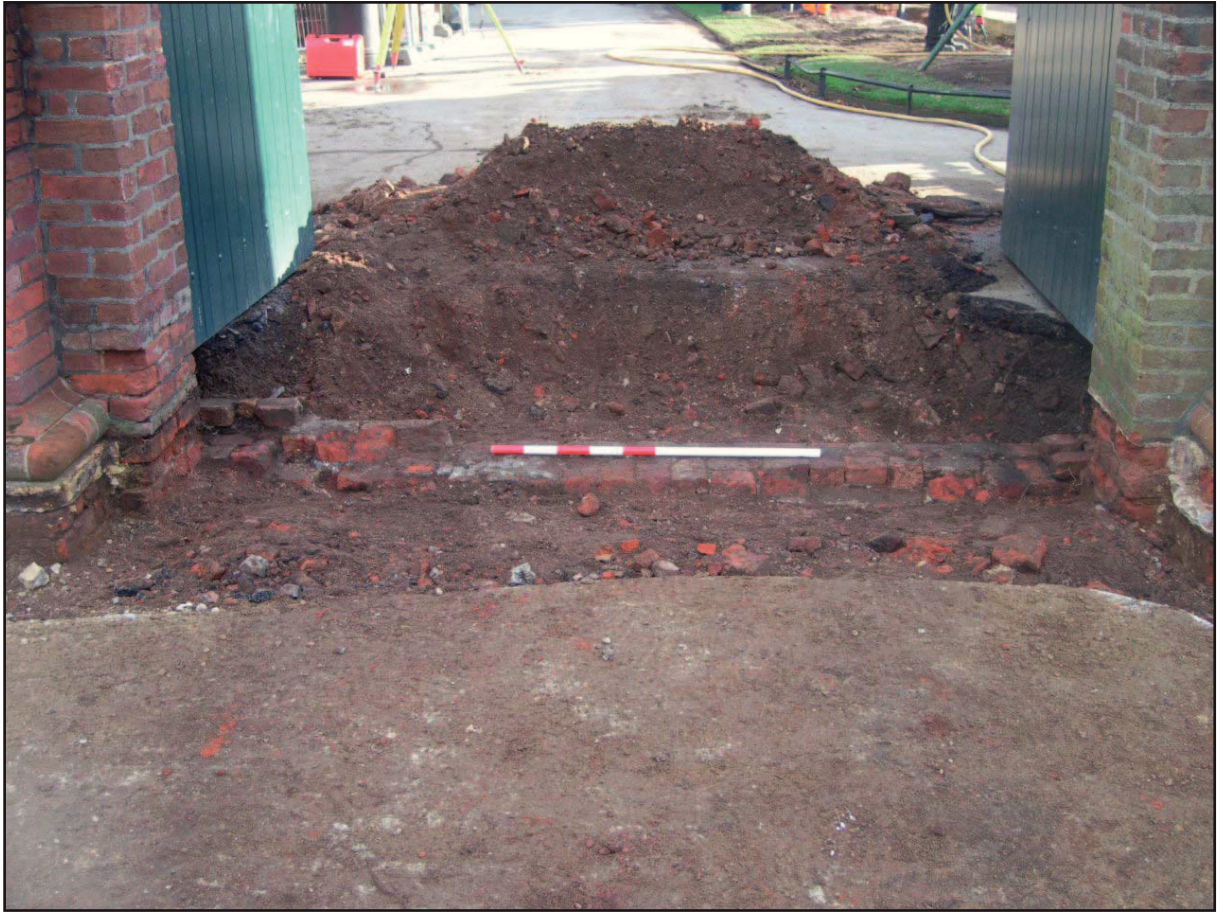
Plate 3 - Structures 102, 103 and 104 exposed within Vrow Walk Gate , Area D
