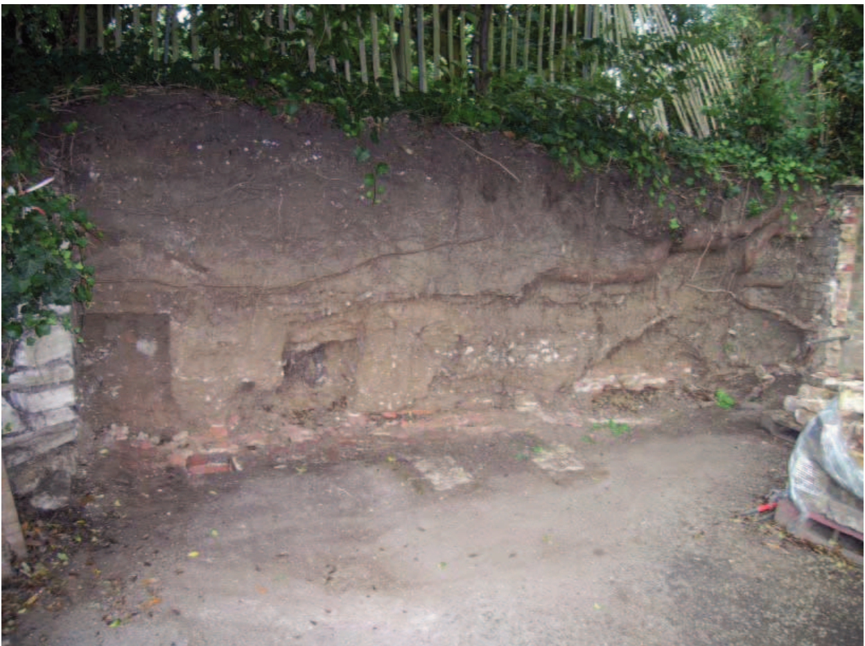
Plate 2: View of wall footings following dismantling
