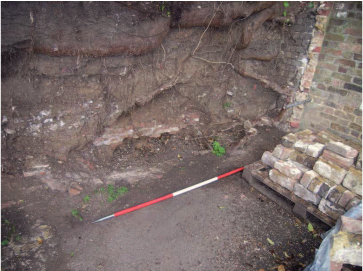
Plate 4: View of wall (east) following dismantling
