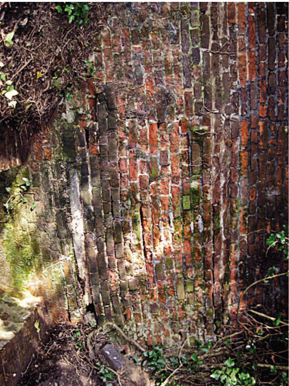
Plate 5: Historic boundary wall above water inlet, looking north
