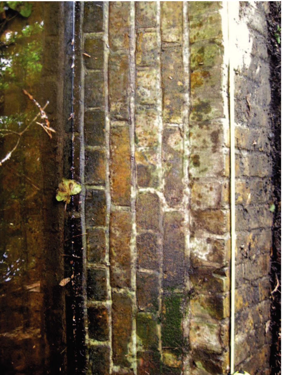
Plate 4: Detail of water inlet, looking west
