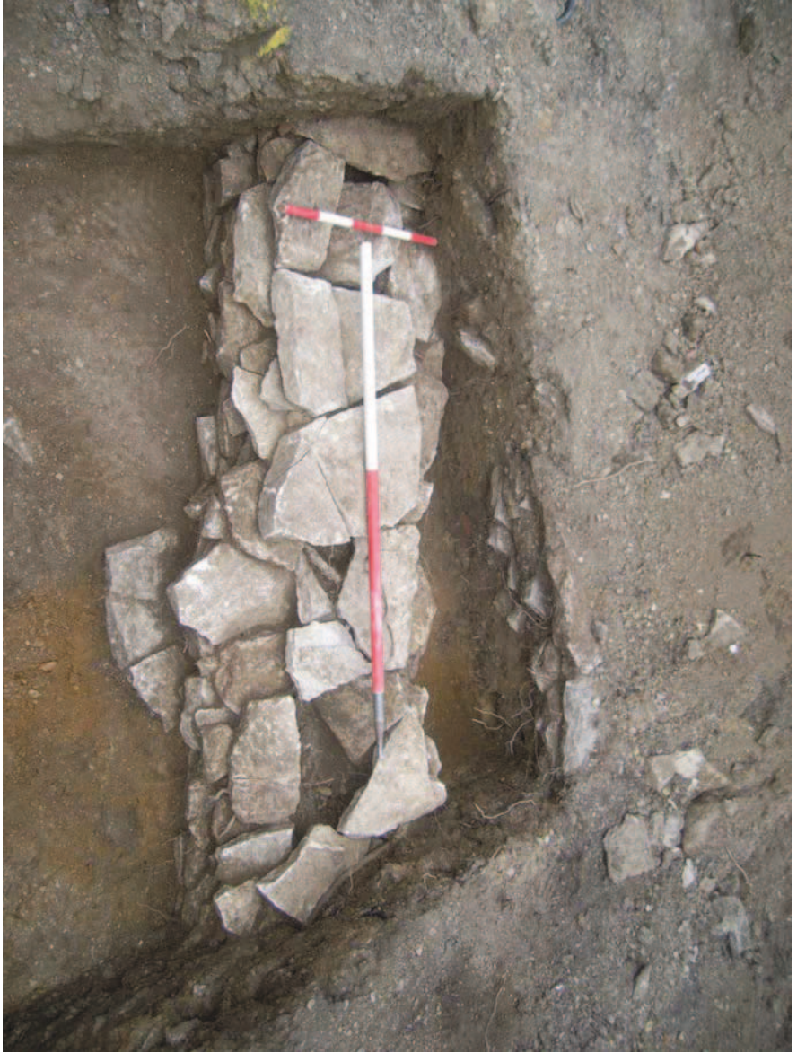
Plate 13: Stone drain 27 exposed, looking north-east
