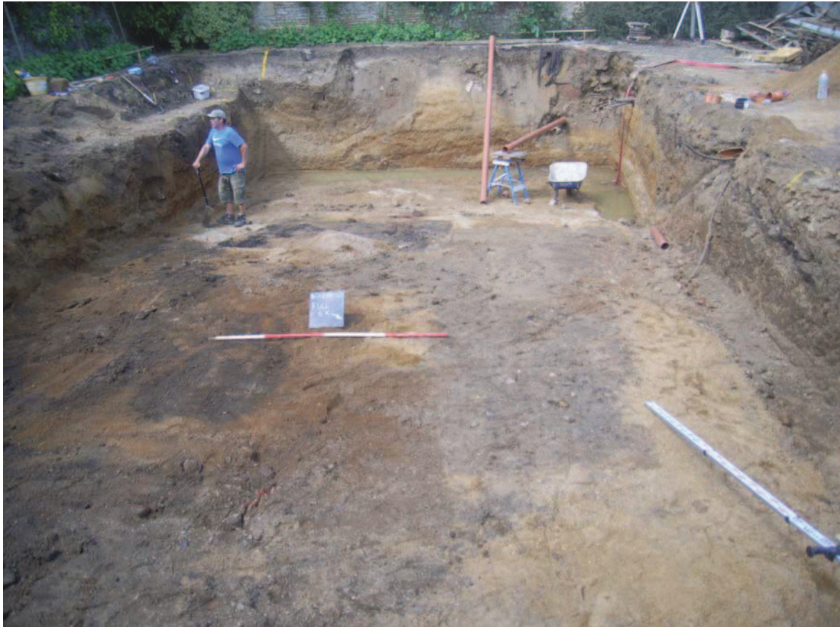
Plate 2: Swimming pool fully excavated, looking west
