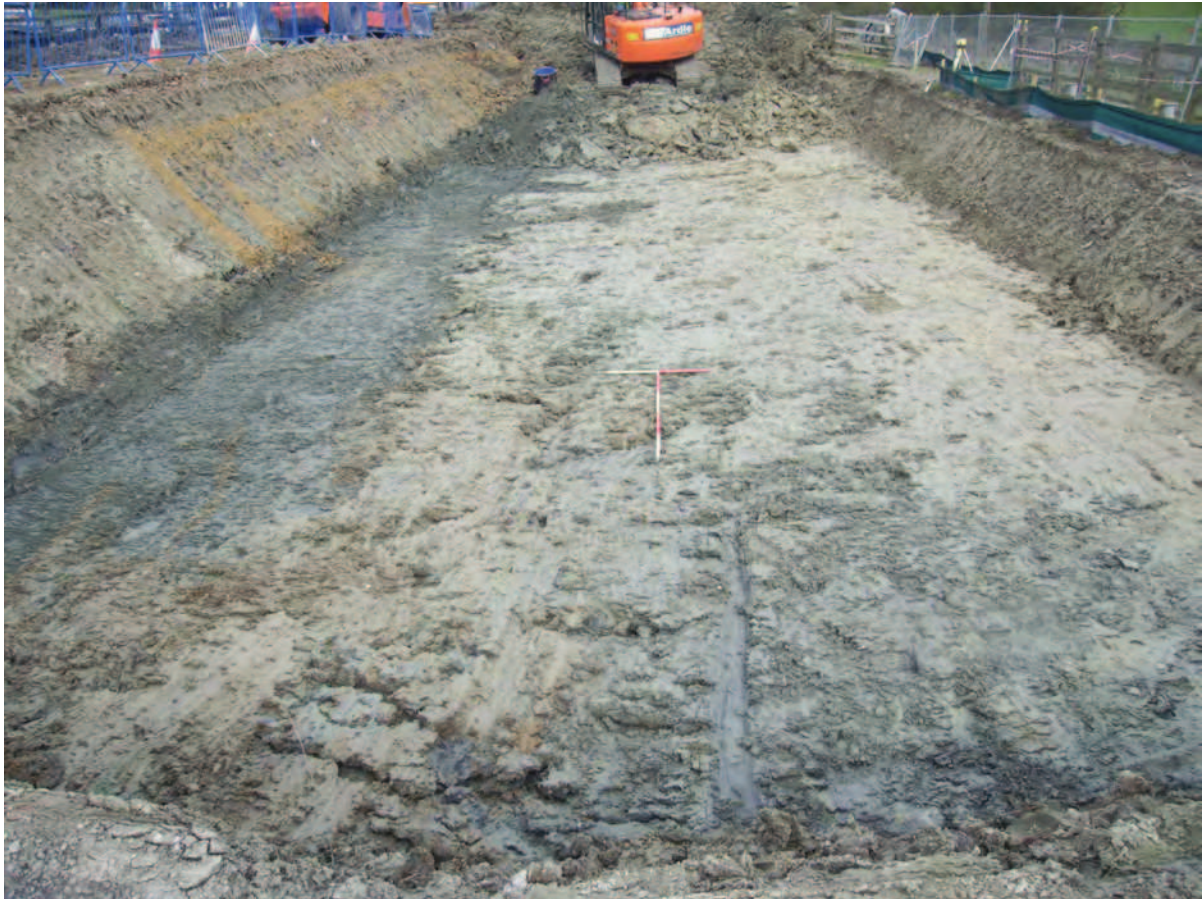
Figure 4: Excavation area to full impact depth
