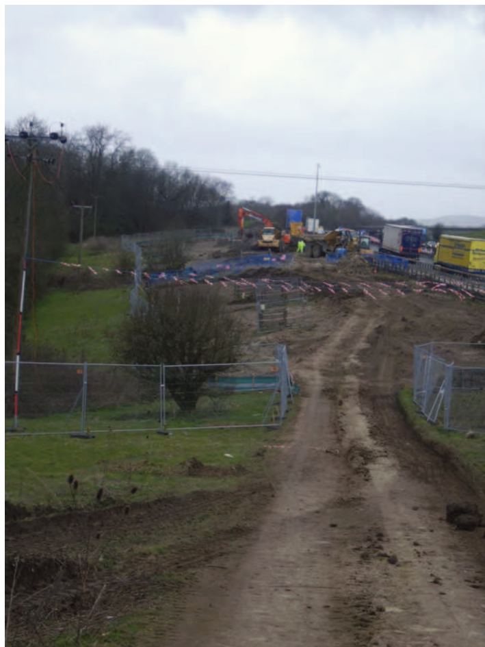
Figure 5: General view of the construction and excavation area showing the motorway embankment. View west
