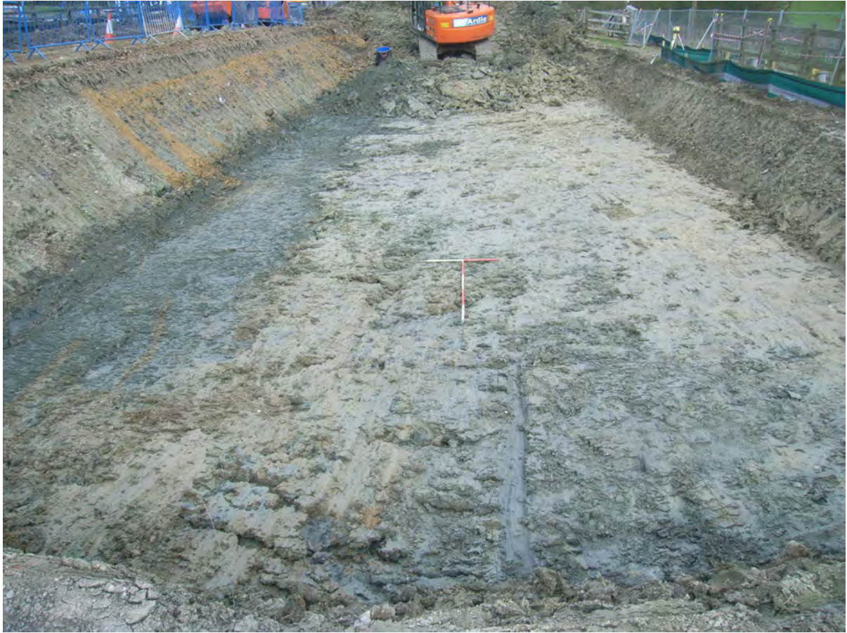
Figure 4: Excavation area to full impact depth
