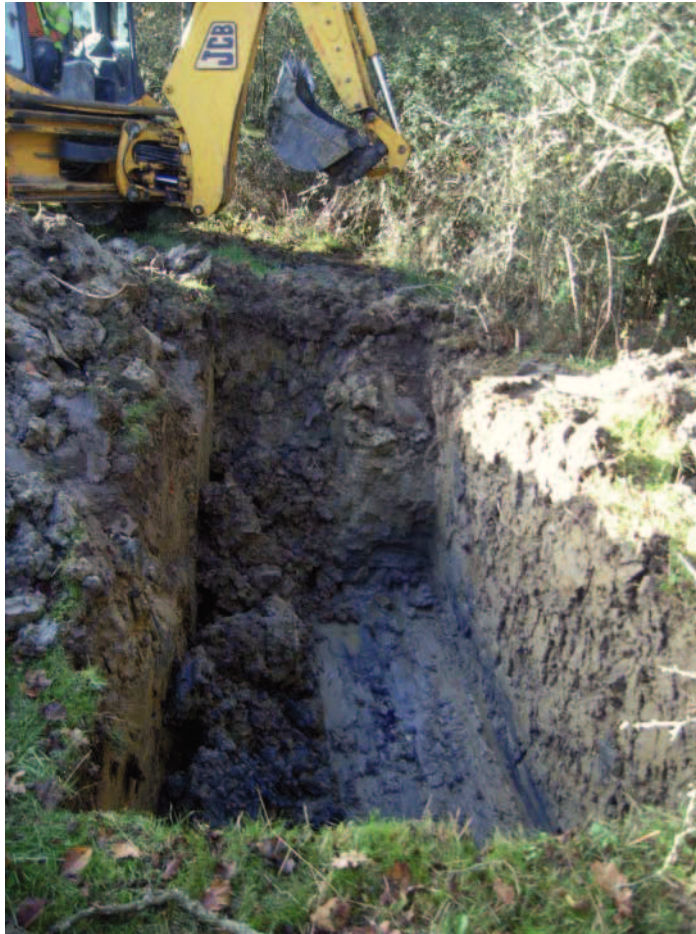
Plate 5: Replacement pole 48 excavated trench
