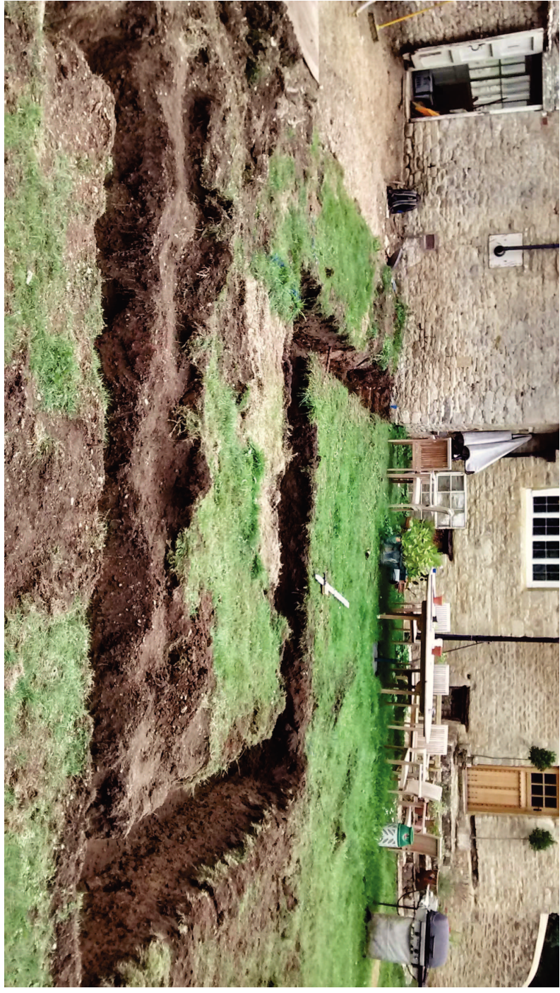
Plate 3: Foundation trenches, looking east
