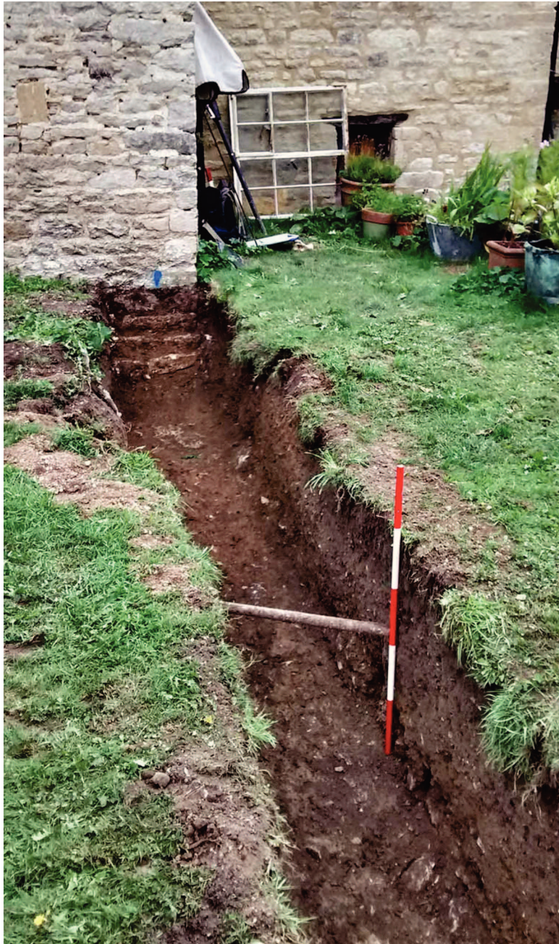
Plate 1: Foundation trench, eastern end showing wall 100, looking east
