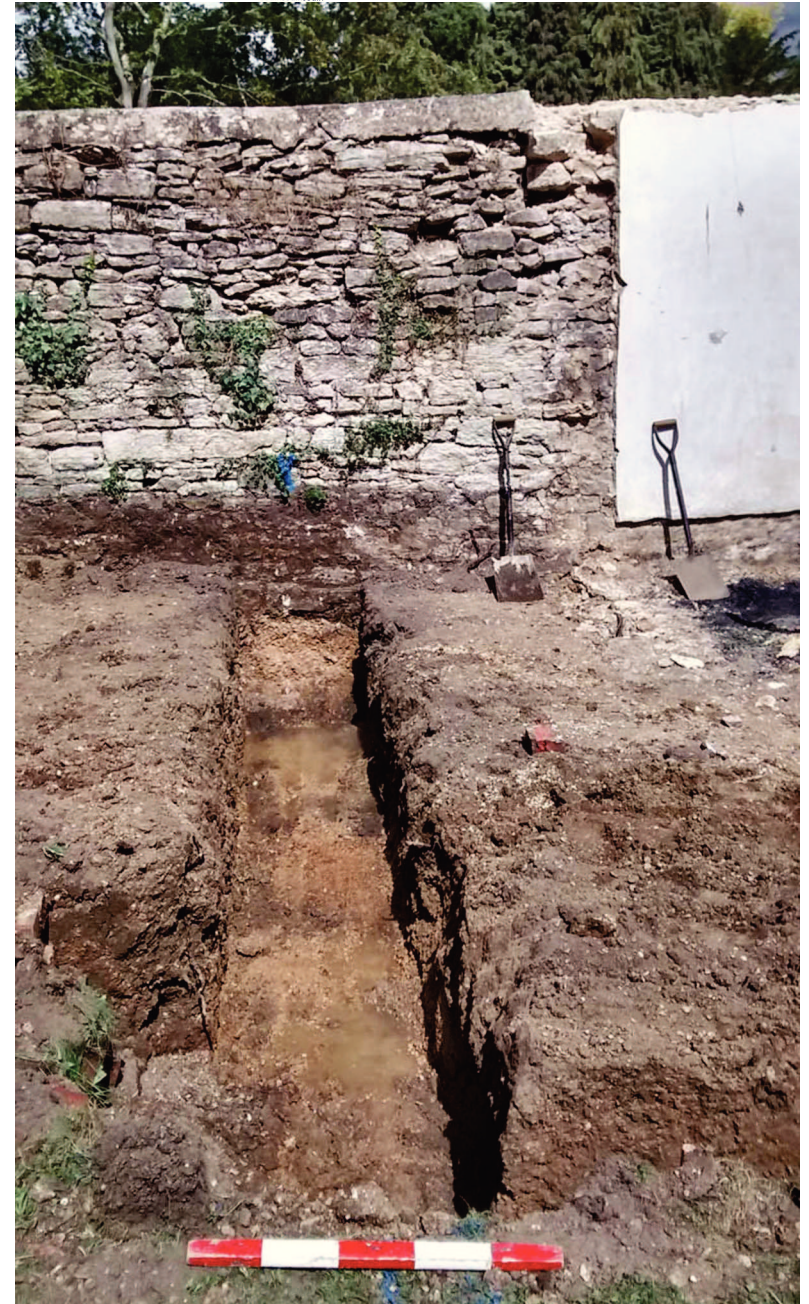
Plate 2: Foundation trench, northern end showing wall 117, looking west
