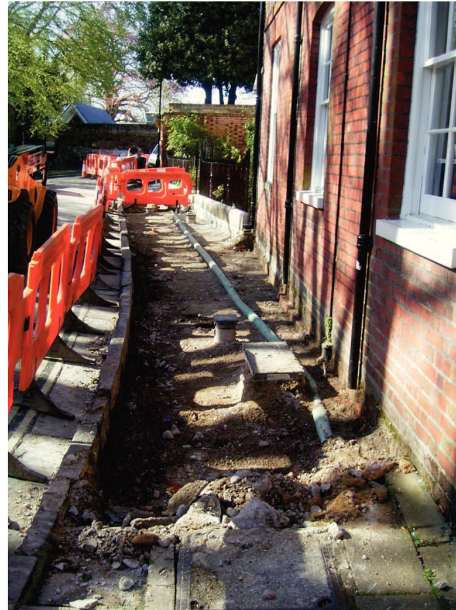
Plate 2: Pavement opposite Minster House at formation level - looking S
