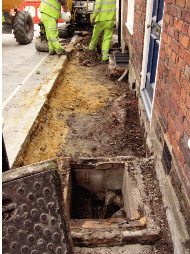
Plate 3: Pavement opposite Nos 1-2 Great Minster Street at formation level - looking N
