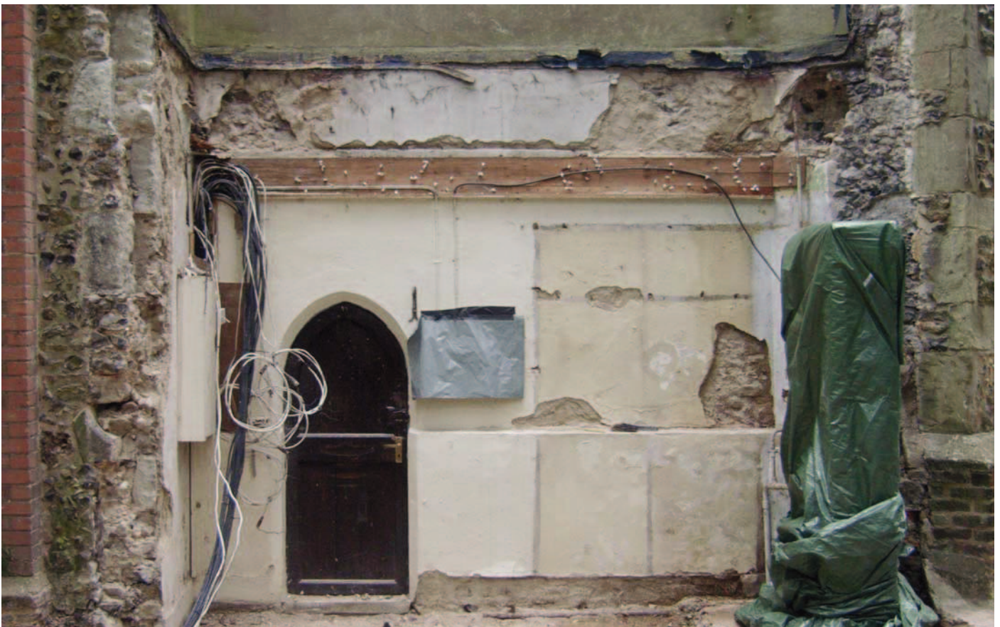
Plate 2: North wall of tower in area of removed vestry
