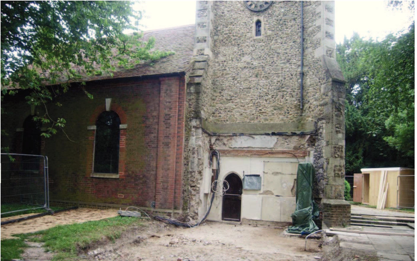
Plate 1: General view of church from NW after demolition of 1950s vestry
