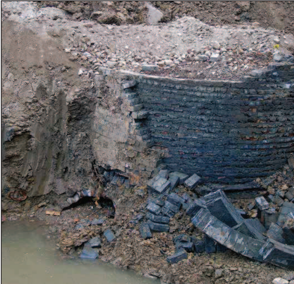
Plate 43: Shaft 8206 showing double skinned wall
