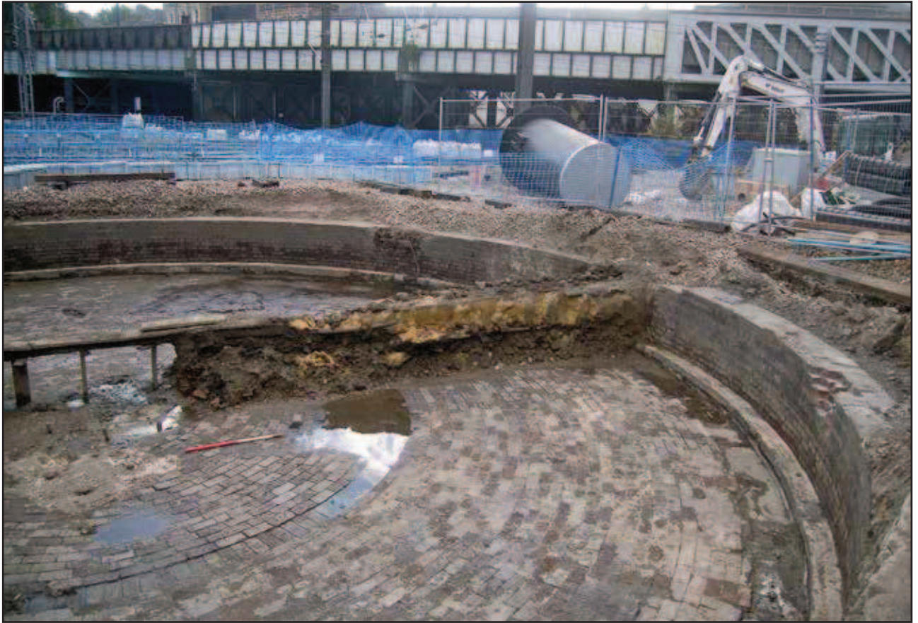
Plate 7: Overall view from north
