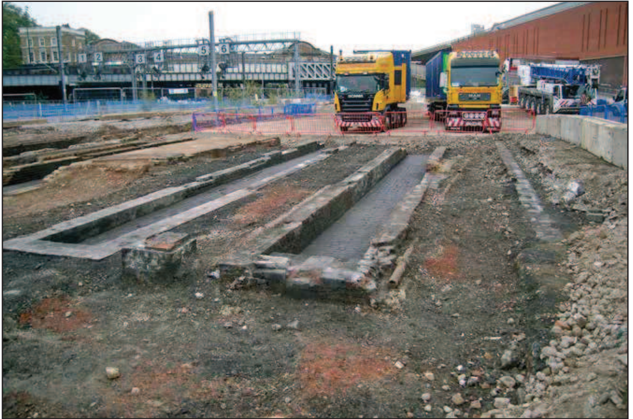
Plate 19: Inspection pits [8786] and [8785] of 1871 shed from east
