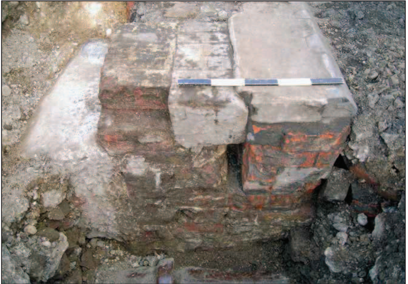
Plate 51: Section through inspection pit sidewalls the southern wall of broad gauge pit on southern sidewall of standard gauge pit
