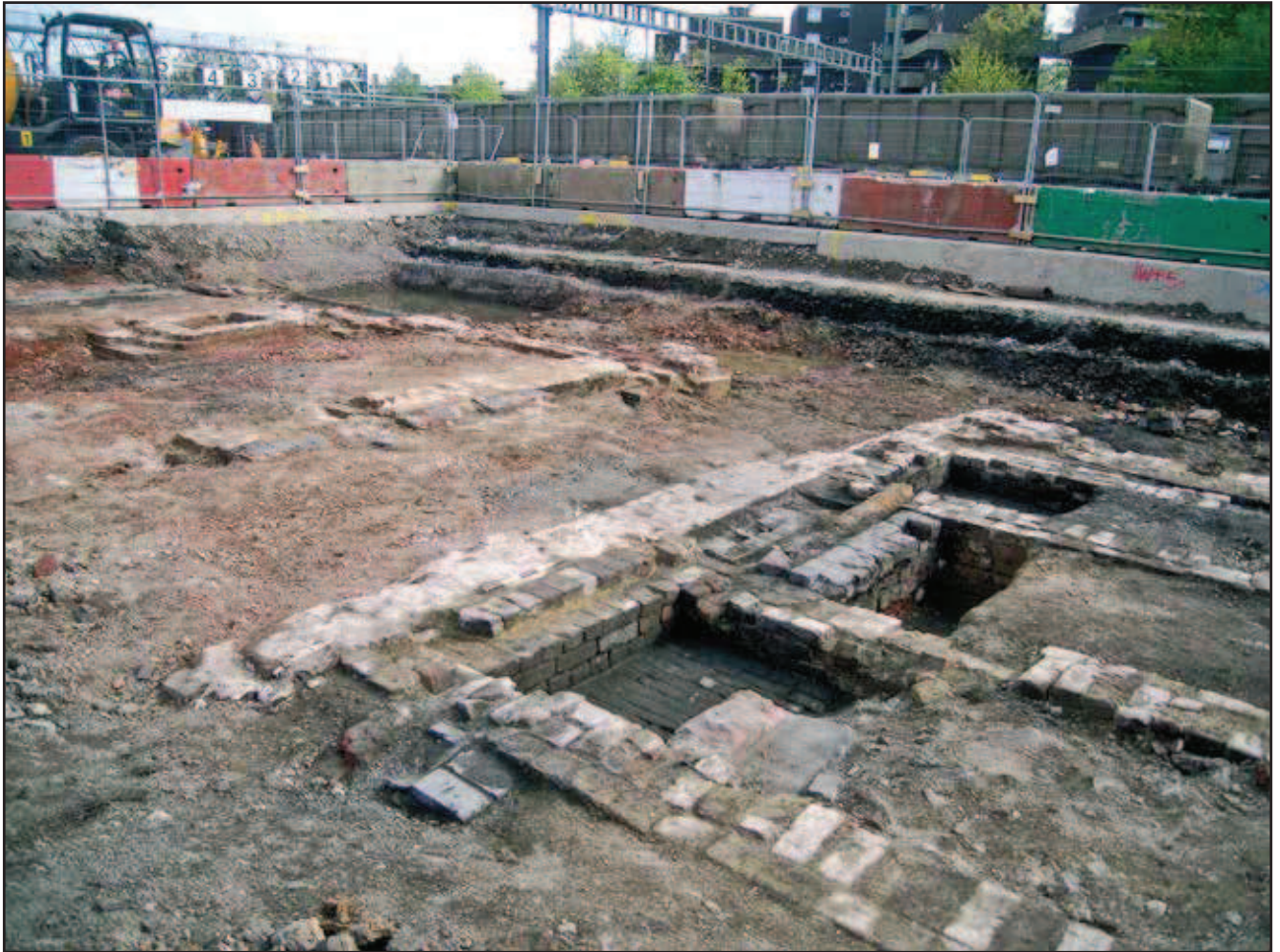
Plate 39: Inspection pits 8915 and 8916 extending into former west wing of 1852 Workshop
