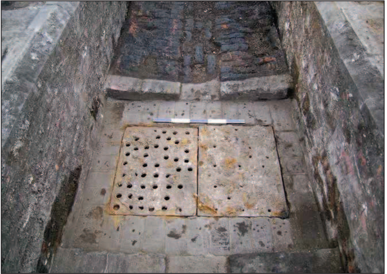
Plate 49: Catchment pit [8358] in base of inspection pit
