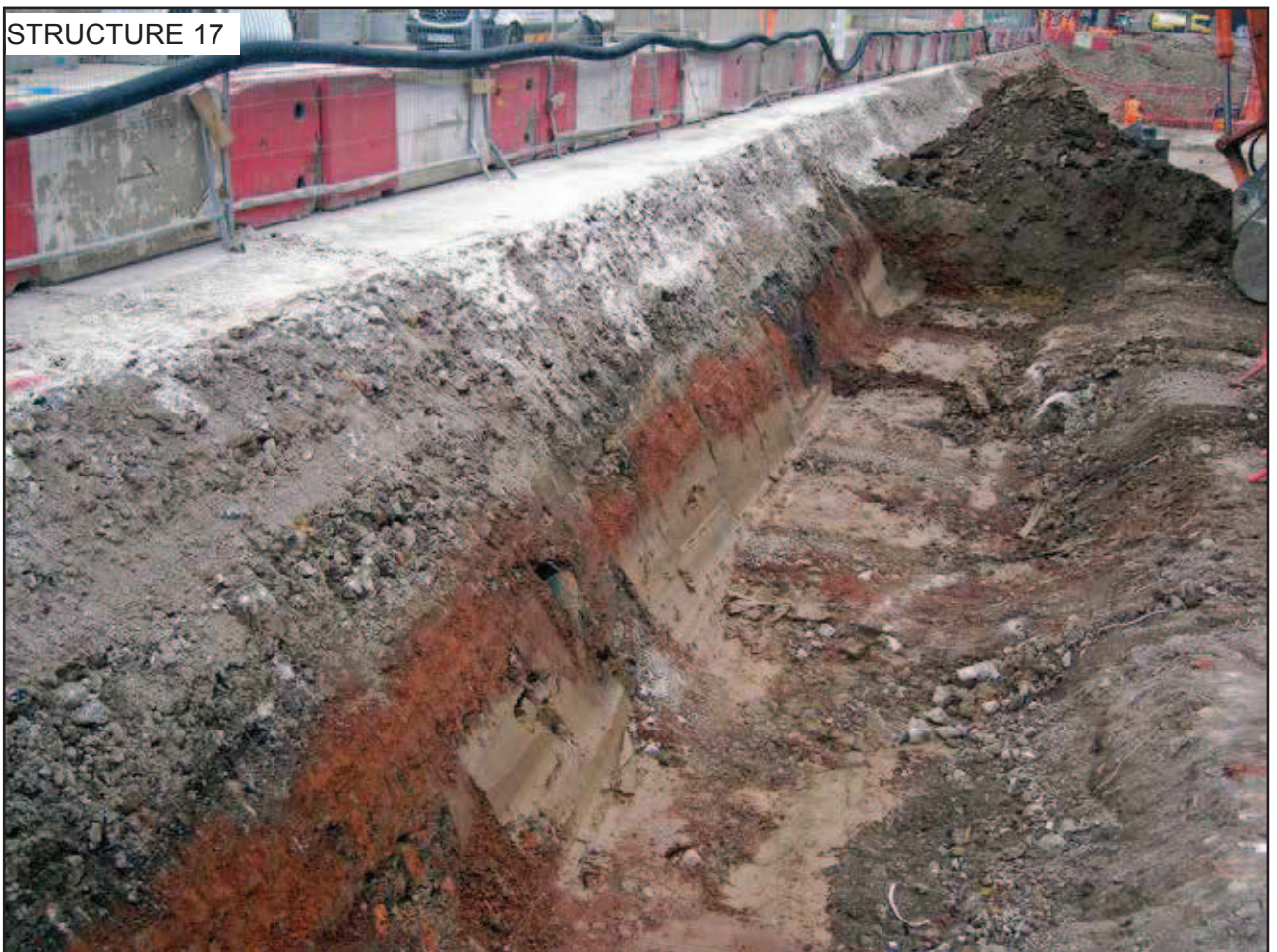
Plate 60: London Clay beneath makeup layer of crushed brick
