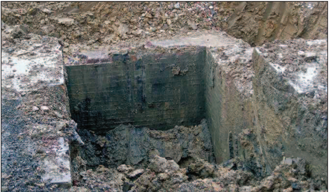
Plate 16: Brick Tank [8828] to north of 1861 shed
