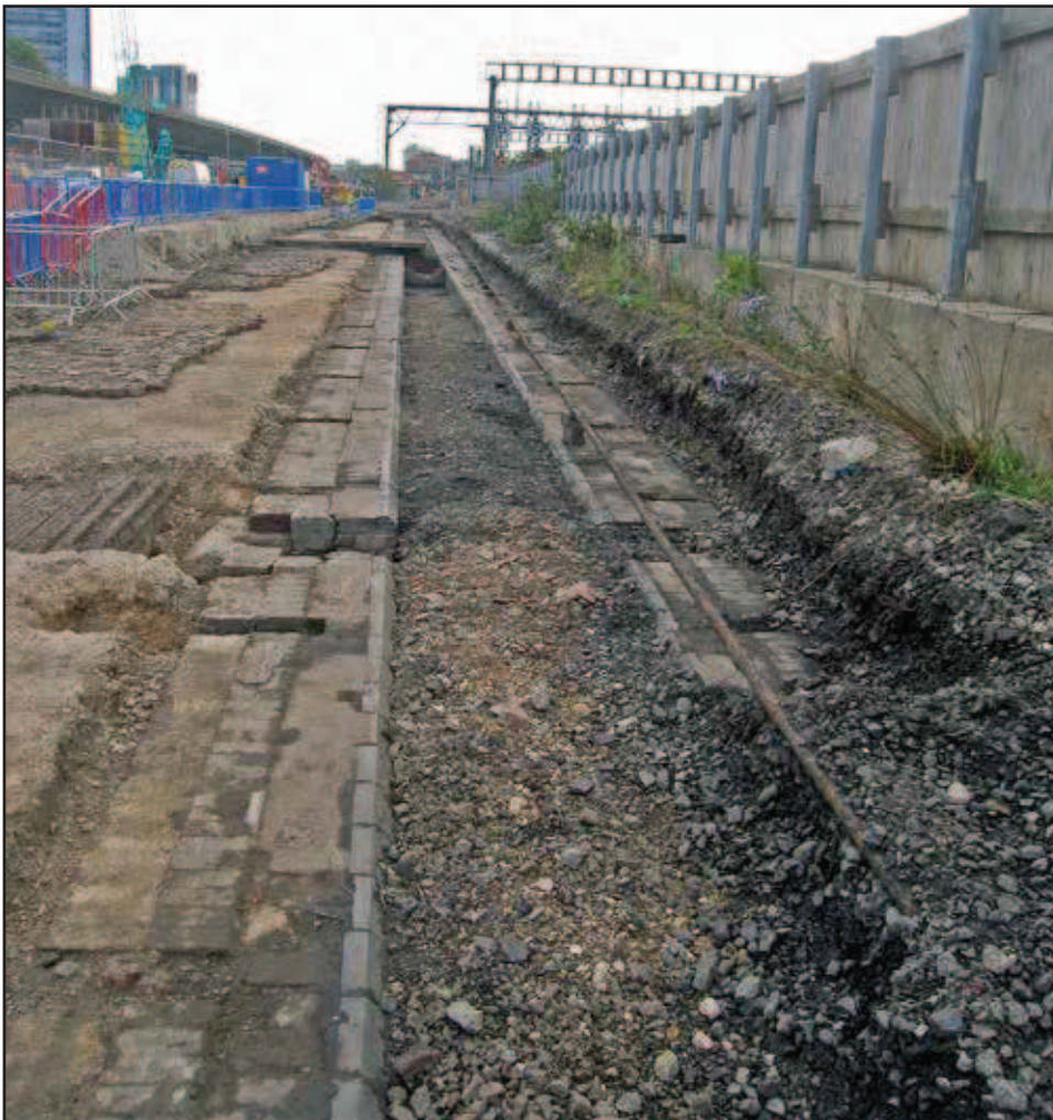
Plate 50: Partly excavated inspection pit
