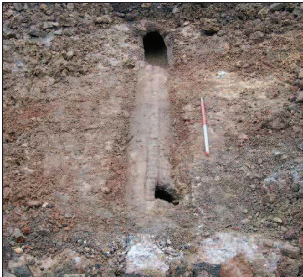
Plate 32: Conduit [8153] beneath 1852 Workshop's "Store Rooms"
