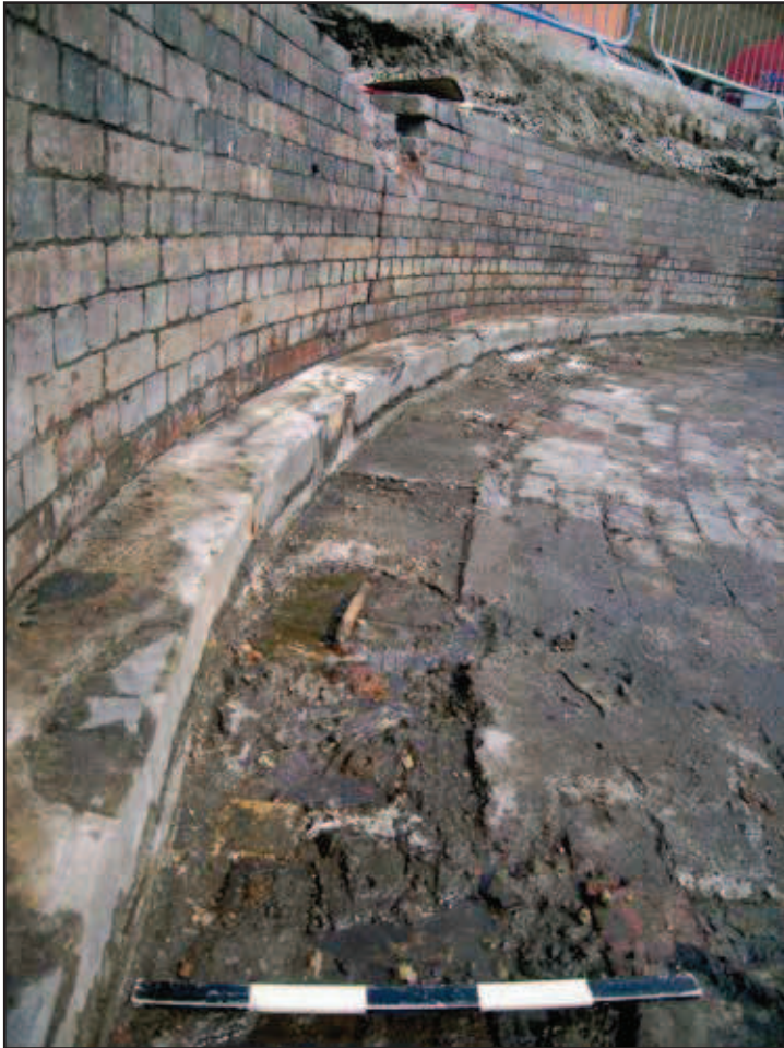
Plate 3: Guide rail gully [8523] and pit sidewall [8521]
