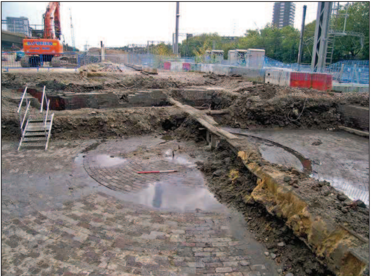
Plate 2: Turntable pit floor [8524] and drainage gully [8525]
