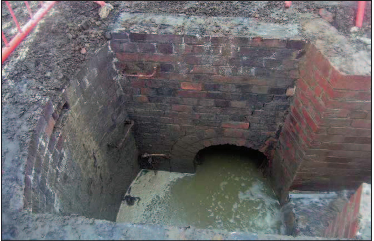
Plate 55: Access chamber [8897] and entrance to Marcon Sewer [8898]
