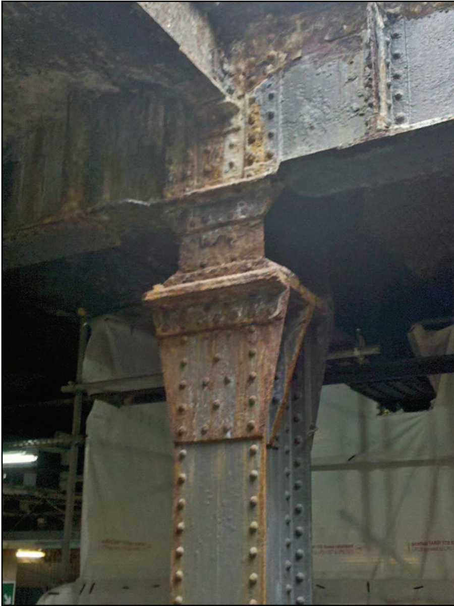
Plate 21: Supporting stanchion of Milk Ramp/Red Star Deck
