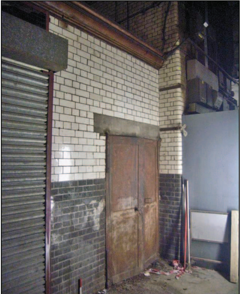
Plate 28: Variation in Brick Bond Associated with Steel Roller Door
