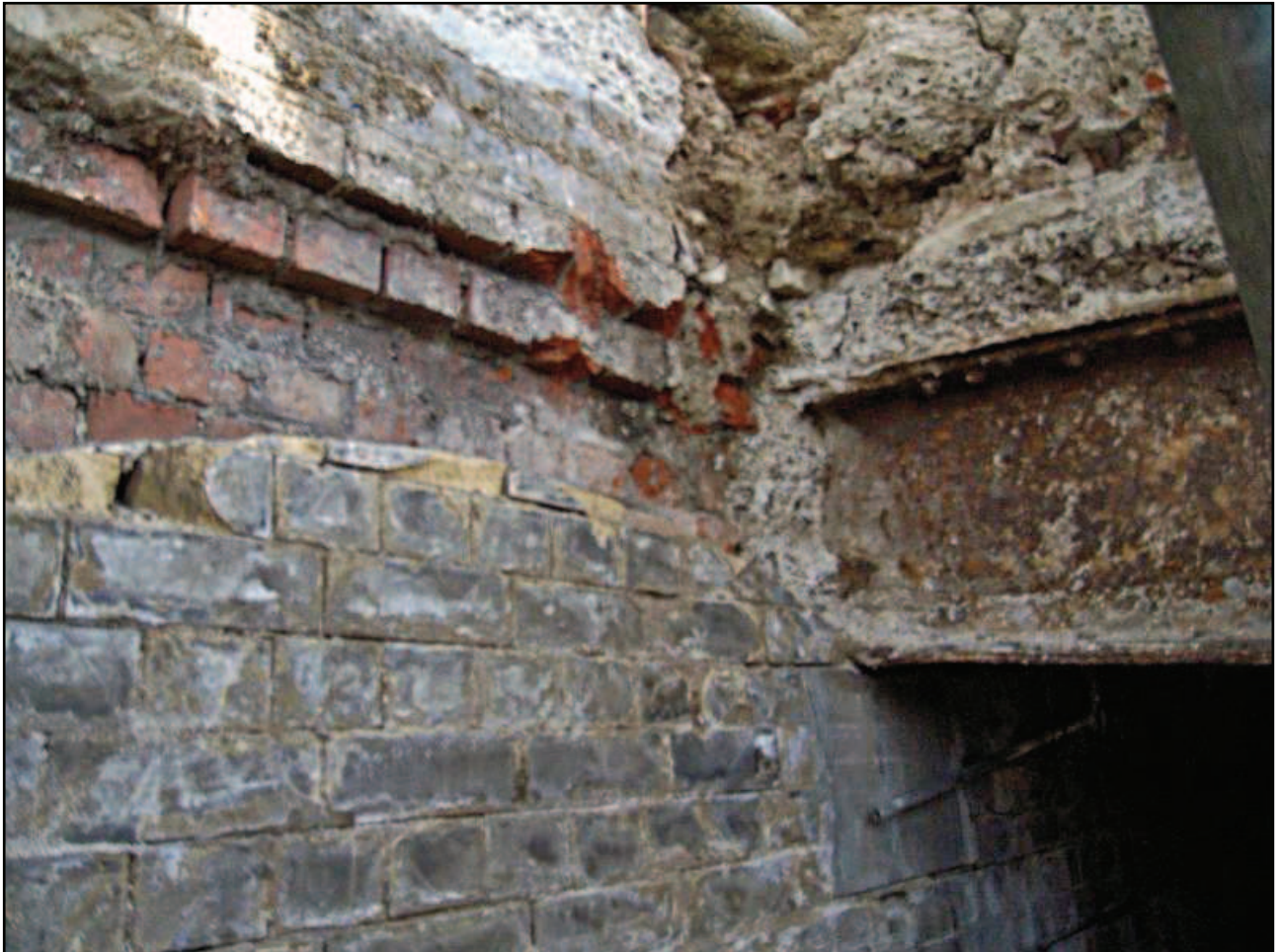
Plate 20: Steel girders within Milk Ramp and northern wall of Ramp. Looking north
