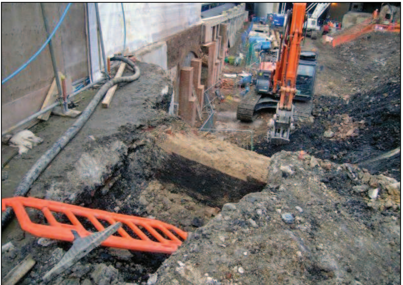
Plate 4: Removal of the walls of 2021. Looking north-west
