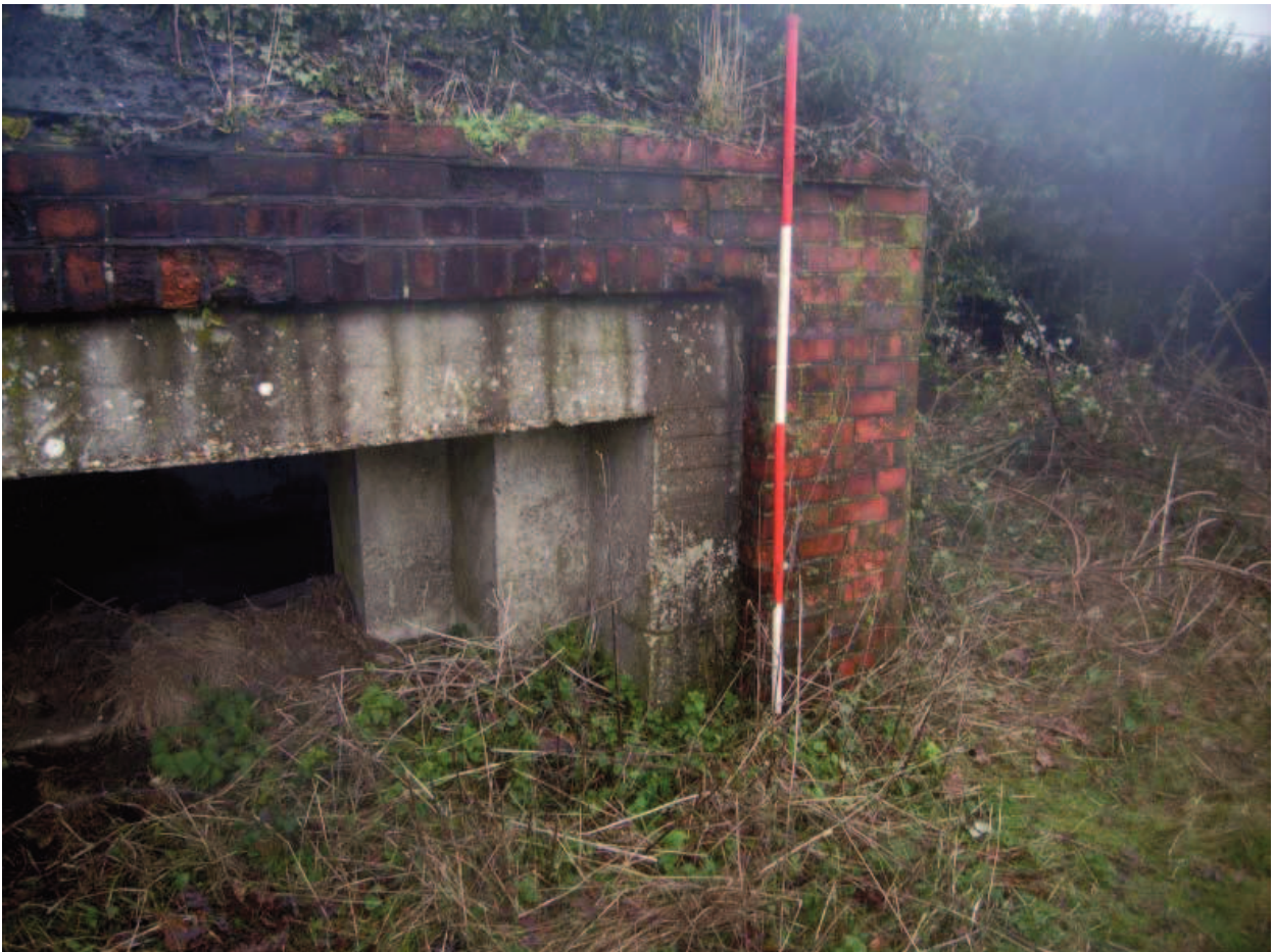
Plate 4: Detail of south-west wall
