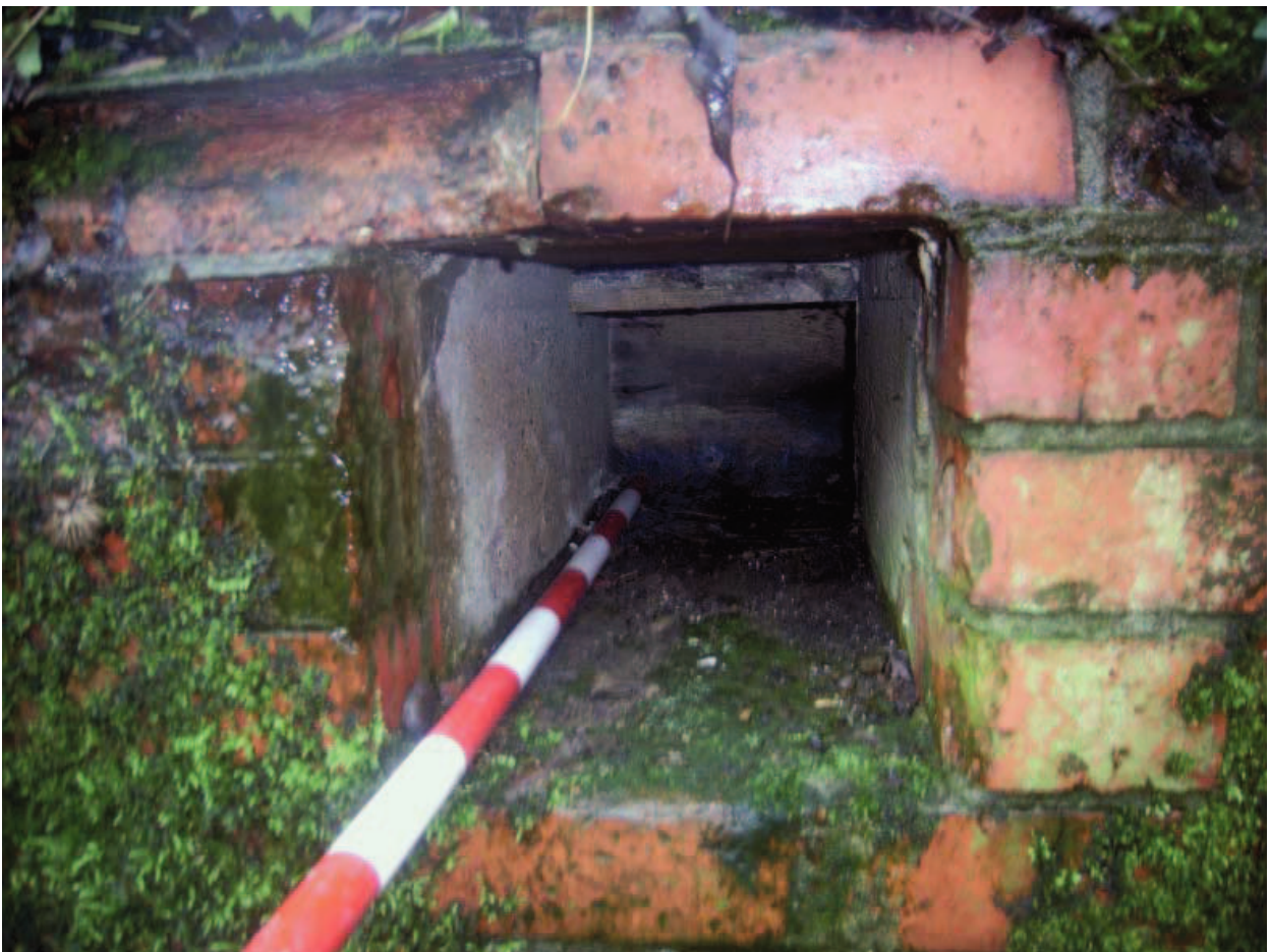
Plate 20: Detail of vent in north-east wall
