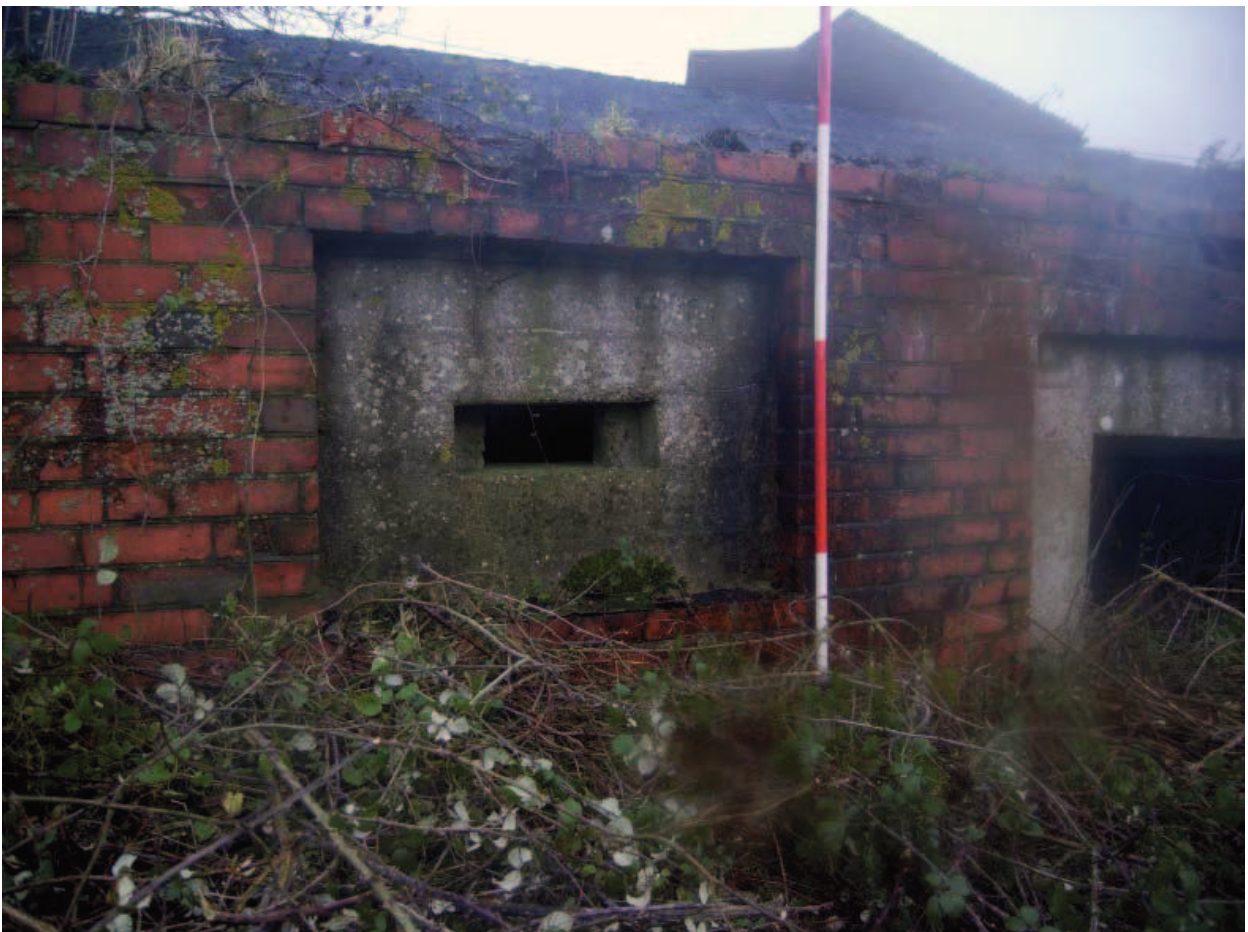
Plate 6: Detail of south-west wall
