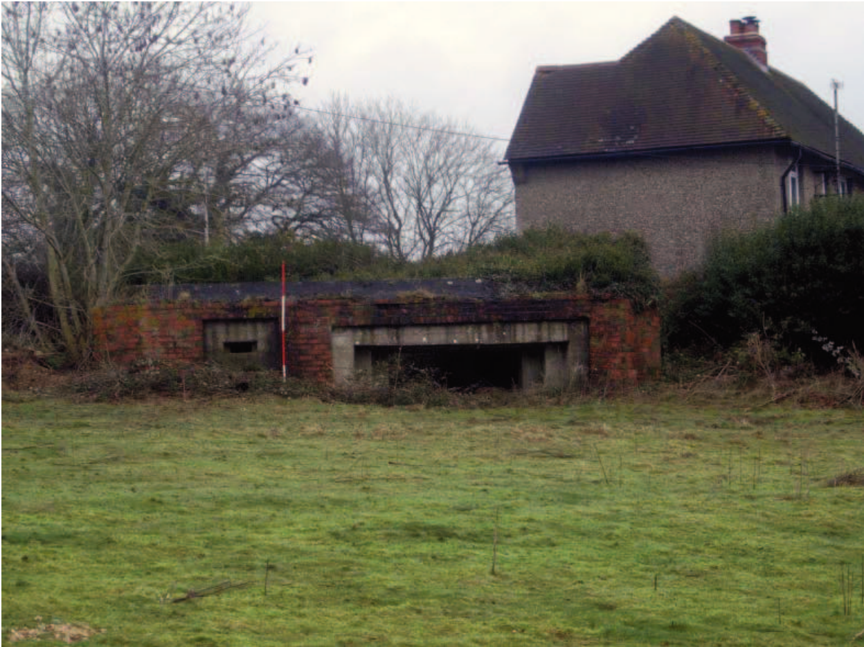
Plate 1: General view of pillbox from south-west
