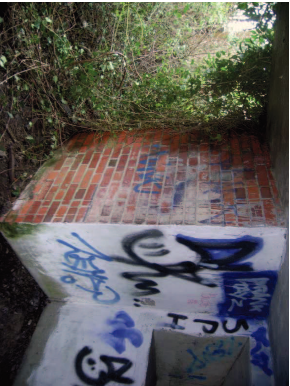
Plate 26: Entrance in SE room
