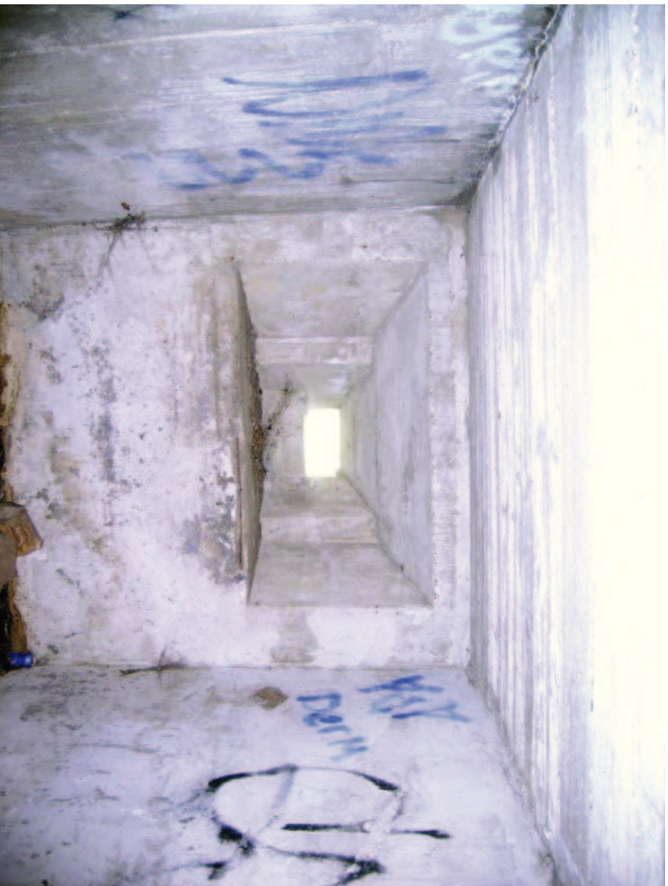
Plate 25: NW room looking SW
