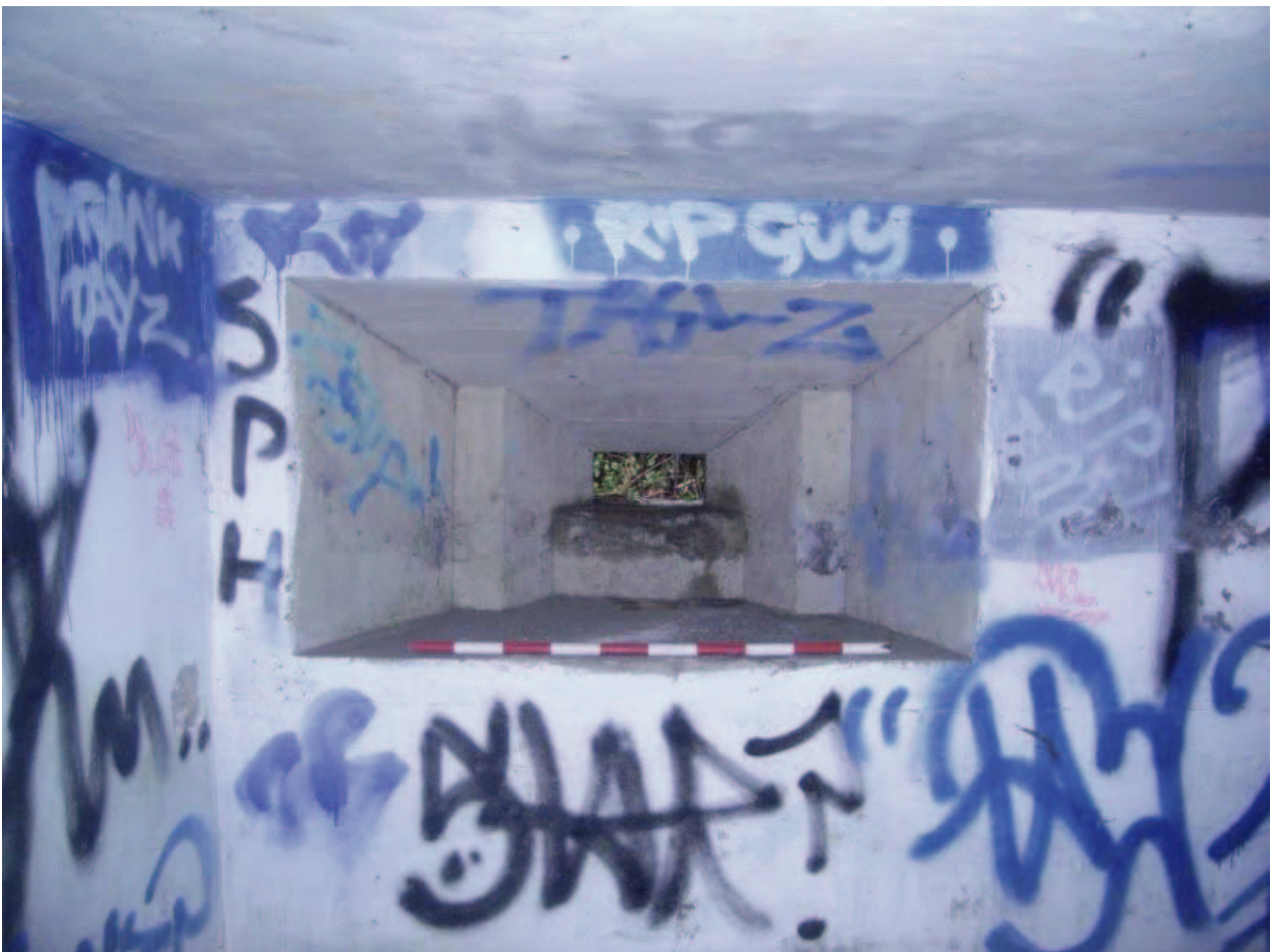
Plate 28: Loop detail in SE room looking SE
