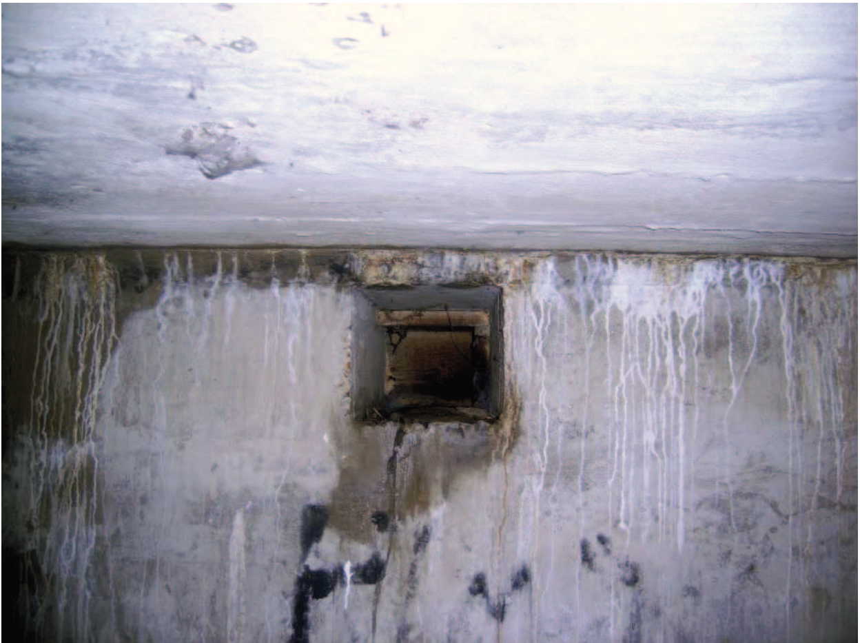
Plate 32: Vent in NE wall
