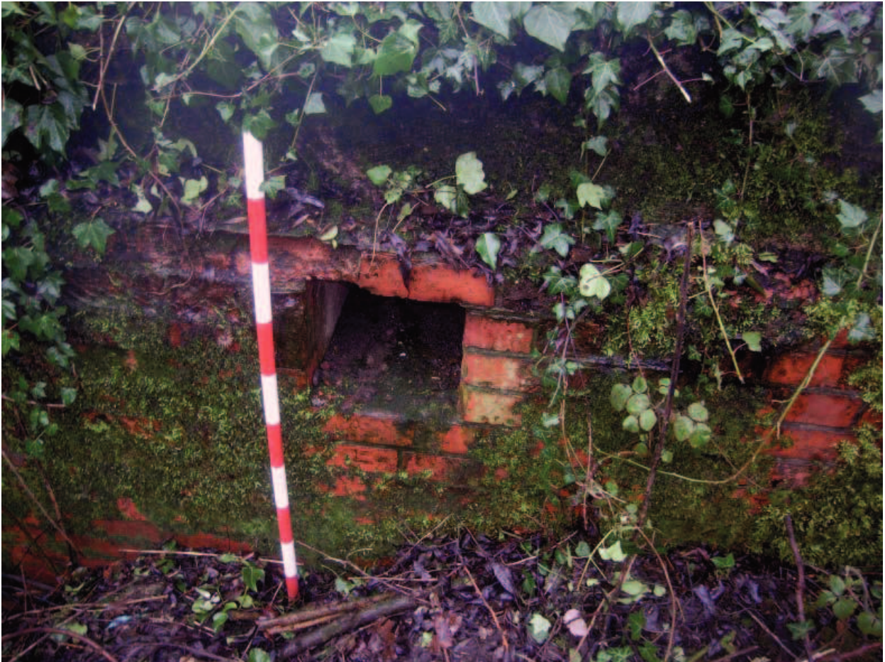
Plate 19: Detail of vent in north-east wall
