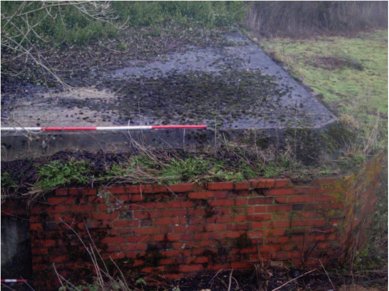
Plate 9: Detail of roof from north-west
