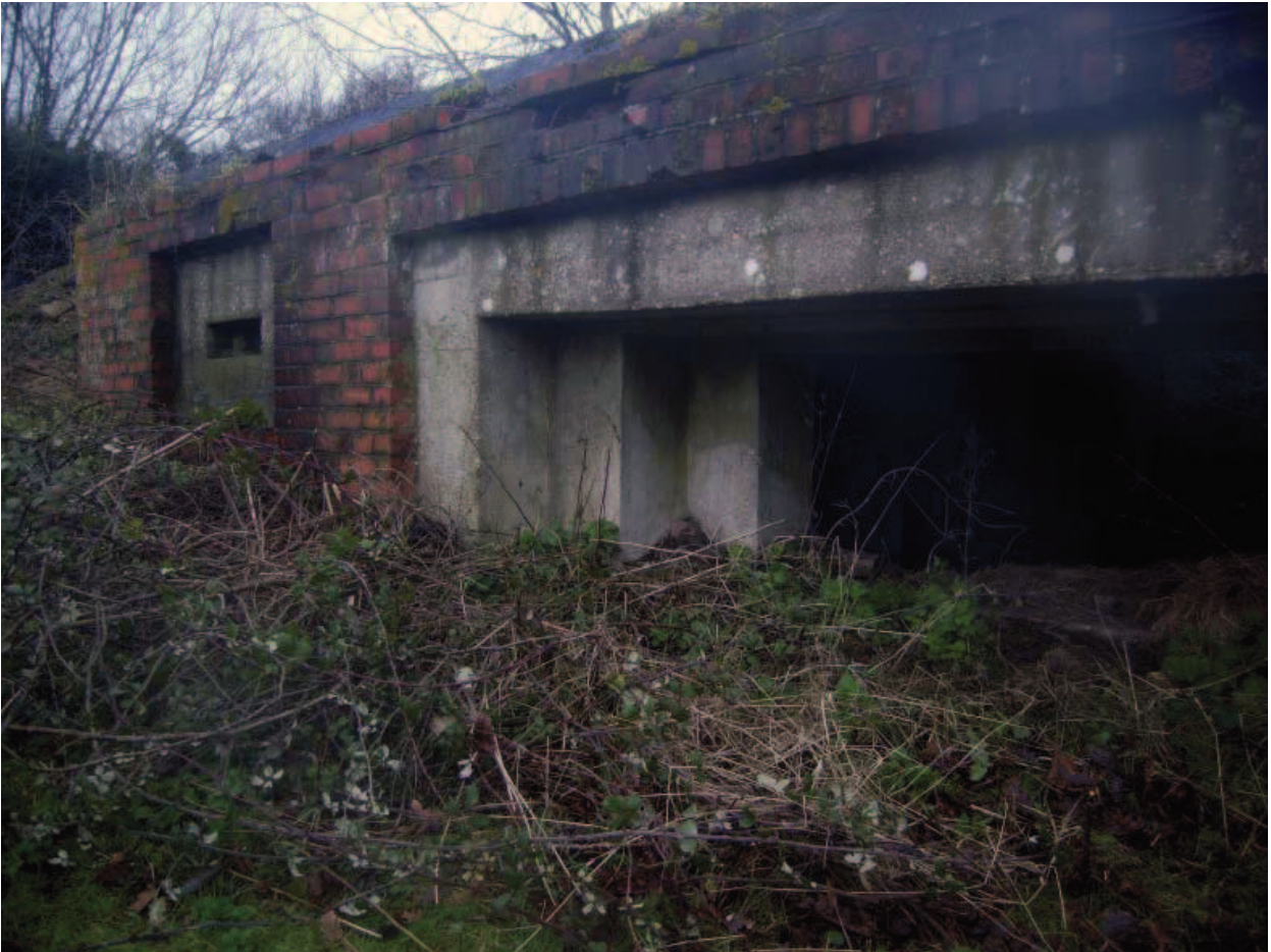
Plate 5: Detail of embrasure in SW wall
