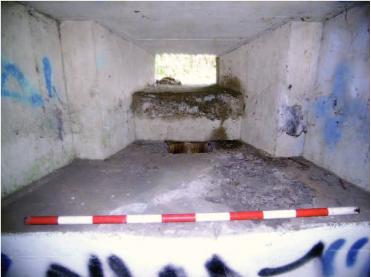
Plate 27: Loop detail in SE room looking SE
