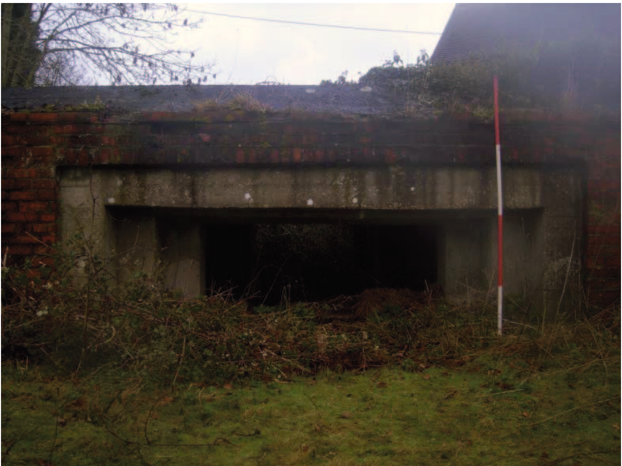
Plate 2: Main gun loop in south-west face of pillbox
