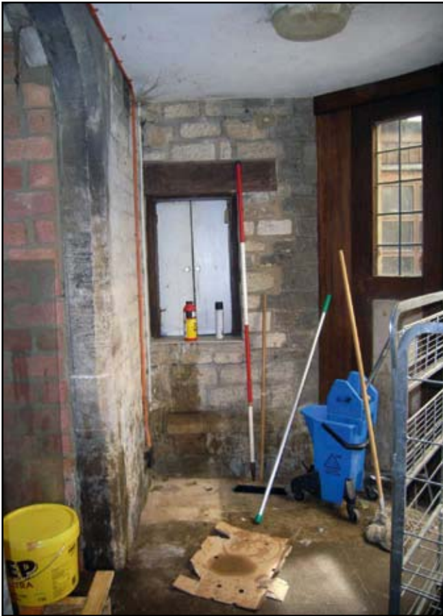
Plate 9: Internal view of porch (viewed east)
