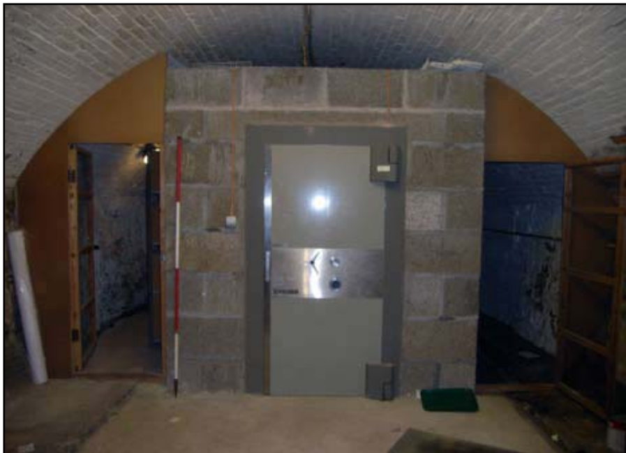
Plate 15: View of Buttery Cellar (east)
