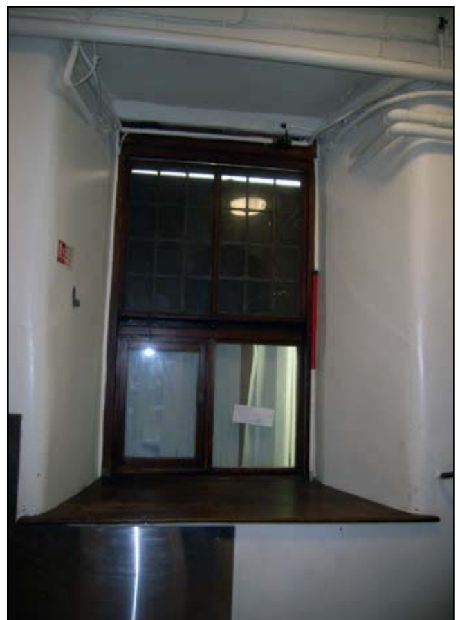
Plate 12: Detail of window within Old Kitchen block (west wall).
