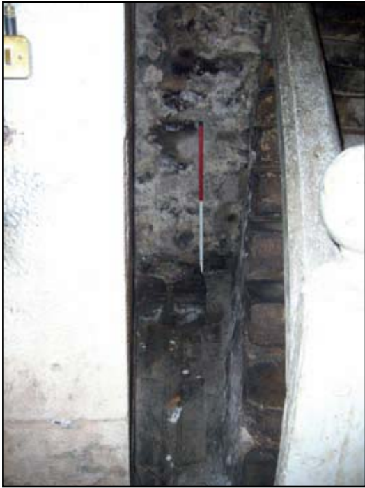
Plate 17: View of drain adjacent to Buttery Cellar stairs
