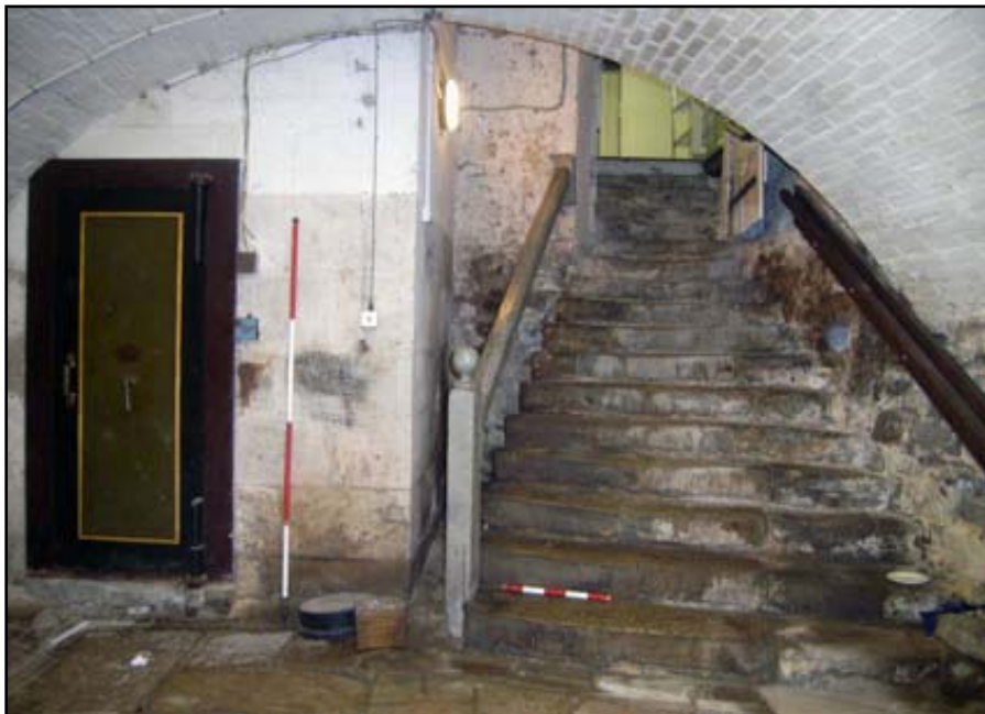
Plate 19: View of Buttery Cellar stairs
