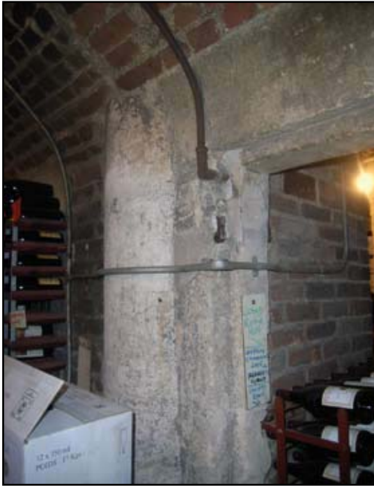
Plate 21: View of stone column in main Wine Cellar
