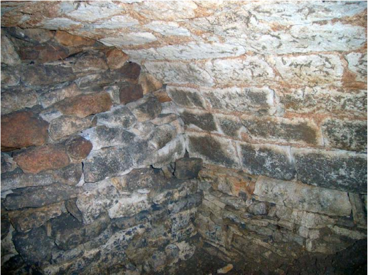
Plate 4: Test Pit 10, interior of barrel vaulted structure
