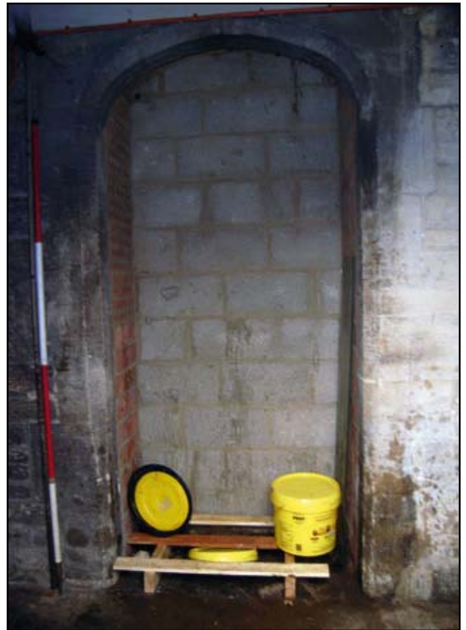
Plate 10: Detail of blocked doorway to kitchen
