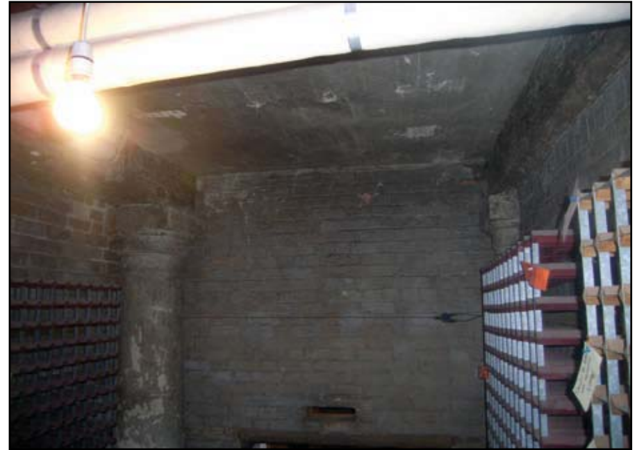
Plate 22: View of main Wine Cellar
