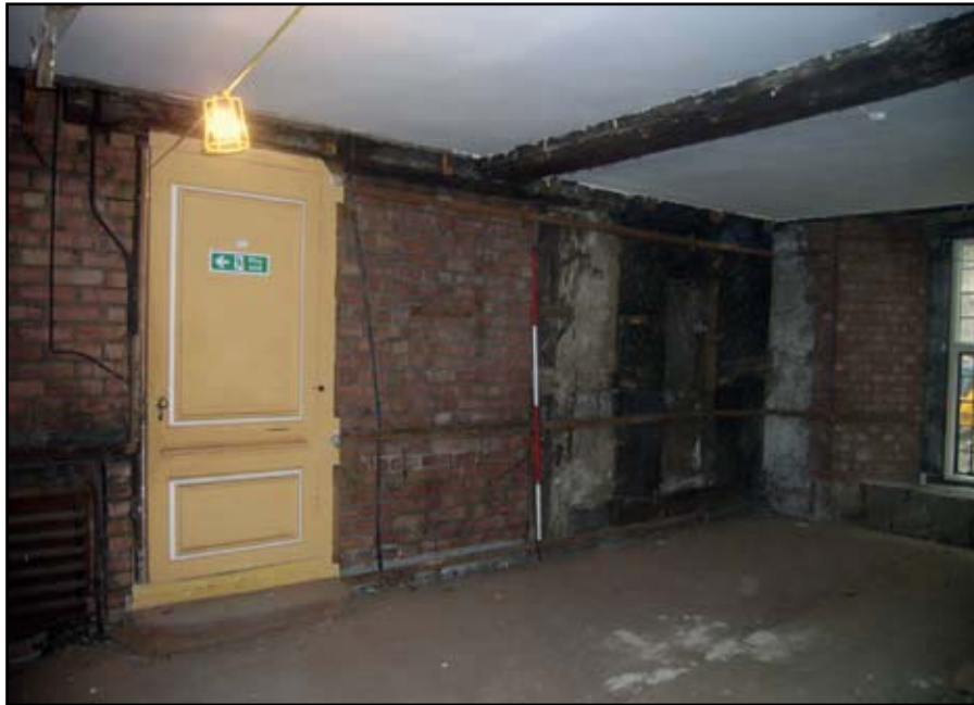
Plate 29: East elevation of Eckersley room
