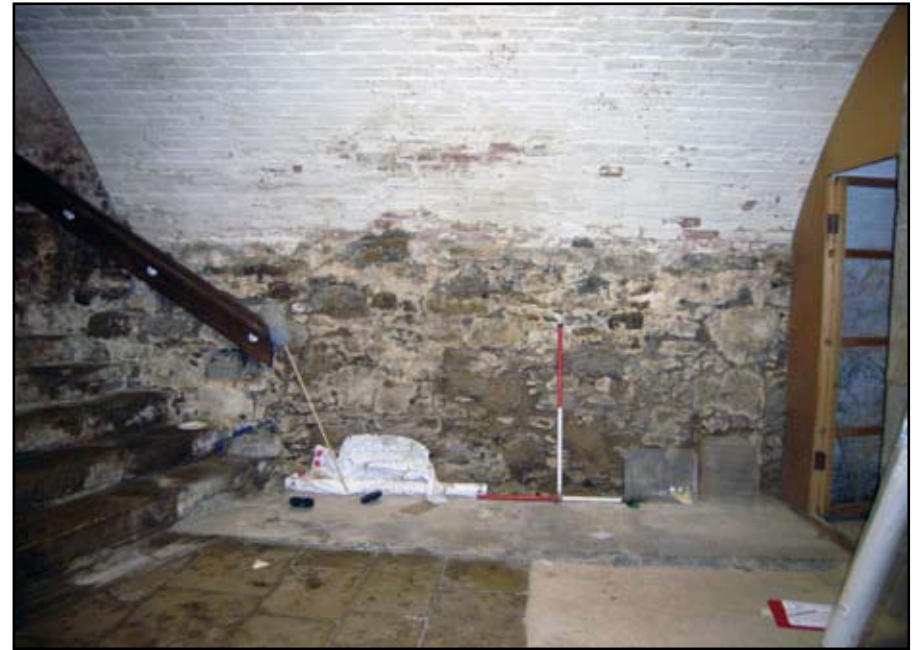
Plate 14: Detail of north wall Buttery Cellar
