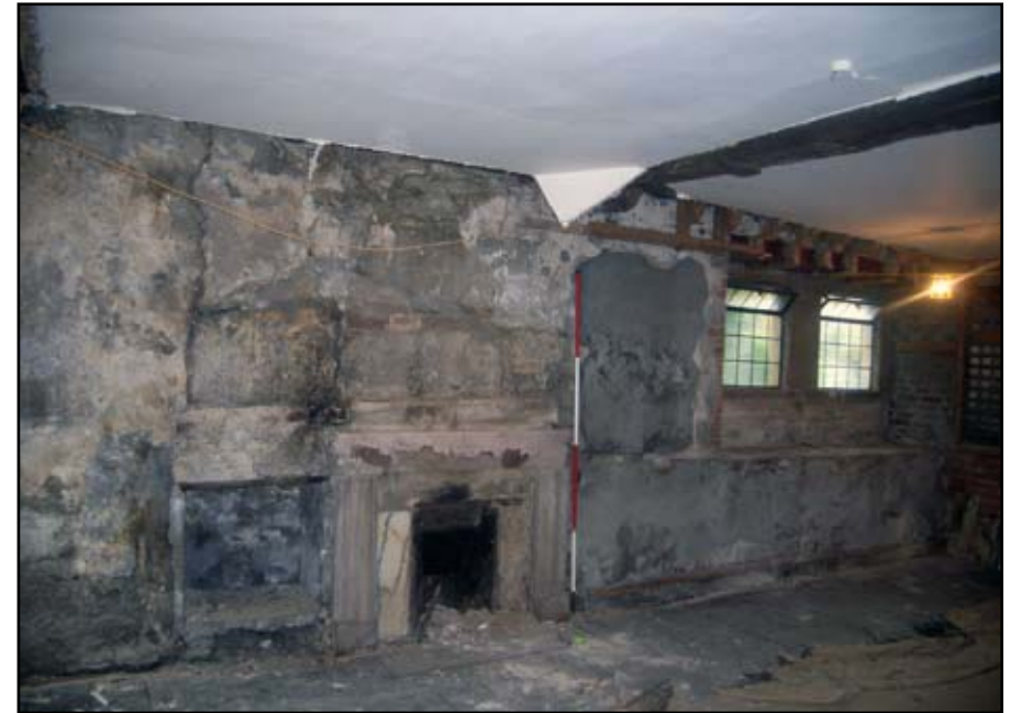
Plate 30: West elevation of Eckersley room
