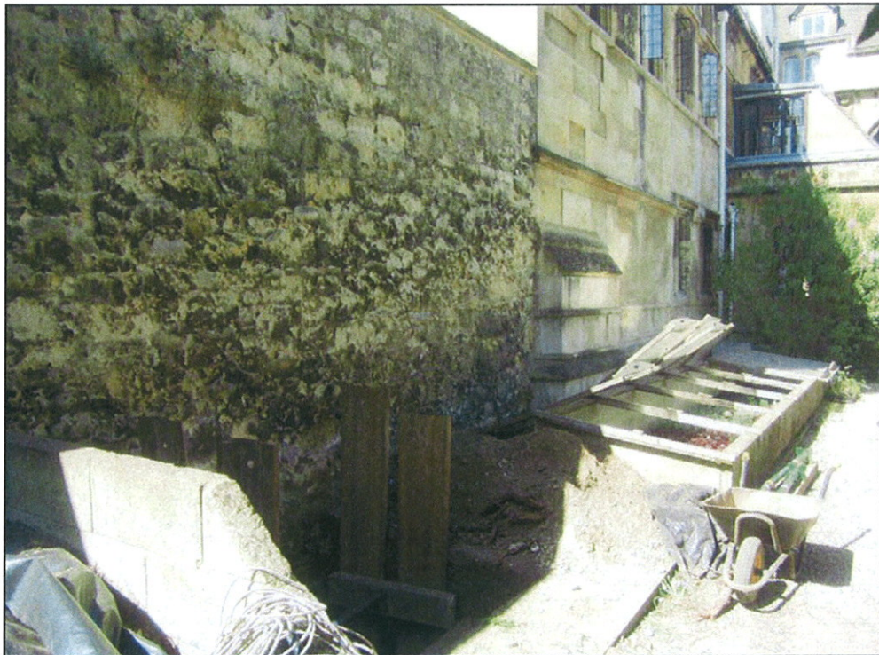
Plate 4: ATP3 General View
