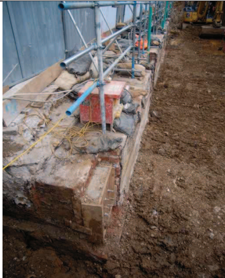
Corner of Macmillan House Basement
