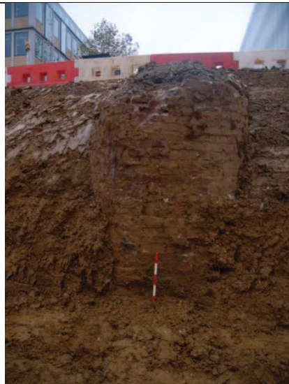
Brick built circular manhole (6553) into Egg Sewer during demolition
