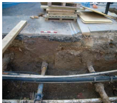
Utilities Trench 1 – Section opposite Cleveland Terrace
