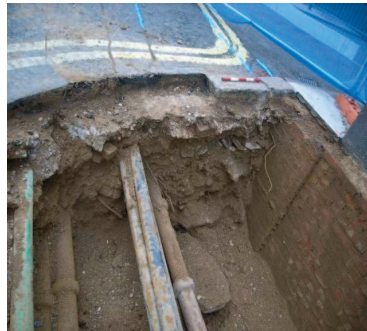
West facing section at east end of trench. Showing pre-existing services and modern brick built retaining wall on right
