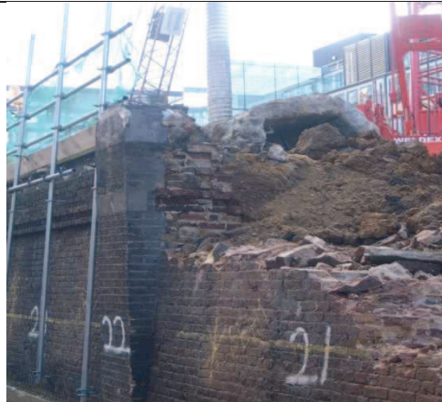
Retaining wall between Eastbourne Terrace and Departures Road during demolition
