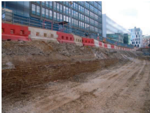
Side of brick built Sewer (6133) looking northwest
