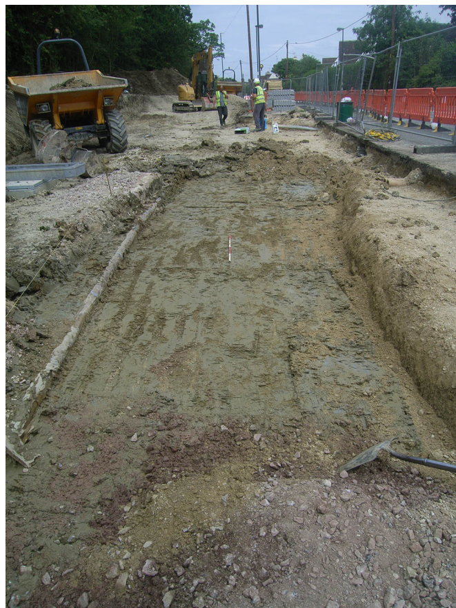
Plate 6: General view of ground reduction
