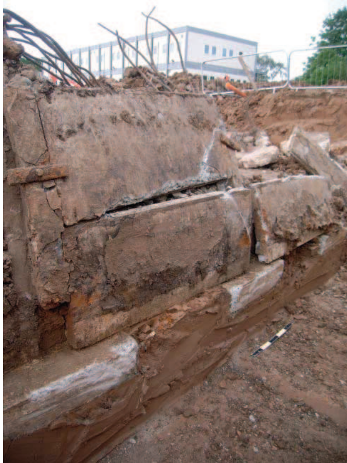
Plate 49: Detail of northern wall of Air Raid Shelter
