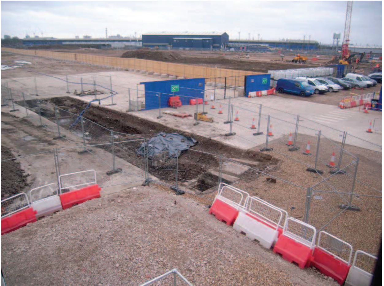
Plate 29: Trench 12. Overall view of trench from NW
