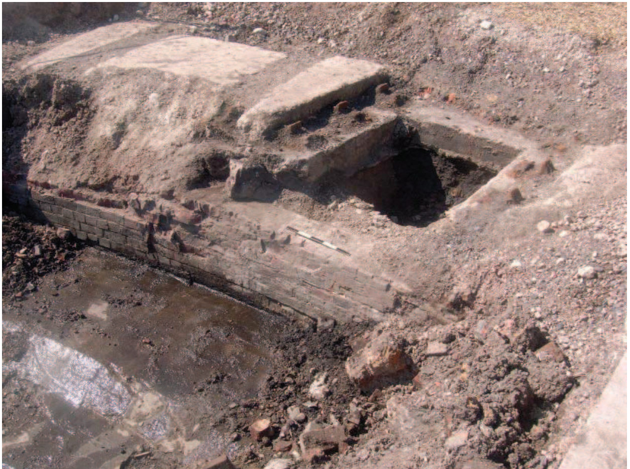
Plate 42: Trench 12. W sidewall [1235] and floor [1223] of turntable
