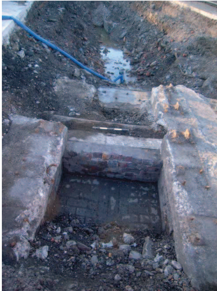
Plate 39: Trench 12. Inspection pit [1243]. Looking W. Showing W end of pit, floor [1216] and step [1222]
