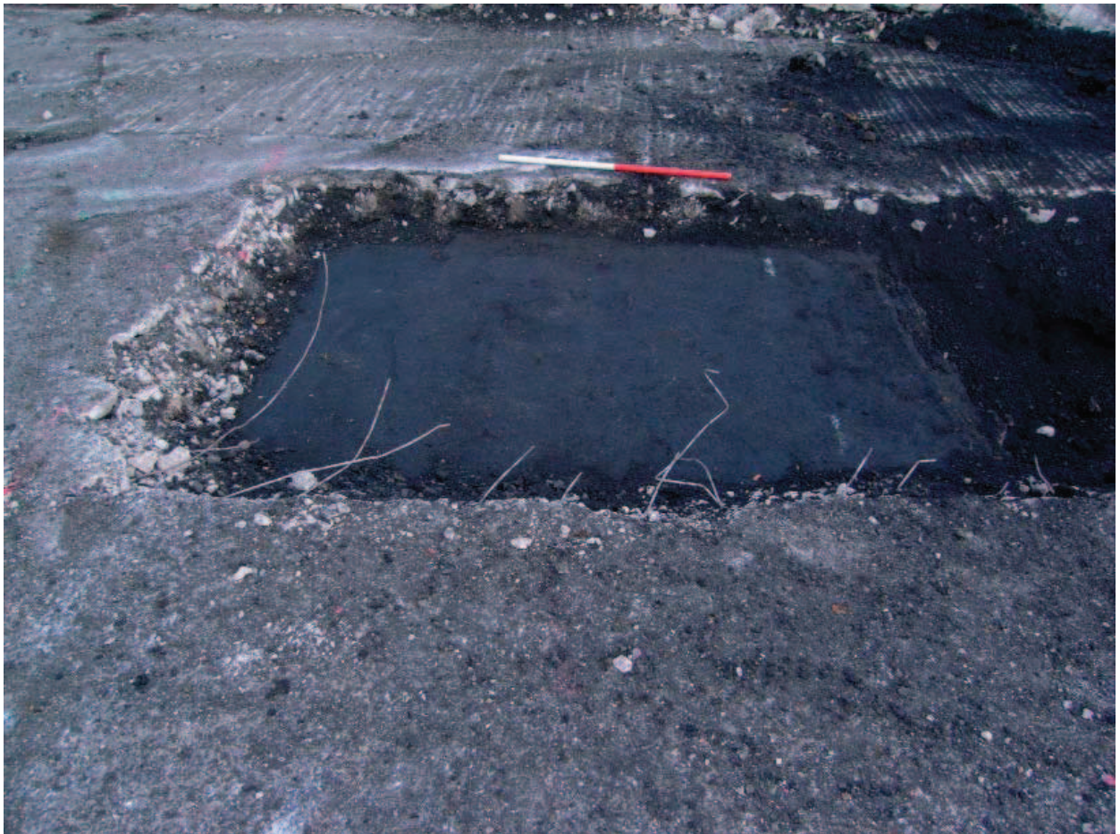
Plate 4: Trench 2. Looking north. Former concrete roadway (203)
