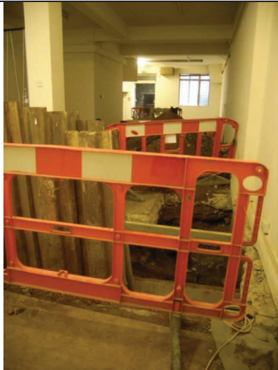
Interior view of 21 Noel Street basement. Looking north
