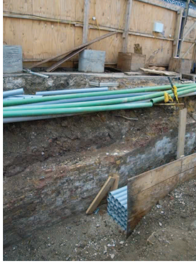
Great Chapel Street, wall
