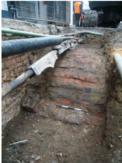
Cellar 5495, looking west
