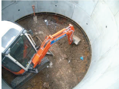
Grout Shaft 1, barrel vaulted sewer
