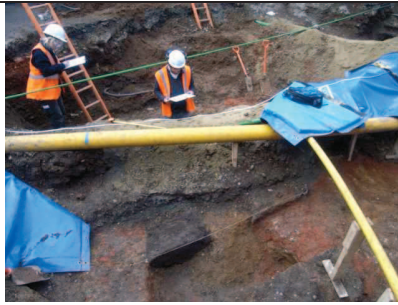
Working Shot of Grout Shaft 5 excavations, looking W
