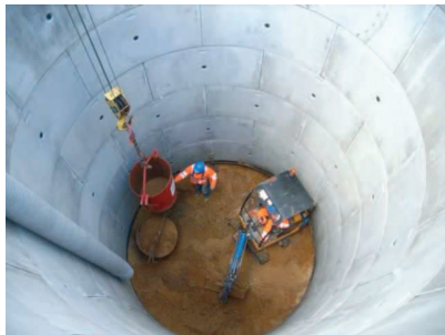
Grout Shaft 1, natural gravels 5501
