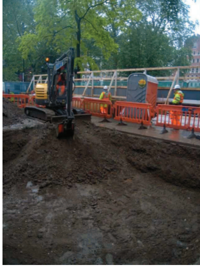
Grout Shaft 2, ready for bulk excavation, looking SE
