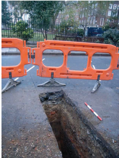
Trench 1, looking S
