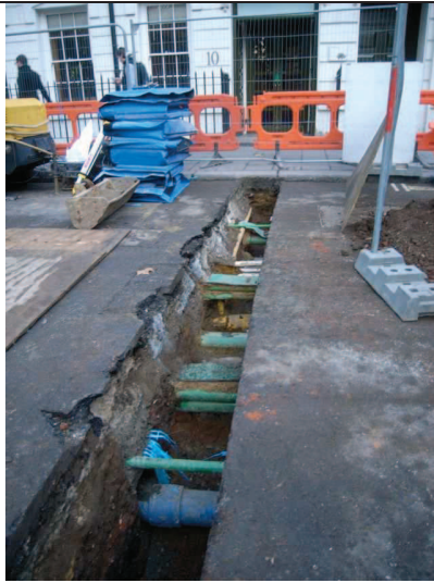
Trench 1, looking N
