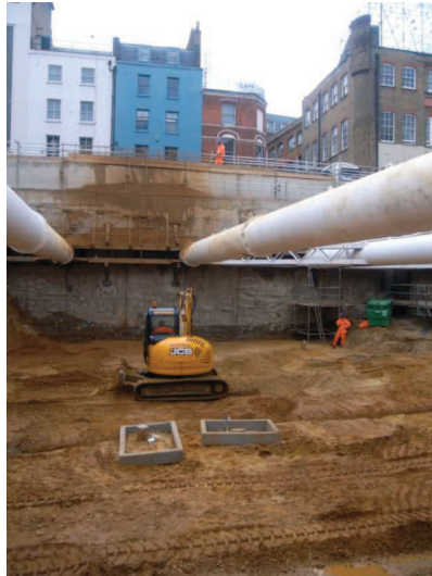
General view of bulk dig, looking west
