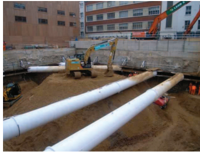
General view of bulk dig, looking SW
