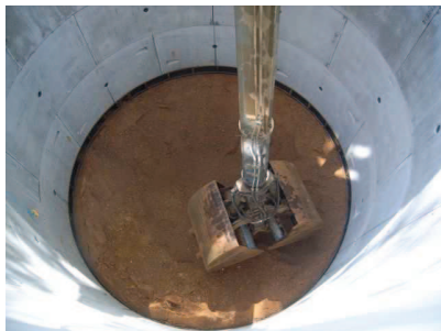
Grout Shaft 2, natural deposits, mid depth
