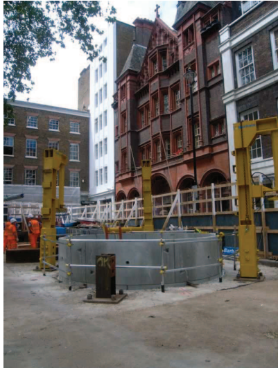
Grout Shaft 2, general view, looking NW
