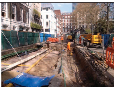
Grout Shaft 2 working shot, looking E
