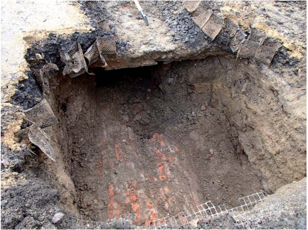
Plate 3: Showing state of condition of culvert
