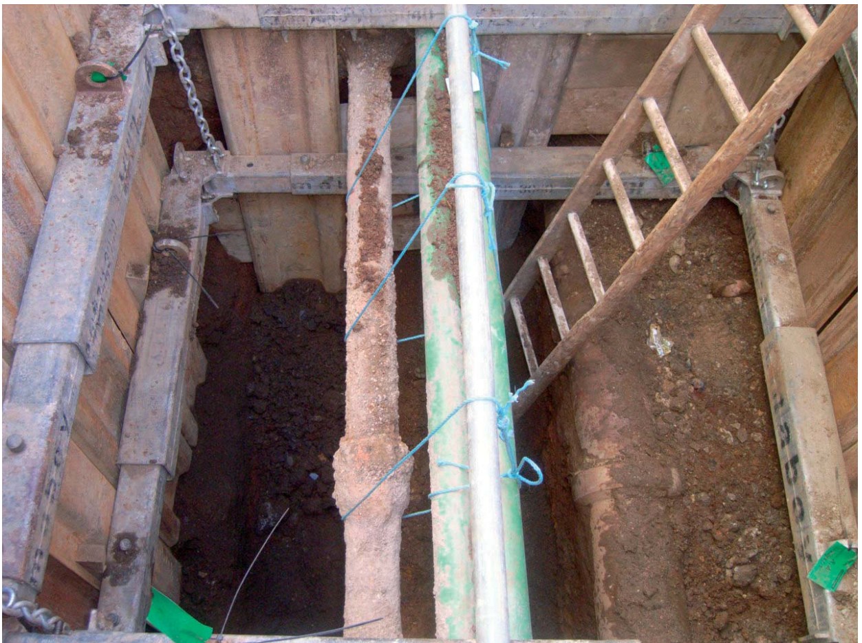
Plate 2. Excavation area, services and access step, looking north
