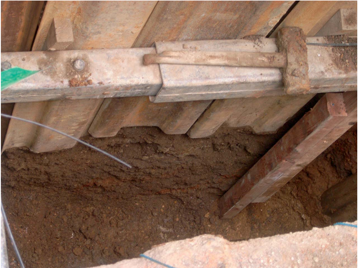
Plate 5. Darker deposits seen on west side of excavation
