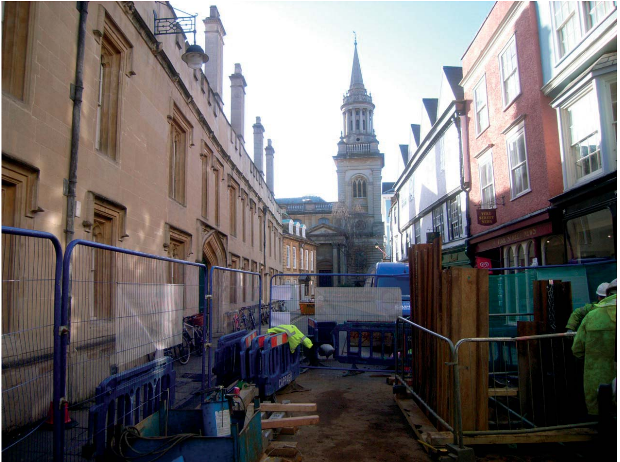
Plate 1. Location of excavation in Turl Street, looking south
