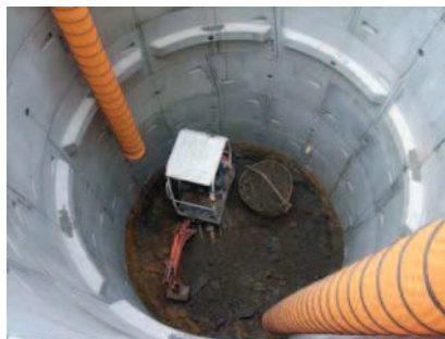
Grout Shaft 3, natural gravels and clay at base
