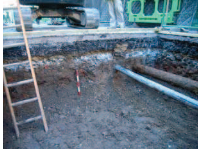
Sewer diversion, upper layers, looking west
