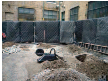
General view of test pits, looking east
