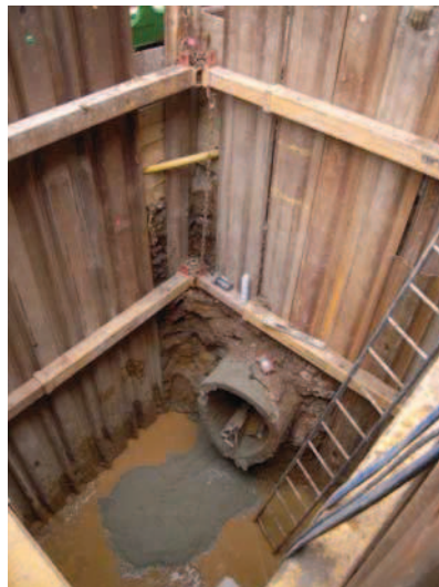
Sewer truncated as part of diversion, looking east
