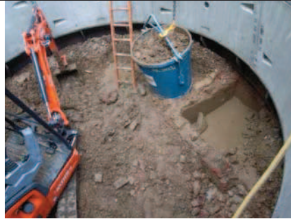
Grout Shaft 4, exposed manhole
