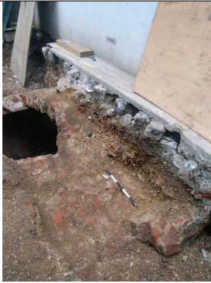
Adjacent brick vaults, looking NE
