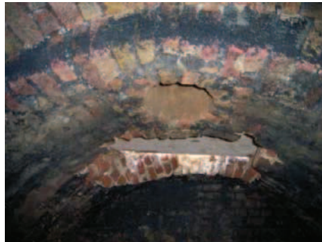
Aperture in 4036 roof, looking east
