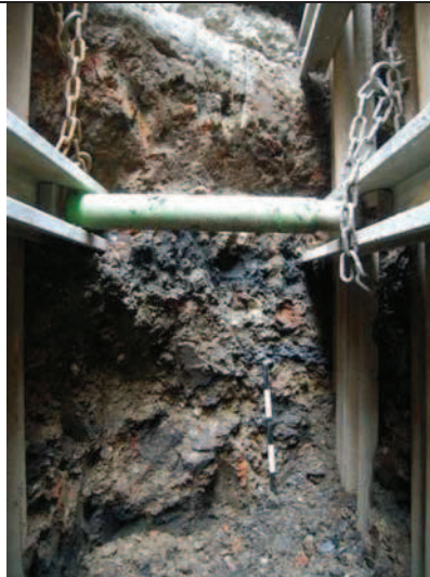
Water and sewer diversion trench, top 1.5m of deposits, looking south-east
