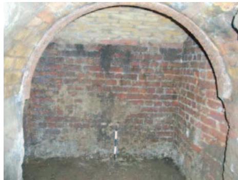
Vault 4036 interior, looking east
