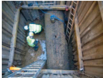
Sewer in situ, looking east
