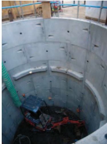
Grout Shaft4, natural clay at the base
