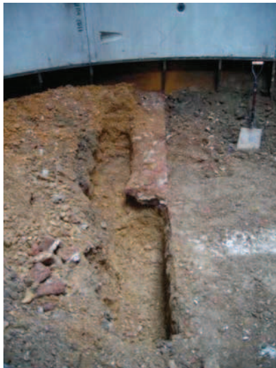
Grout Shaft 3, lower brick structure
