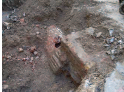
4769 and manhole 4770 from south west
