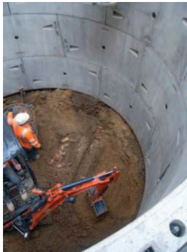
Grout Shaft4, partial excavation
