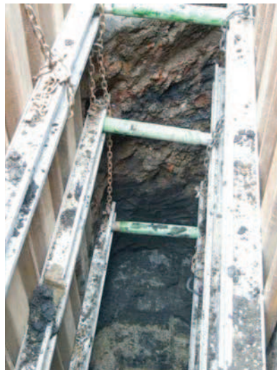
Water and sewer diversion trench, bottom 1m of deposits, looking south-east
