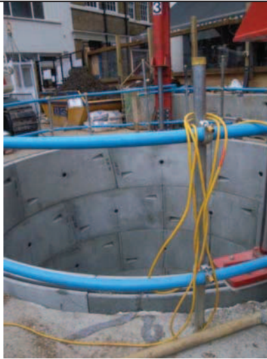
Grout Shaft 3, location view, looking west
