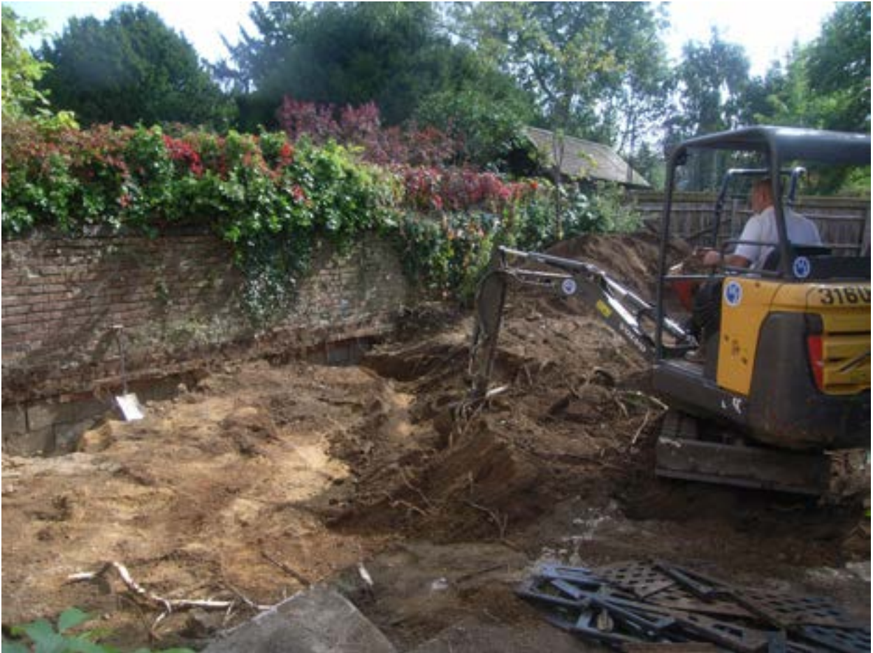
Plate 1: 0011 Topsoil stripping underway
