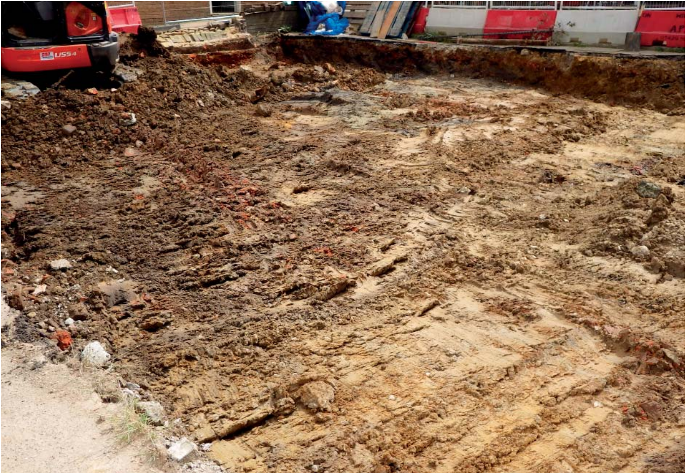
Plate 1: General site area
