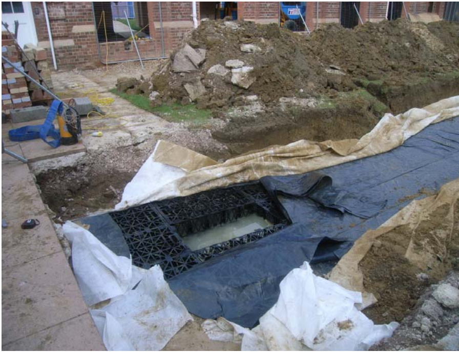
Plate 1: NW view of courtyard. Exposed soakaway crates.
