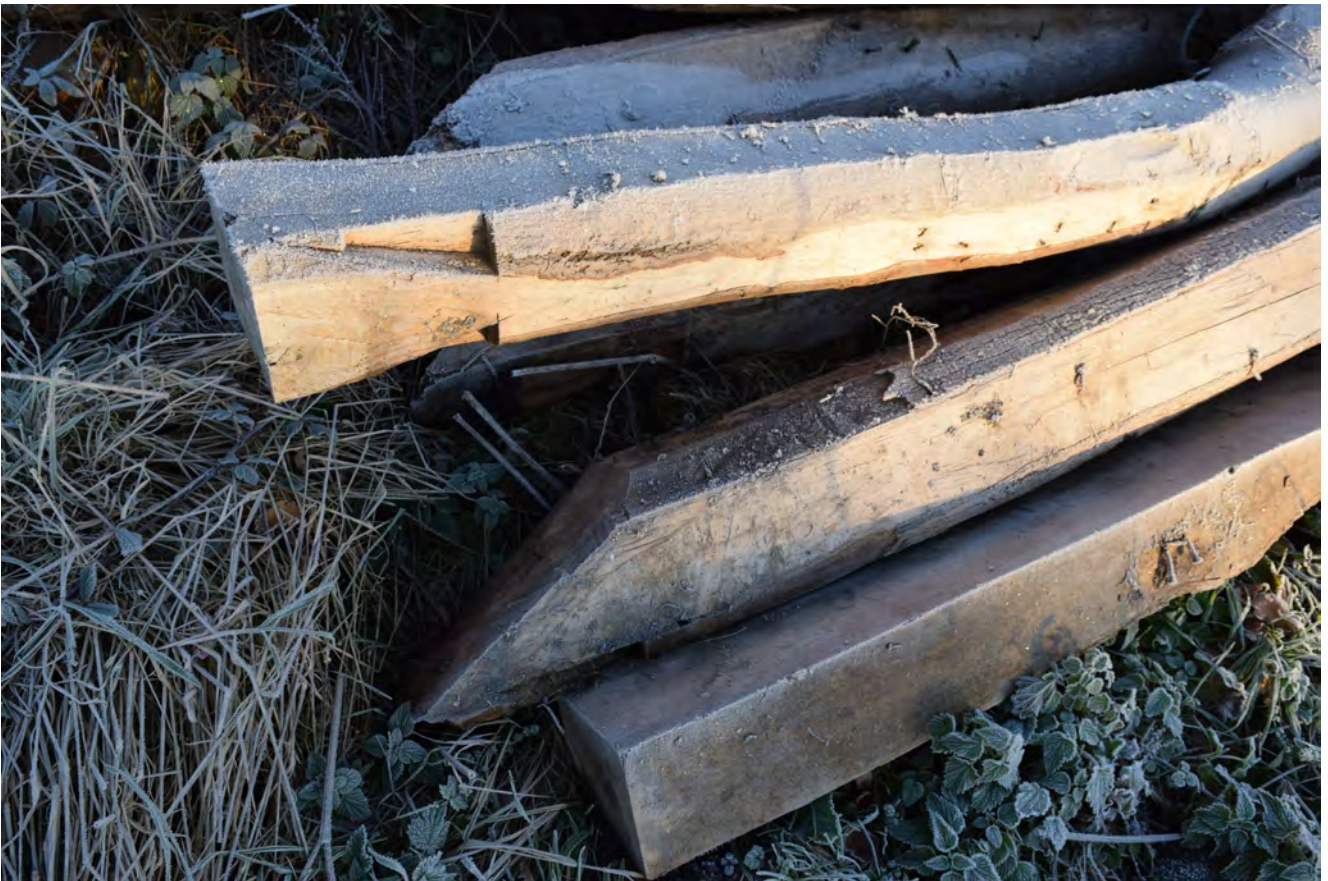
Plate 20: Example of the lap dovetail joints in the beams
