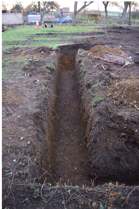
Plate 33: A typical featureless foundation trench cut well into the natural. Looking west
