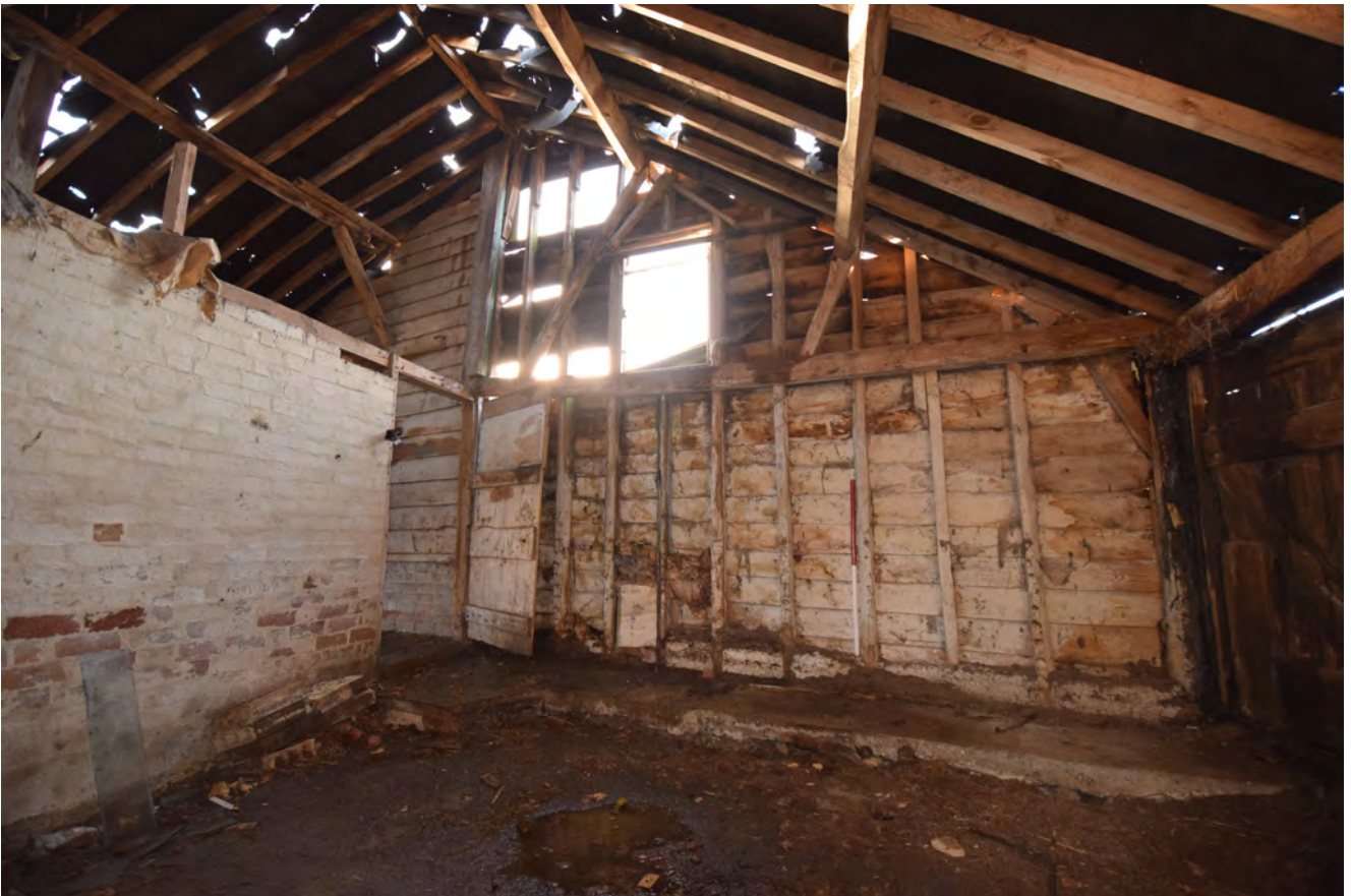
Plate 16: The wall frame of the west end of the barn
