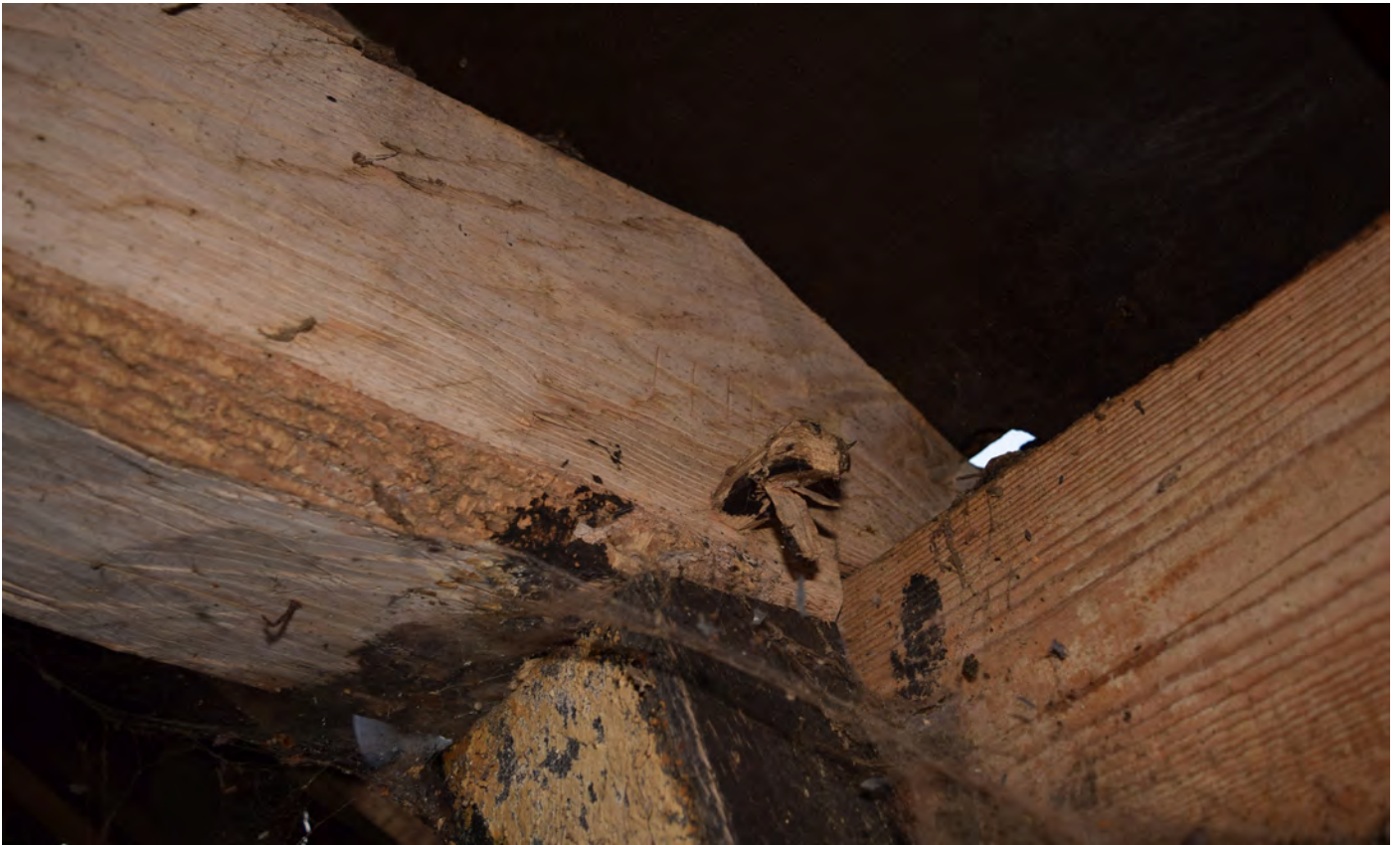
Plate 21: A carpenter's mark which does not appear in the adjacent timbers
