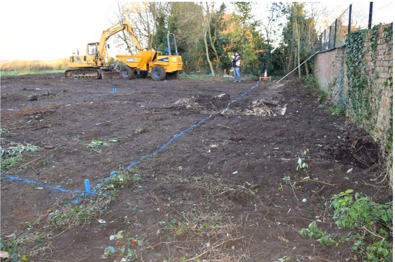
Plate 29: The stripped area and the concrete path and base. Looking north
