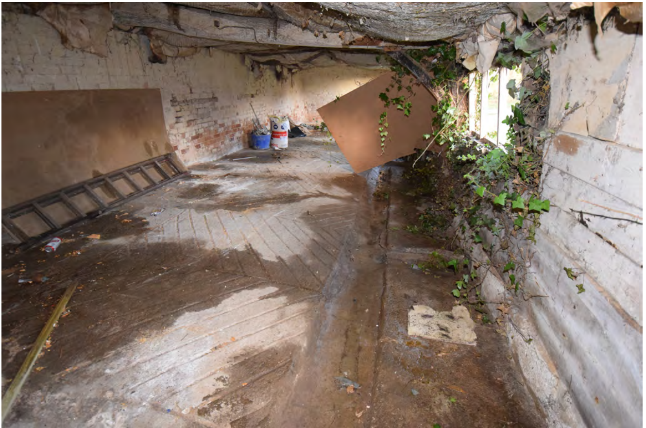
Plate 22: The modern concrete floor in the south half of the barn. Looking east
