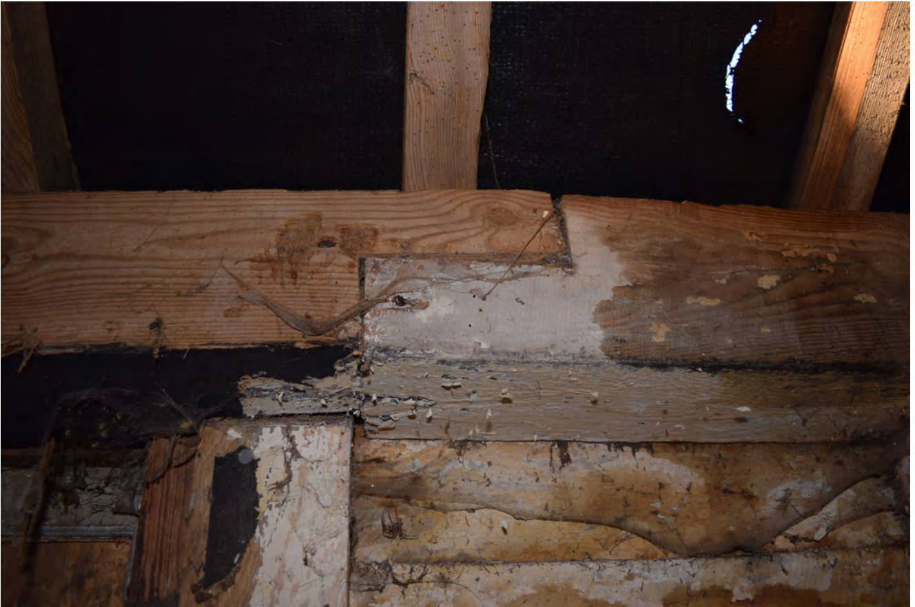
Plate 19: Example of the rough scarfing of the wall plate
