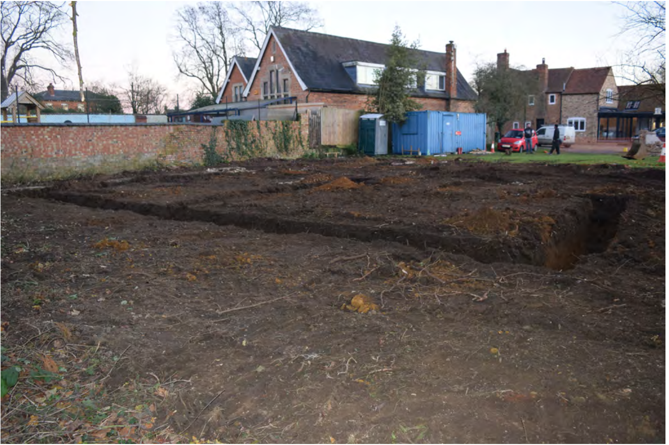
Plate 34: The site following excavation, prior to concrete pouring. Looking south east
