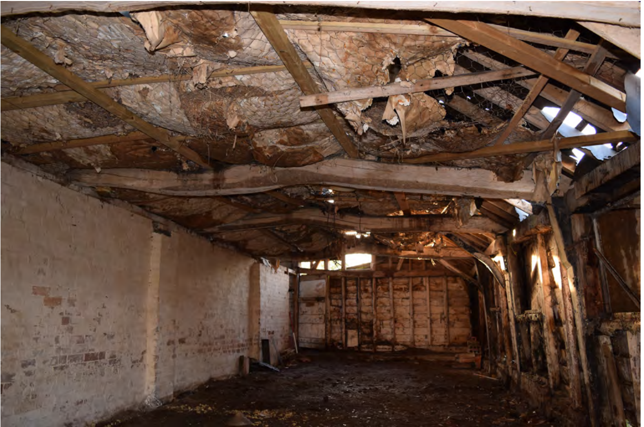
Plate 17: The north half of the barn including the waney, irregular tie beams. Looking west
