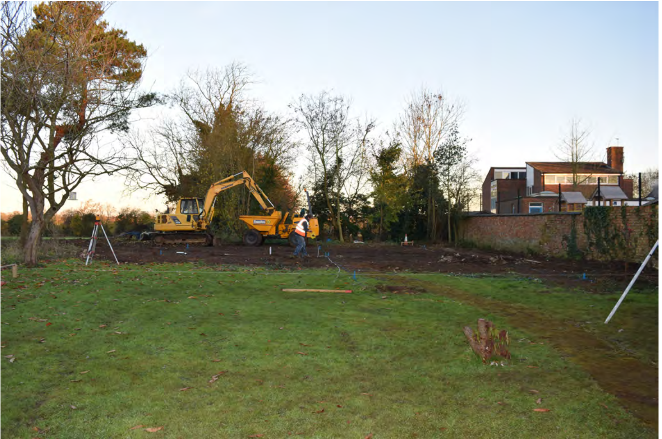
Plate 28: The site of the new building prior to stripping. Looking north
