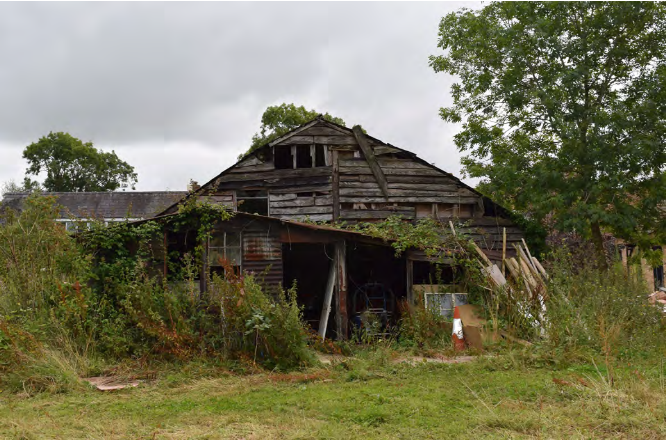
Plate 9: The west elevation of the barn
