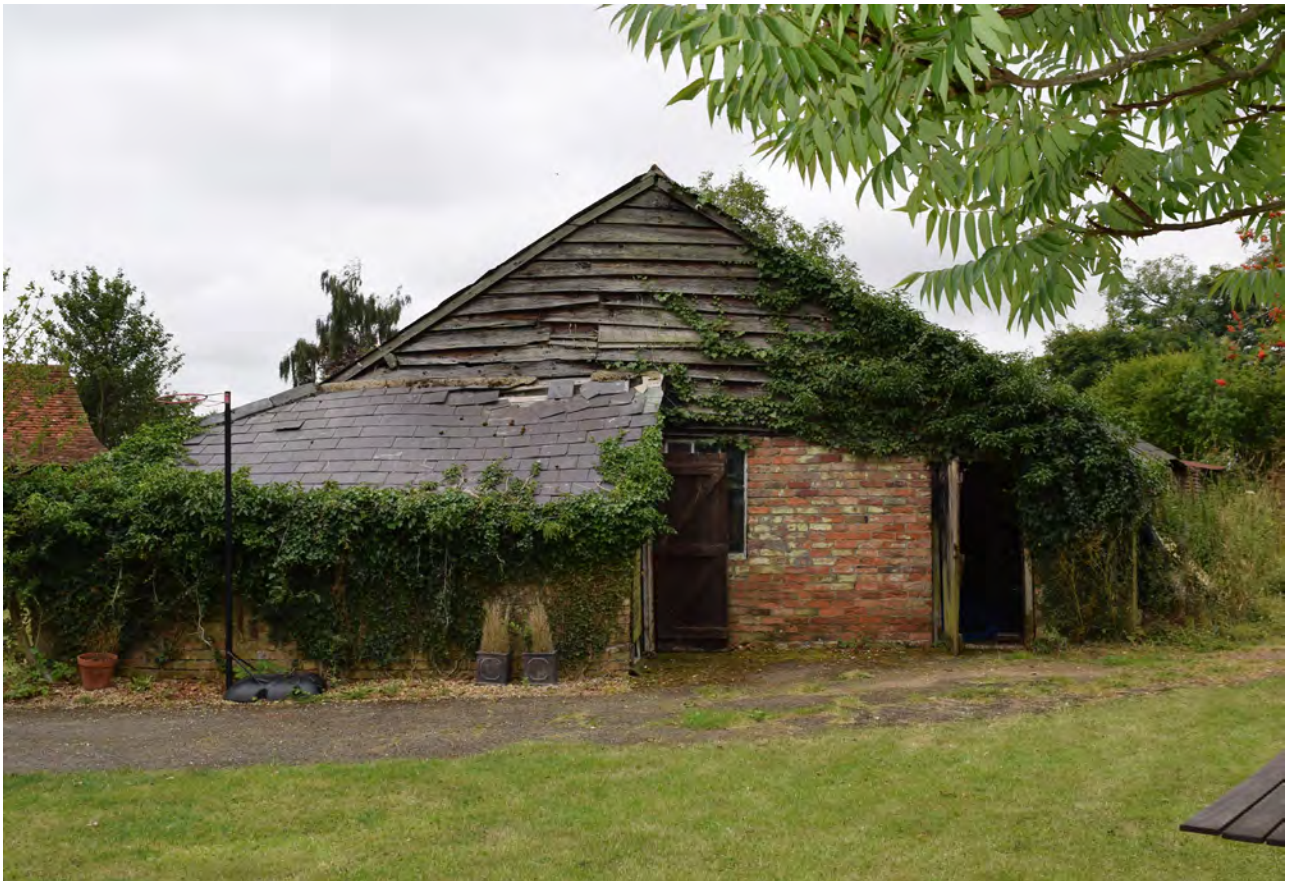
Plate 8: The east elevation of the barn
