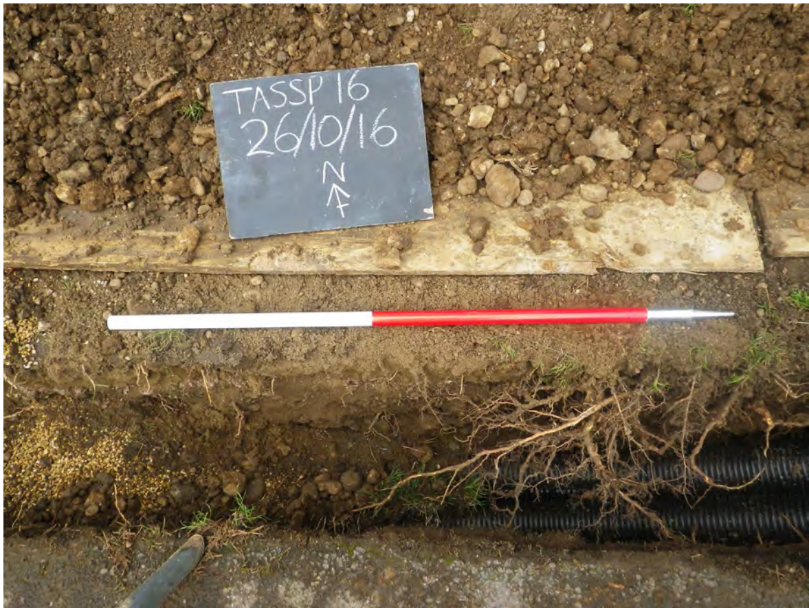
Plate 30: Southern end of avenue trench
