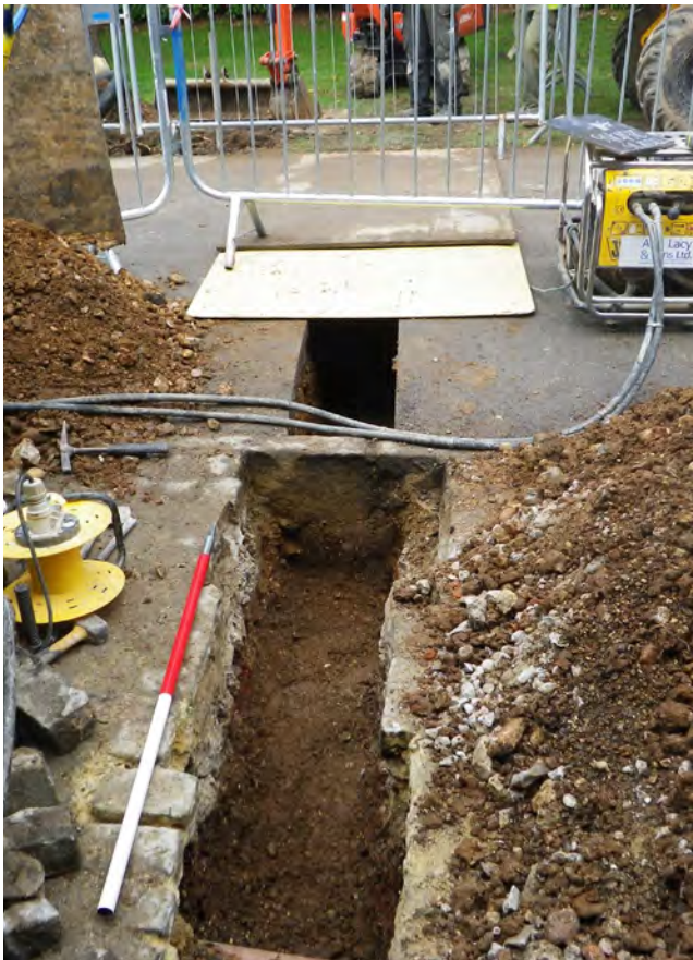
Plate 33: Trench to north of kitchen where it crosses road, looking north
