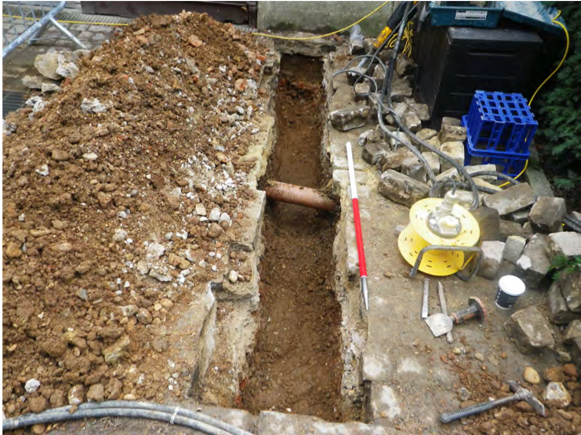
Plate 32: Trench in cobbled area immediately north of kitchen, looking south
