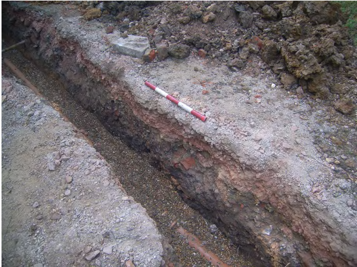
Plate 4: Southernmost section of trench in overflow car park, looking south
