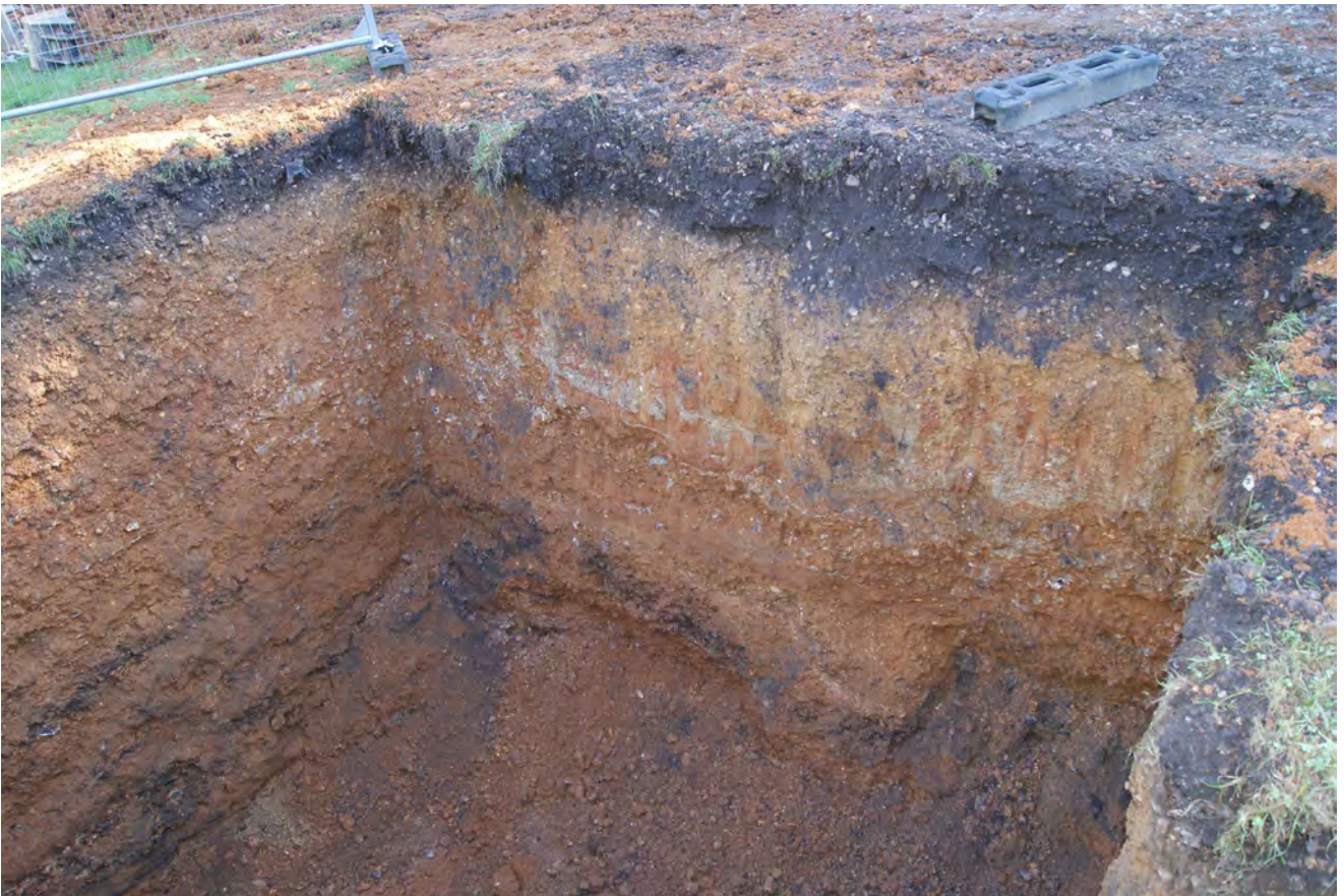
Plate 18: East face of soakaway
