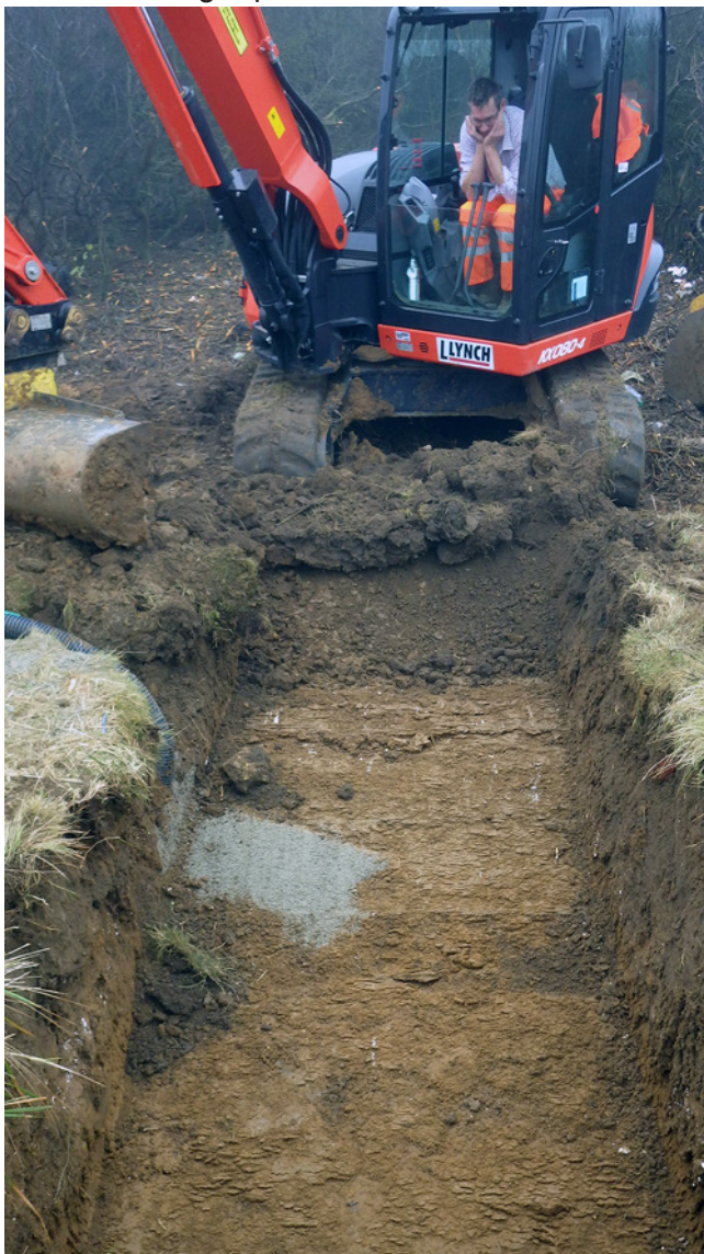
Plate 2: Trench A working shot
