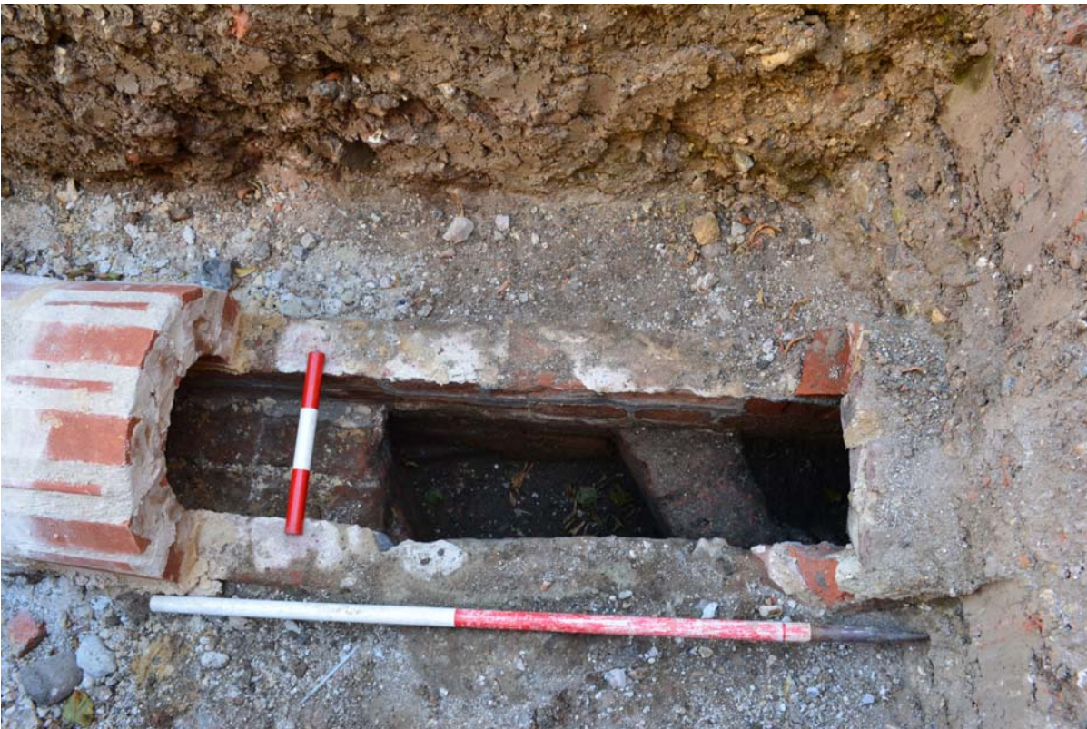
Plate 8: Repaired culvert sections with signs of early drainage at the base
