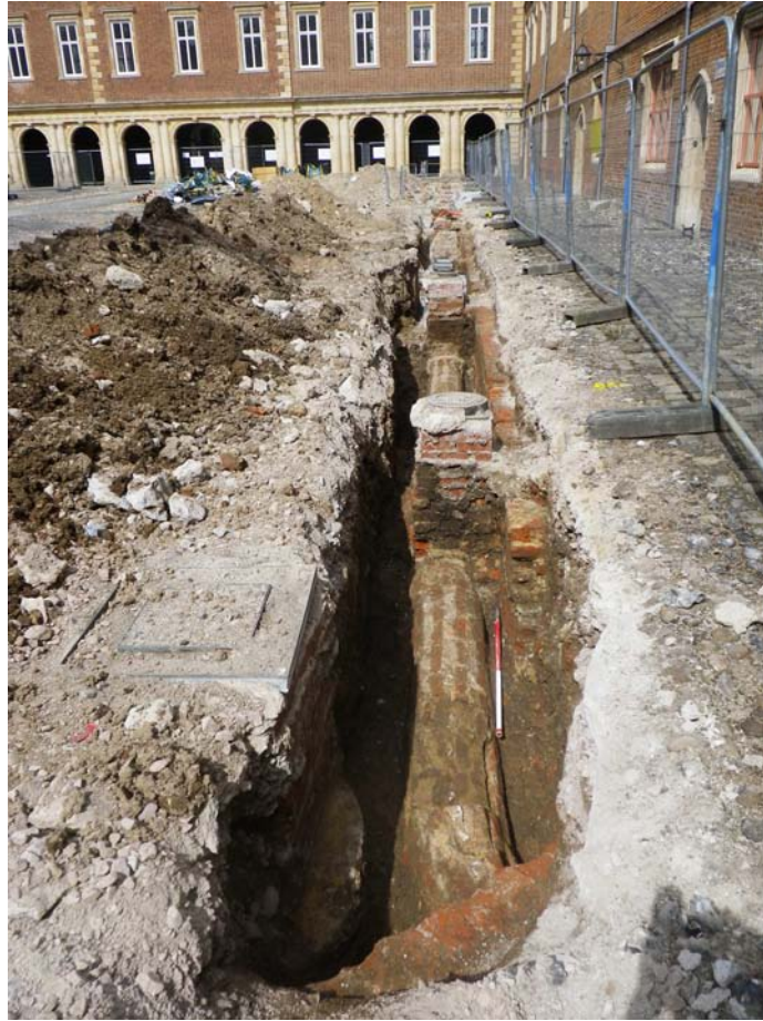
Plate 5: Excavations of the main drainage culvert (looking west)
