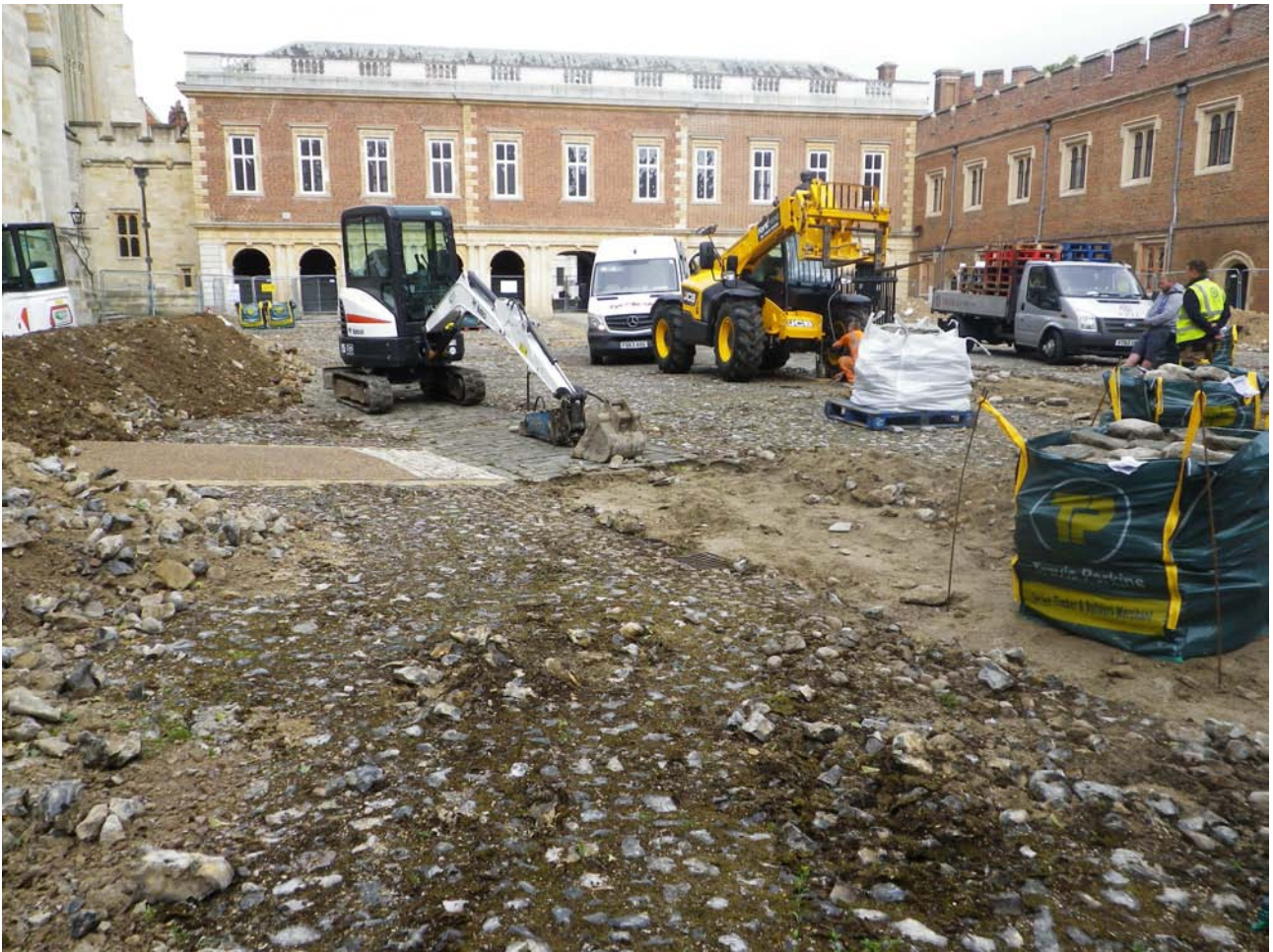
Plate 3: Monitoring of the removal of the existing cobbled surfaces (looking northwest)
