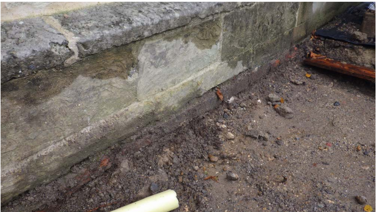
Plate 10: Revealed foundations of the College Chapel
