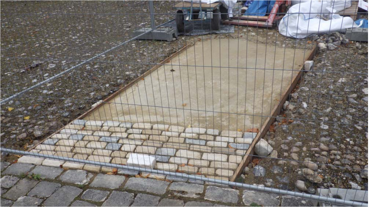
Plate 5: Insertion of one of the new stone designs in Trial Area B
