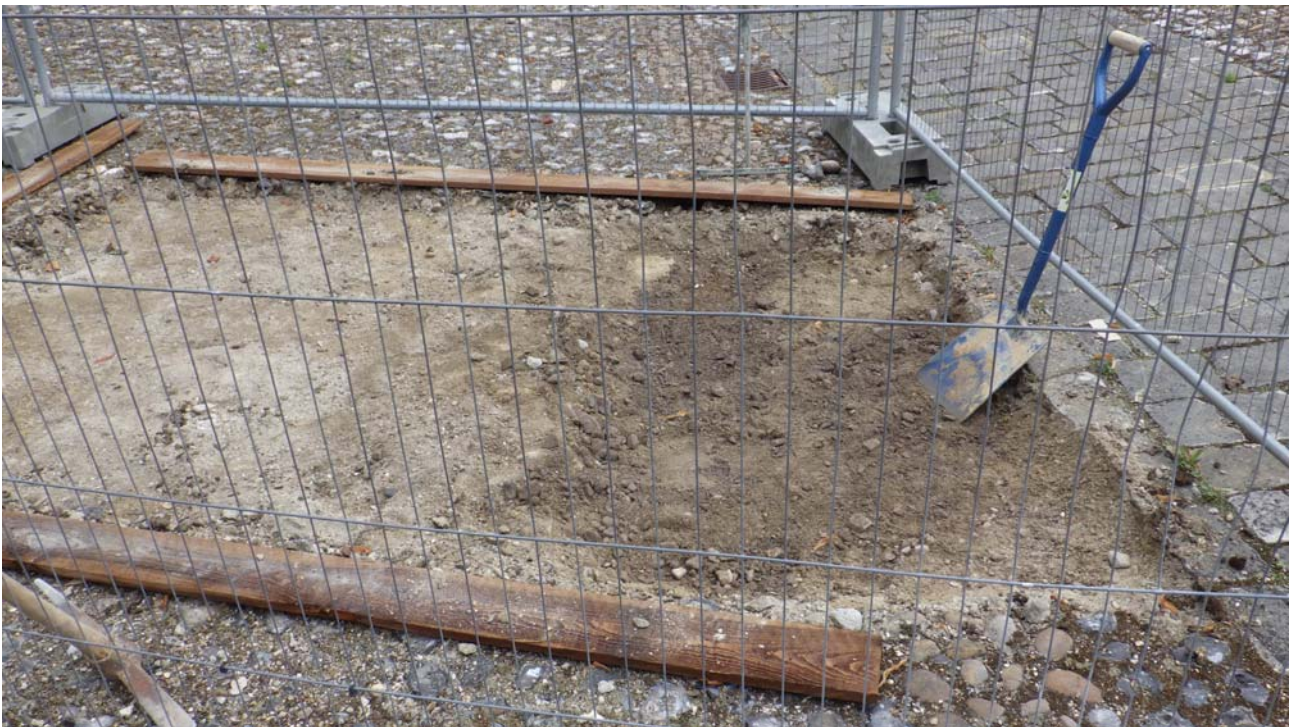
Plate 4: Trial hole with the cobble surface removed in Trial Area B
