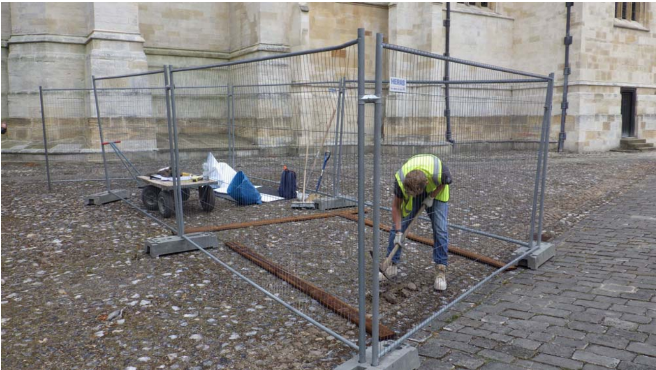
Plate 3: Hand excavation of the cobbles within Trial Area B
