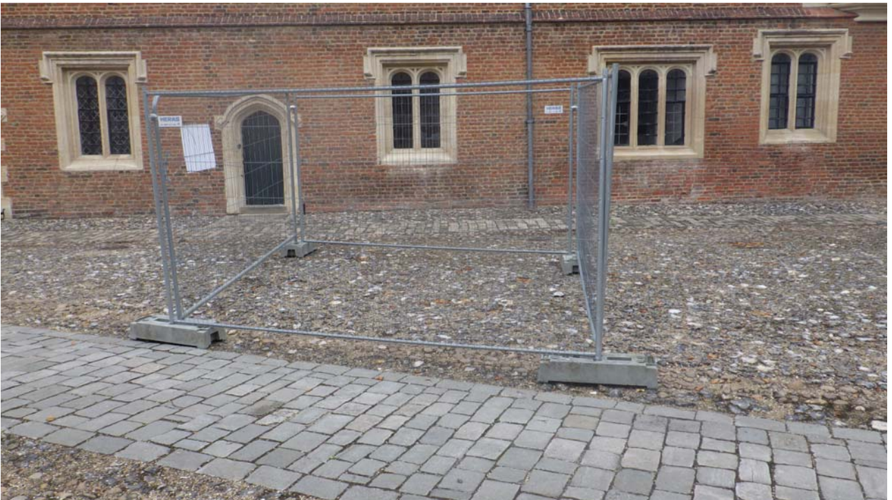
Plate 6: Trial Area A pre-excavation
