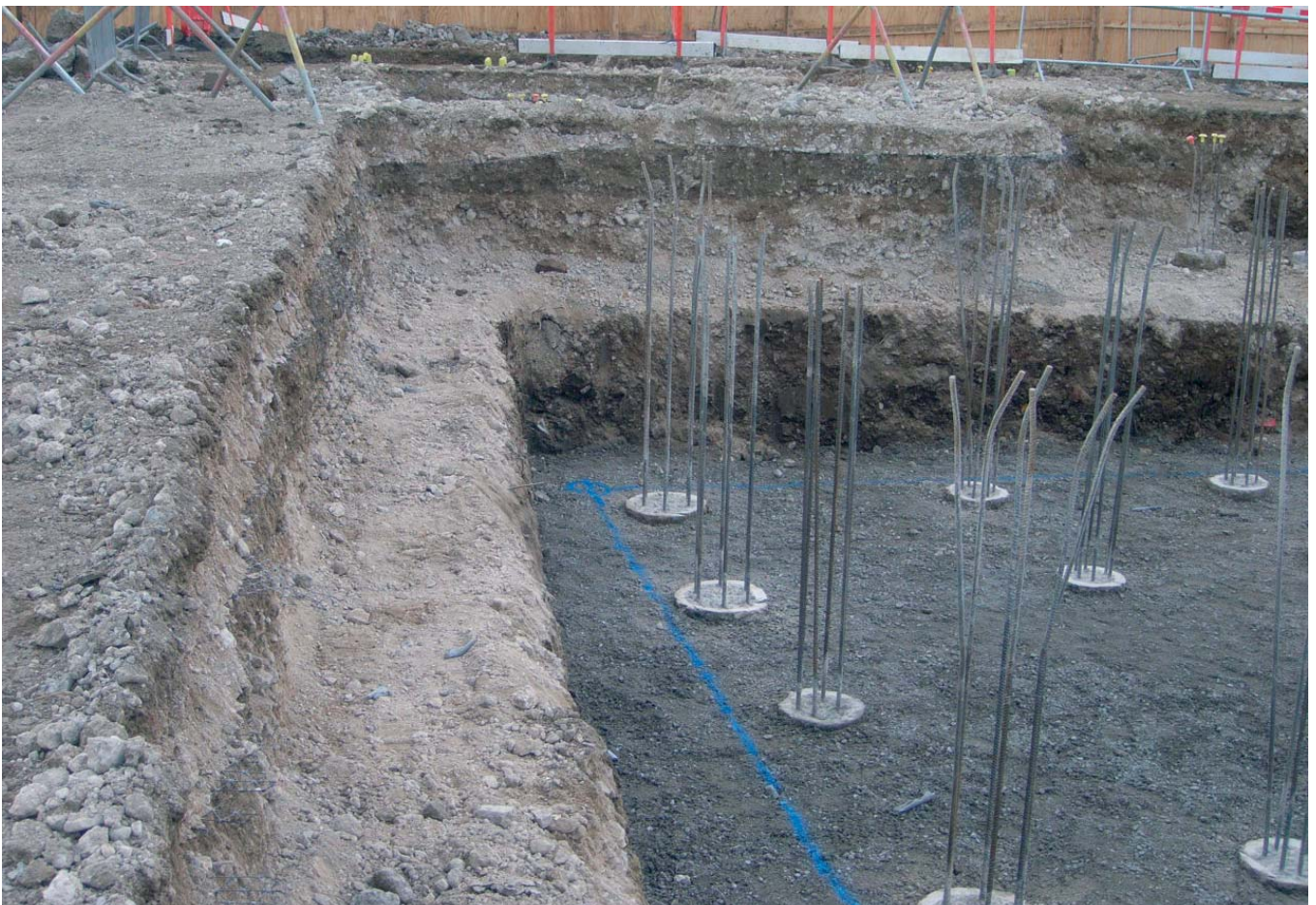
Plate 2: Typical pile cap excavation in NW area of site
