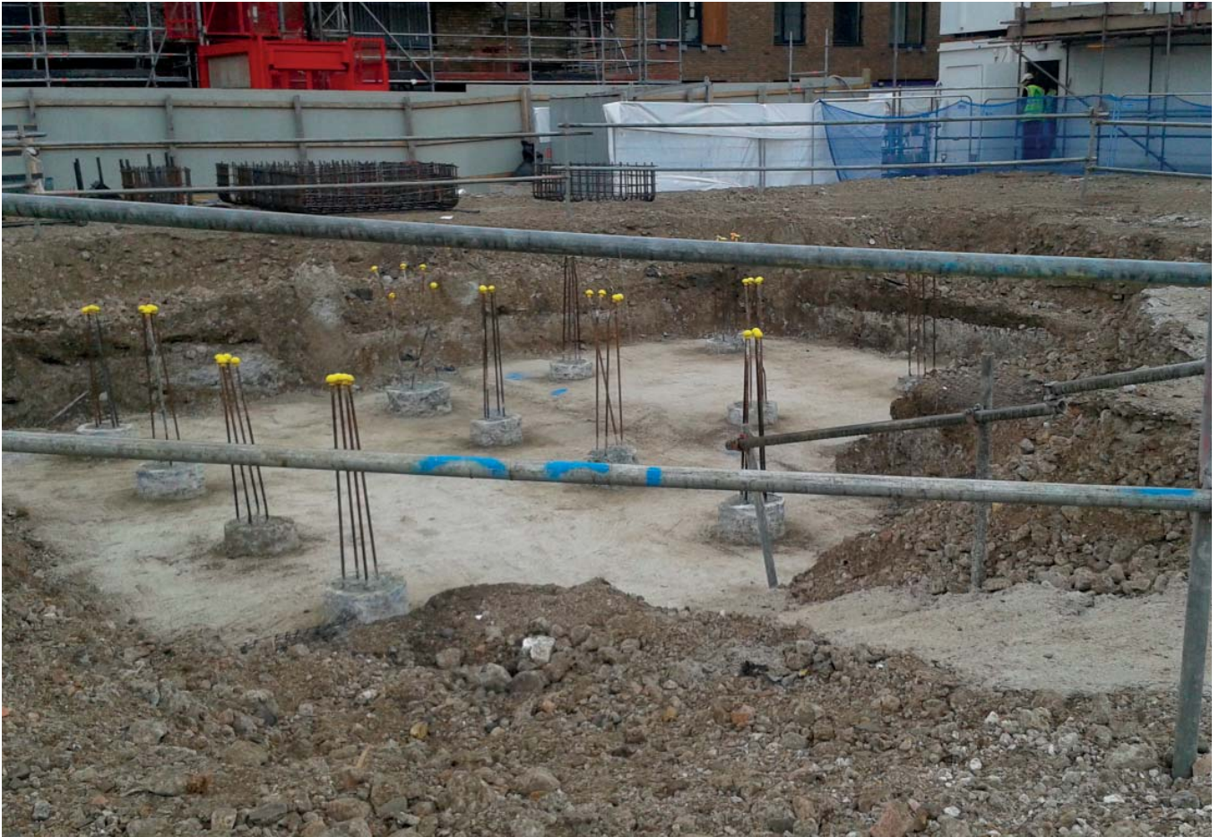
Plate 1: Typical pile cap excavation in NE area of site
