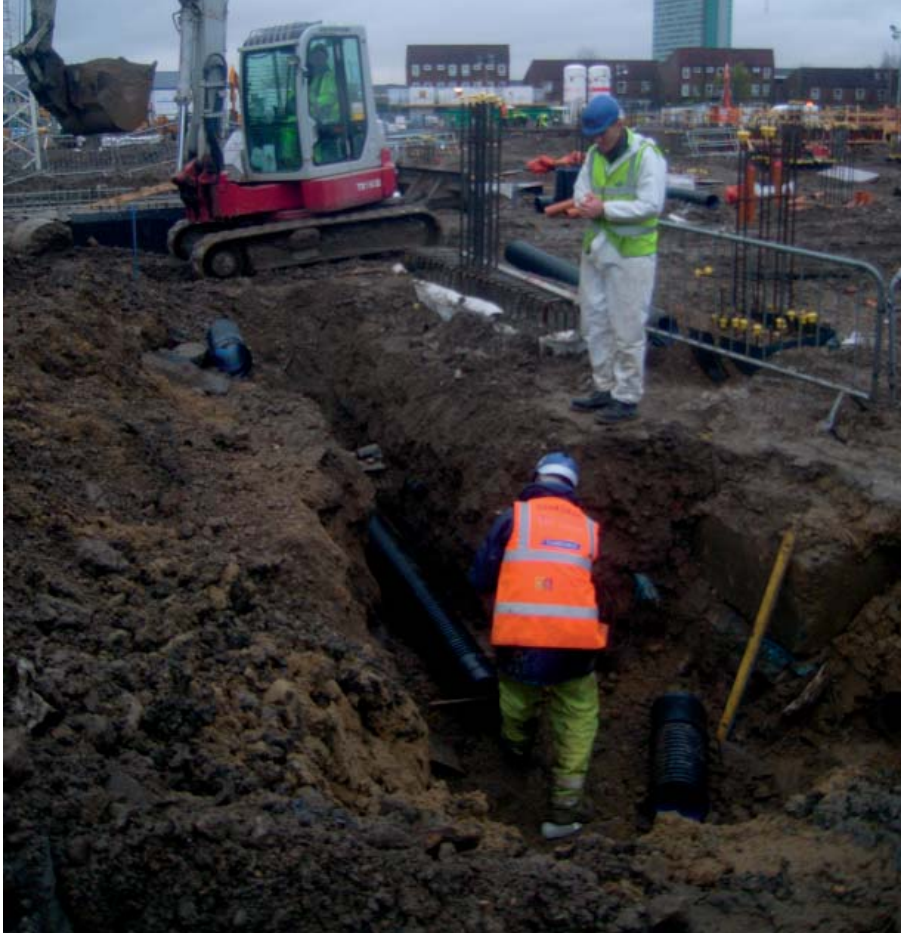
Plate 3: Service trench excavation through modern made ground
