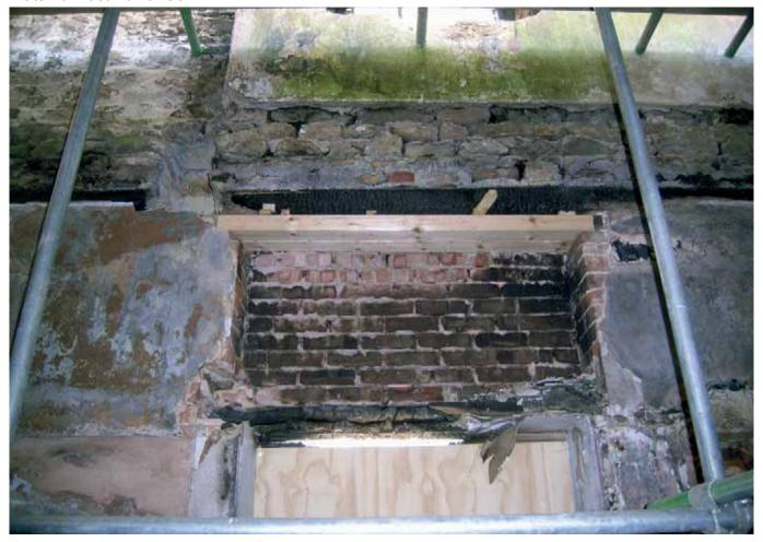
Plate 49: Blockwork above window in G5
