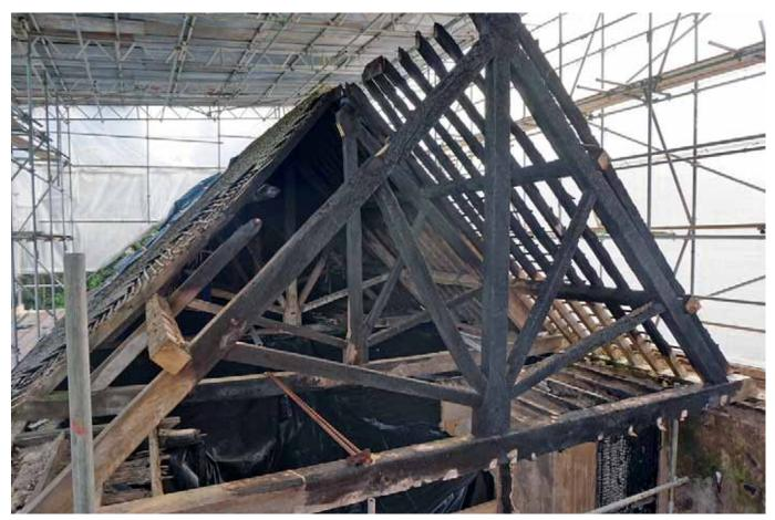
Plate 69: Surviving roof truss to east of F1
