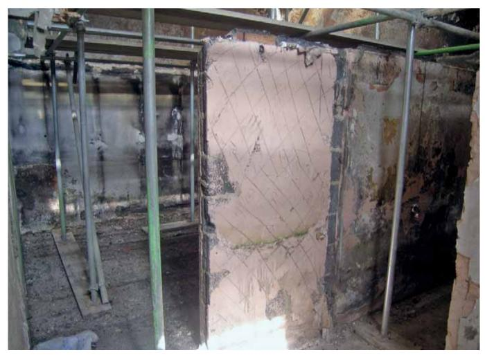
Plate 45: Concrete blockwork forming south wall of G4
