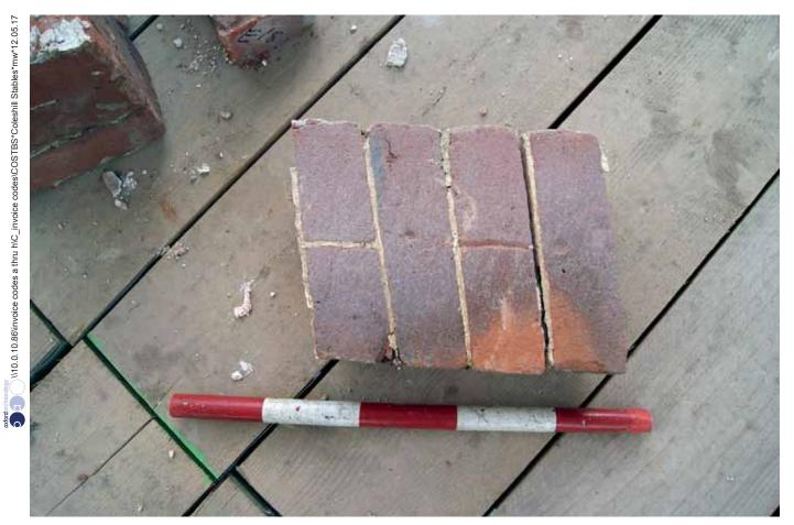
Plate 88: Rubbed bricks from dismantled first floor lintel
