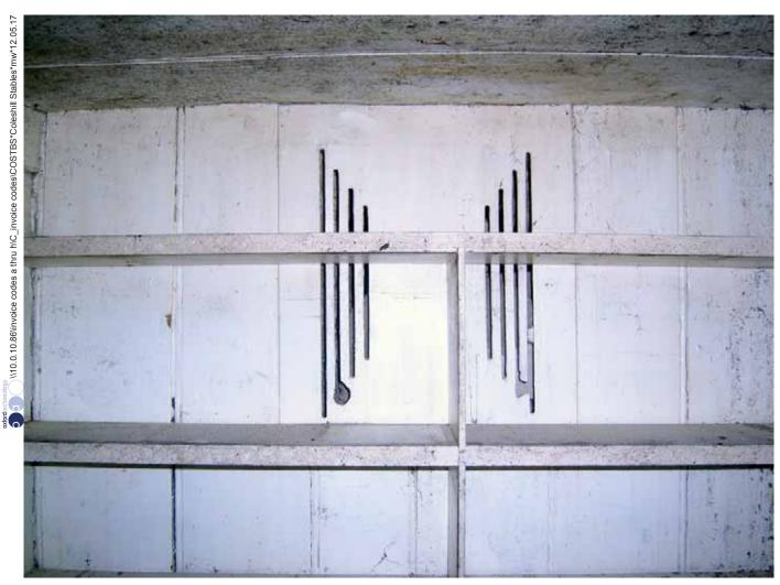
Plate 60: Possible vent in north wall under stairs
