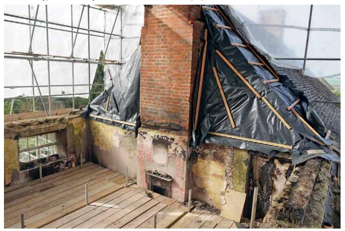
Plate 101: West end of fire damaged area at first floor level (F6)
