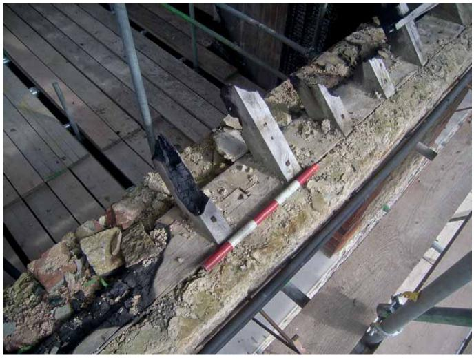
Plate 73: Wall plate with rafter feet in F1
