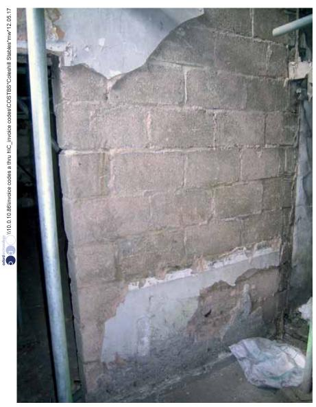
Plate 46: Concrete blockwork forming west wall of G4
