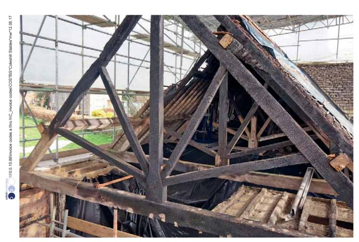
Plate 70: Surviving roof truss to east of F1
