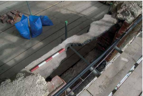
Plate 91: Fire damaged timber lintel in F4
