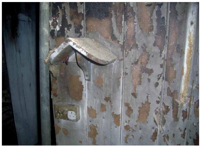
Plate 26: Saddle bracket in former Harness Room (G1)
