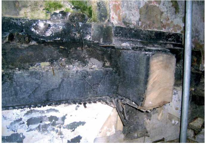
Plate 65: Truncated principal joist in north wall of G7
