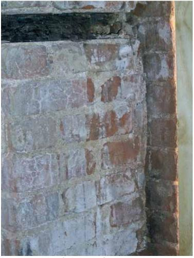
Plate 38: Jambs of window in G3 showing brick courses not aligning
