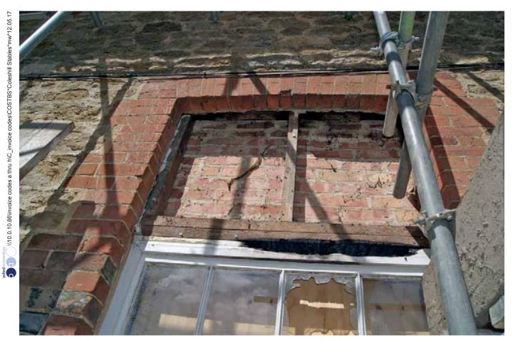
Plate 11: Window to G5 with infilled upper section due to lower inserted ceiling
