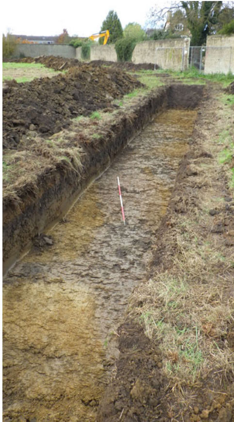
Plate 11: Trench 10: plan view, looking north
