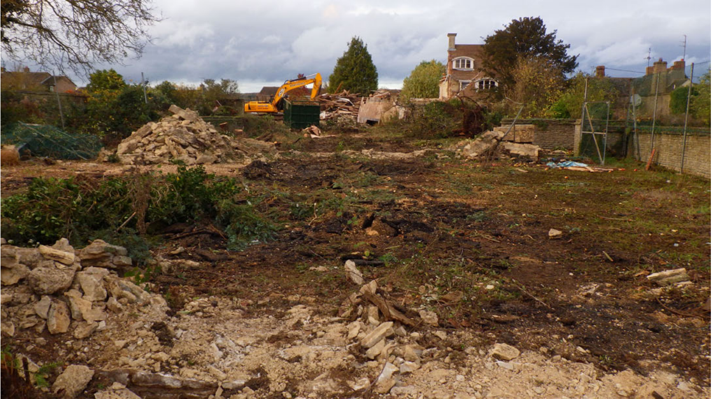
Plate 14: Area B: general view, looking north
