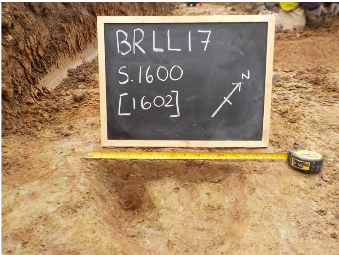
Plate 17: Section of posthole 1602 facing north-west
