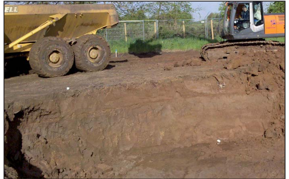
Plate 16: West Field, stone drain 1045 in section, looking west
