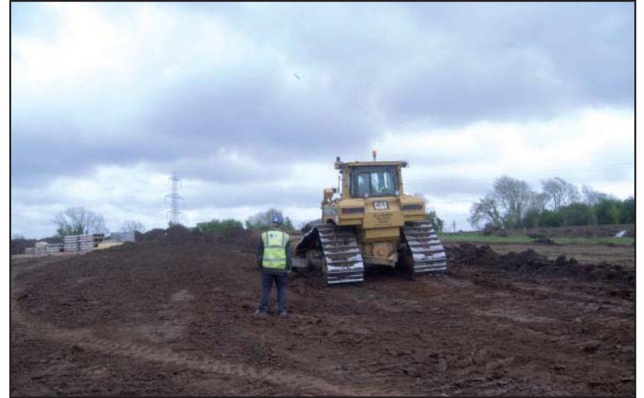
Plate 2: Main Field, stripping by bulldozer being supervised, looking east
