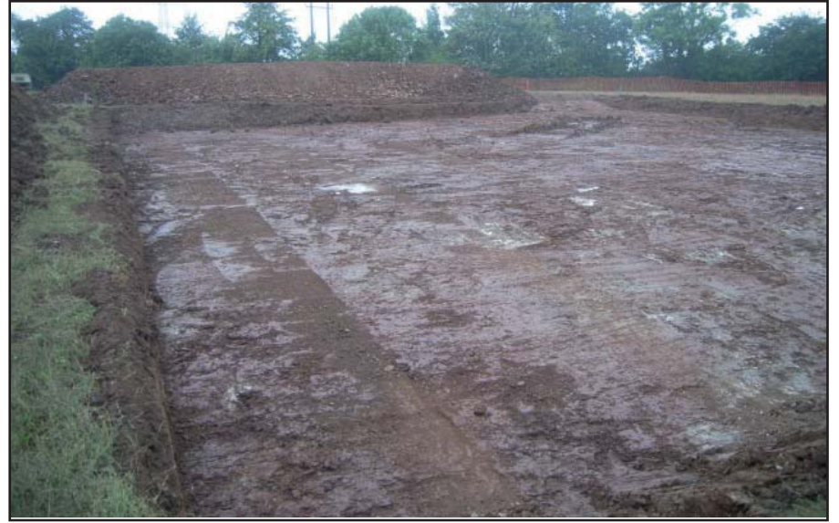
Plate 34: Trench 45 Excavation Area, looking north-west
