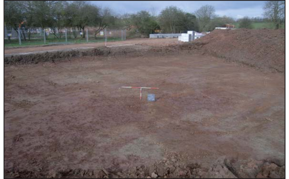
Plate 30: Trench 27 Excavation Area, looking south-west
