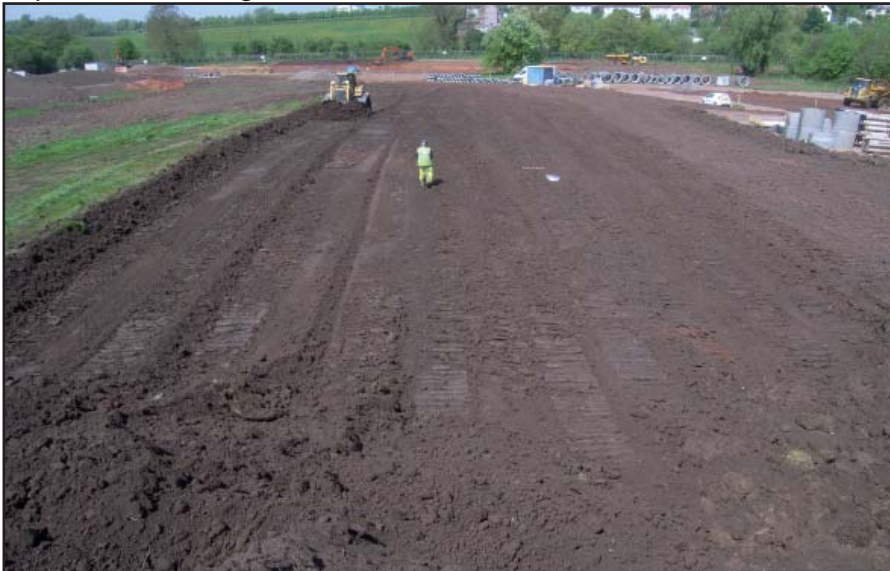
Plate 3: Main Field, stripping by bulldozer being supervised, looking west
