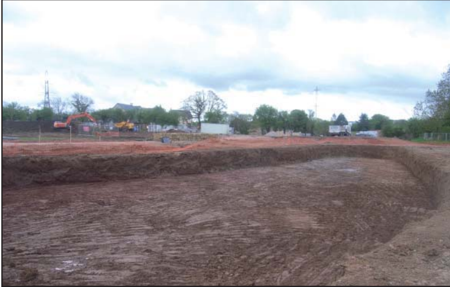
Plate 5: West Field, completion of the Balancing Pond, looking south
