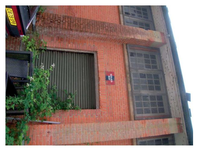
Plate 9: Inserted loading door in north elevation
