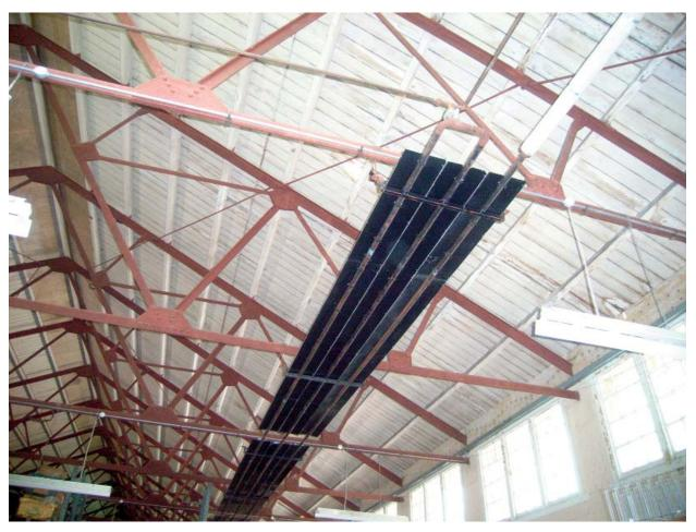
Plate 24: Heating racks on roof
