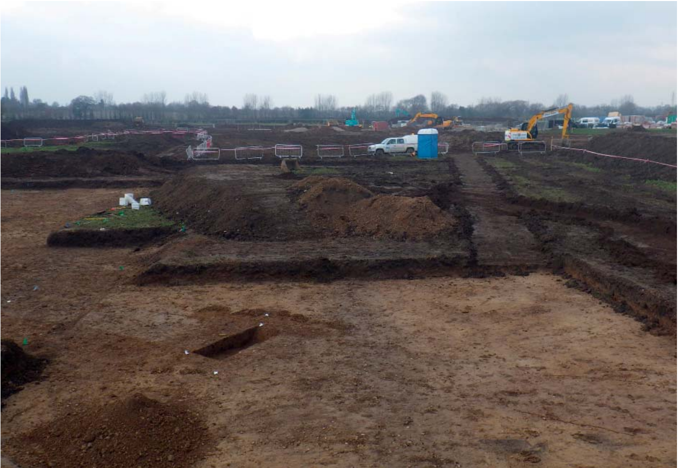
Plate 11: Area 15, northern excavation, site view
