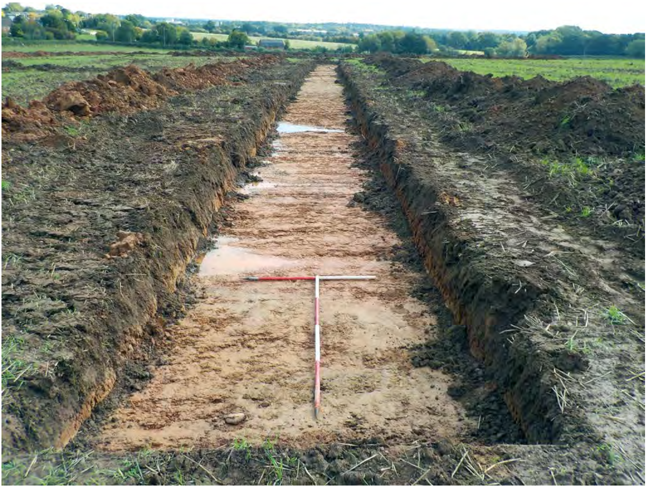
Plate 5: Trench 5 - View to ESE
