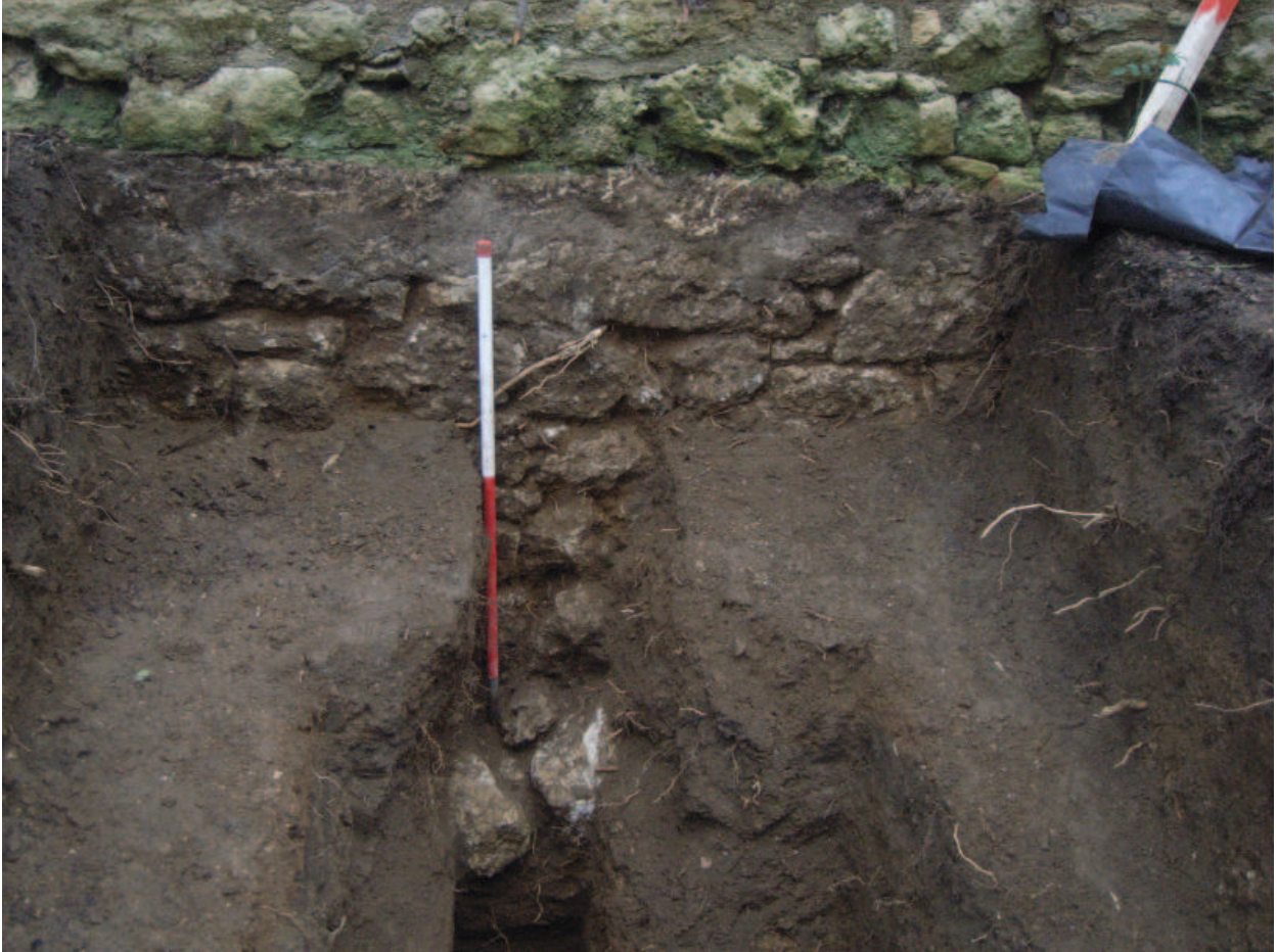
Plate 5: Sprotts Wall foundation looking E in Trench 3
