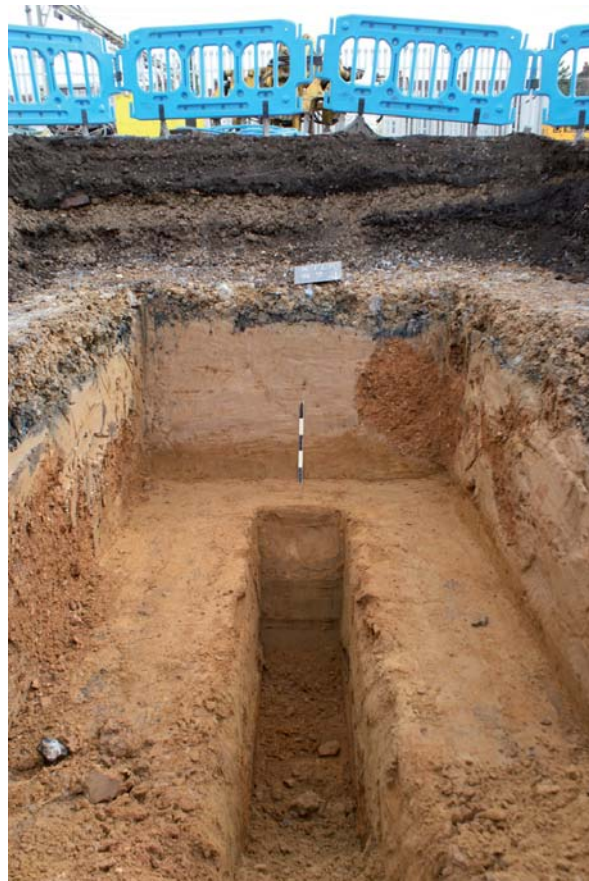
Plate 2: North-facing section of ATT9 showing the Ilford Silts (32) with sand filled ice wedge beneath modern "made ground" and above sands (36)
