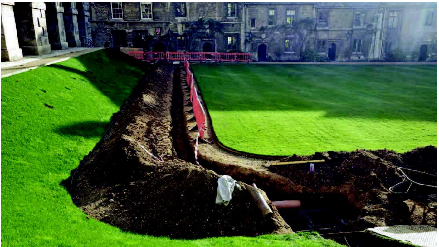
Plate 8: Shot of works through Main Quad, looking south
