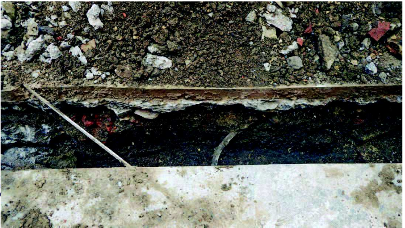
Plate 3: Layers beneath concrete path, Pump Quad, looking south
